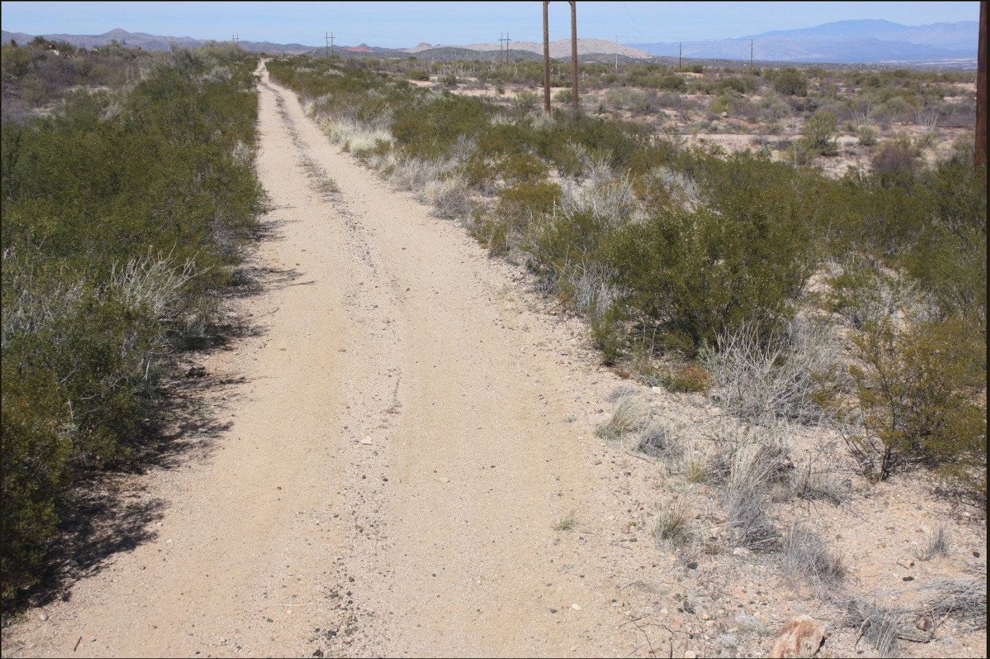
Northwestward view of the SMA (1955) switchback line to the San Manuel copper mine, a half mile west of the previous location where the grade emerges from the regraded smelter site. It's hard to tell in this view but this present dirt road is on a substantial fill grade.
