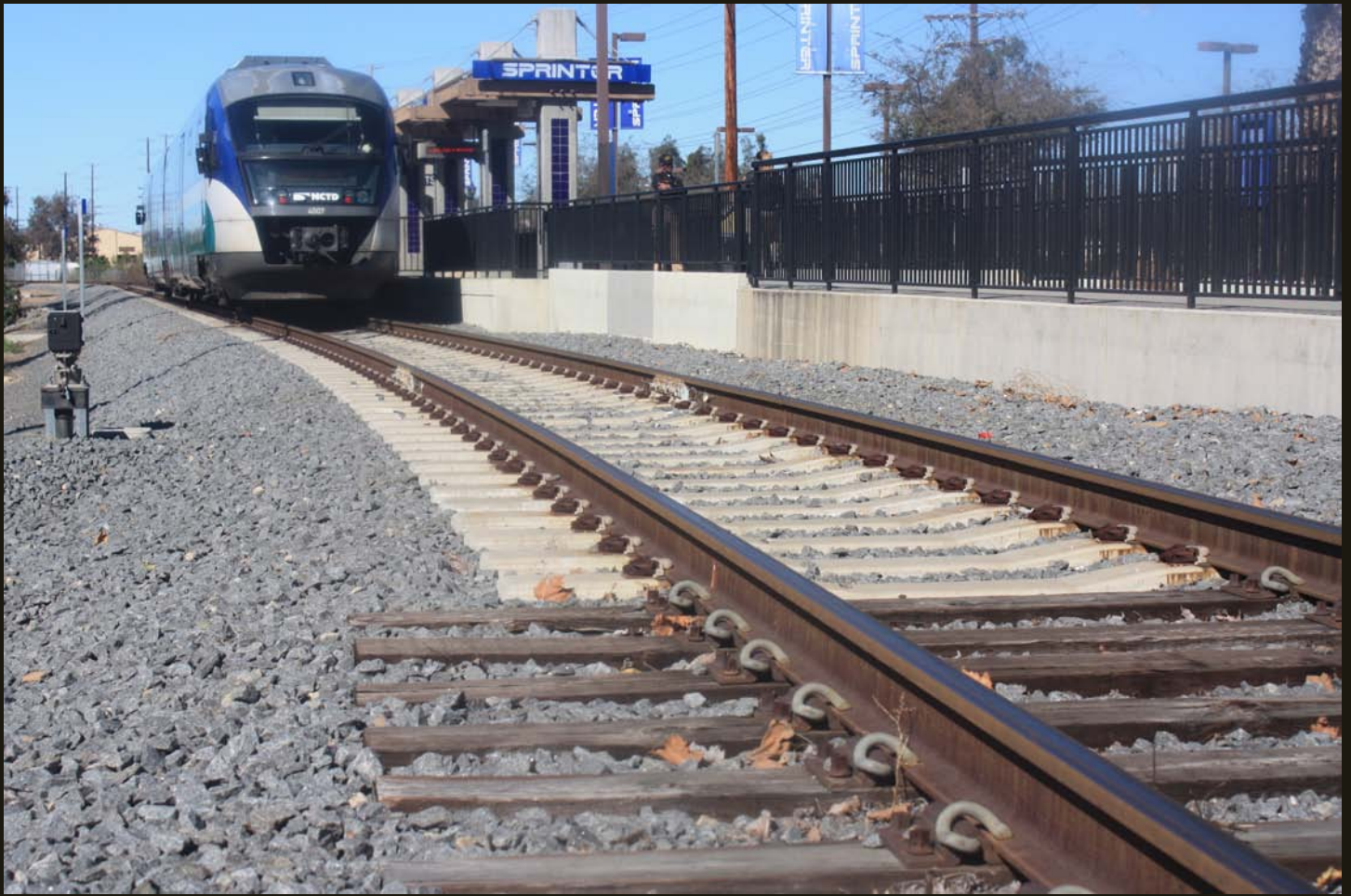
Closer view of the SPRINTER loading passengers at the Escondido Transit Center, the last stop on the line. Note the upgraded concrete ties on the SPRINTER route and the old wooden ties that continue to the old end-of-track.
