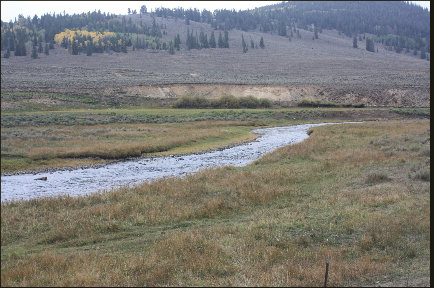
Southeastward view of the D&RG (1883n) and Tomichi Creek at the same location as previous. The fill grade alignment is straightening out, and at the far right edge of the photo the fill is starting to get eroded by Tomichi Creek (the cut grade at the base of the distant hill is a road).
