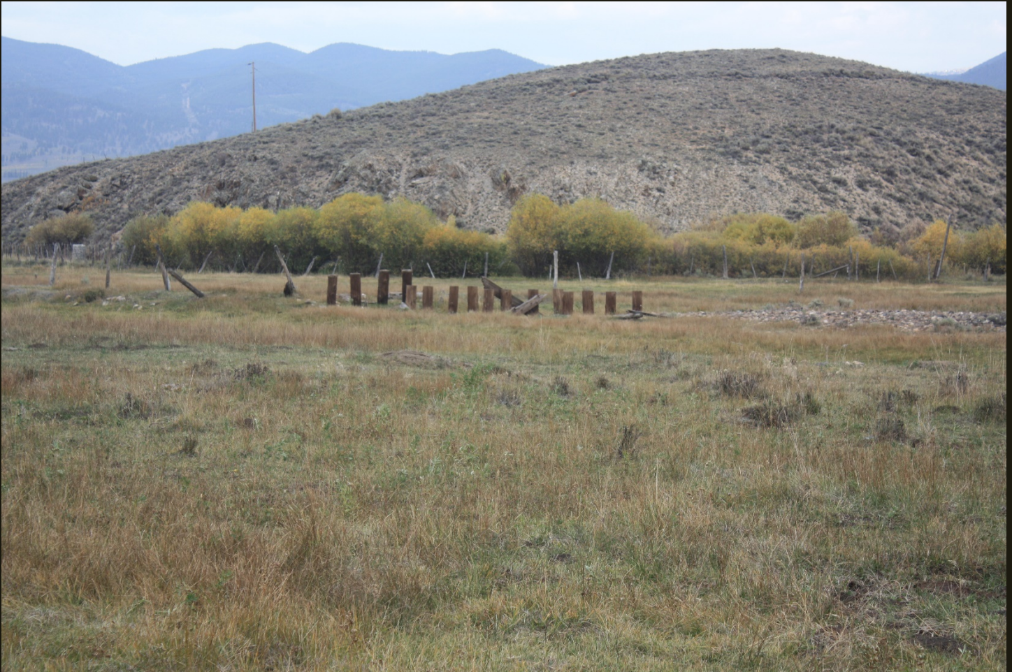
Eastward view of the D&RG (1883n) 1,500 feet south of the previous location. The pilings do not cross Tomichi Creek, which runs just in front of the pilings and is marked by gravel but the water cannot be seen in this view. The pilings may have been a bridge to carry the railroad over a former course of the creek or it may have supported a trackside facility.
