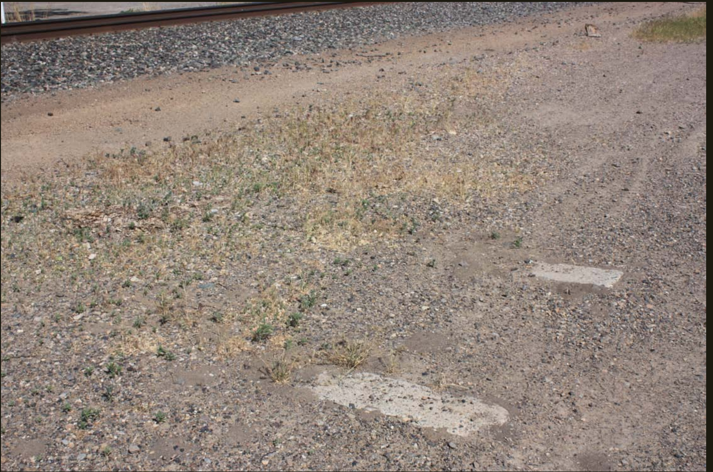
Traces of old foundations at the northern terminus of the NC (1880s) at Battle Mountain. The CP (1869), now UP, is at the top left.
