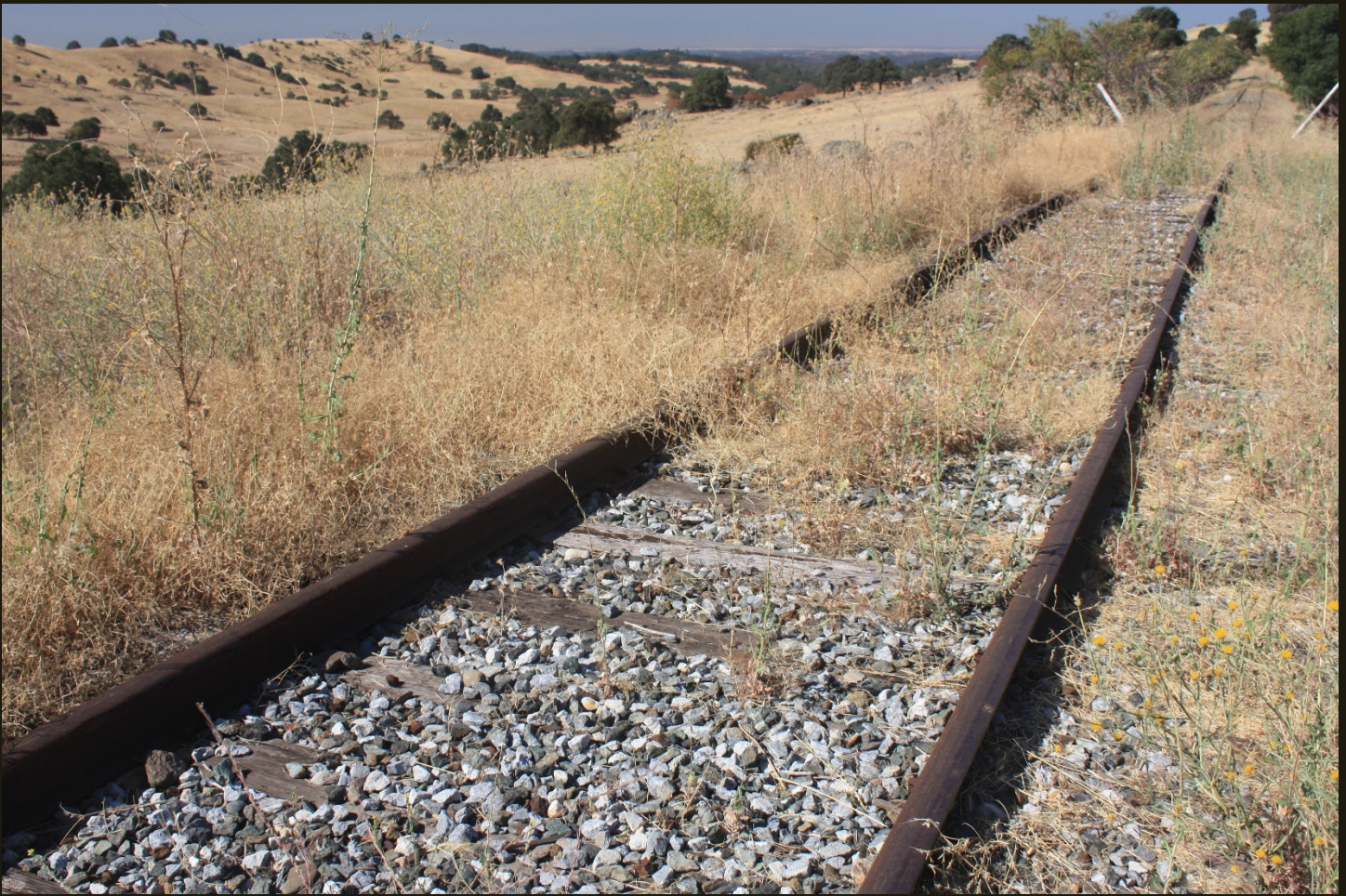
Westward view of the AC (1904), 2 miles east of previous location.
