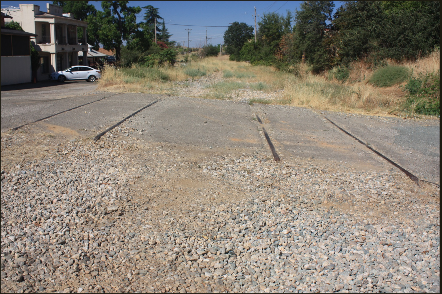
Southwestward view of the AC (1904) end of the line at Martell, 1.5 miles east of previous location where the track currently ends. The tracks are removed except for those in the road crossing. The road where the car is parked on the left is Depot Road.
