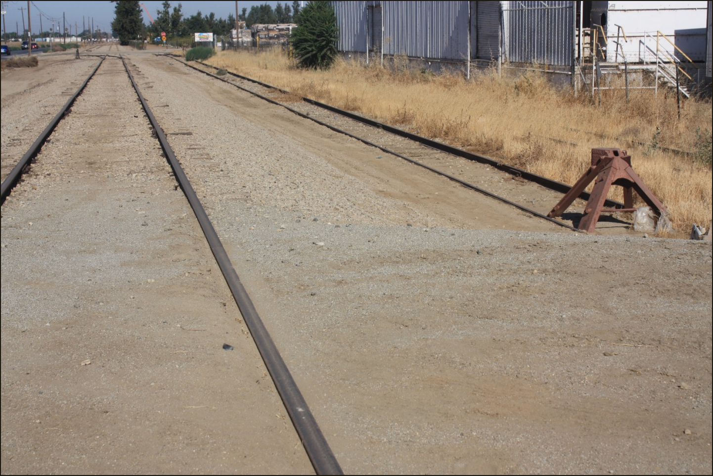
Westward view of the SP Arvin Branch (1923), 1.3 miles east of the curve at the previous location. The mainline is in the foreground, an agricultural siding ends in the right (north) foreground, and another siding splits off to the left of the mainline in the middle distance.
