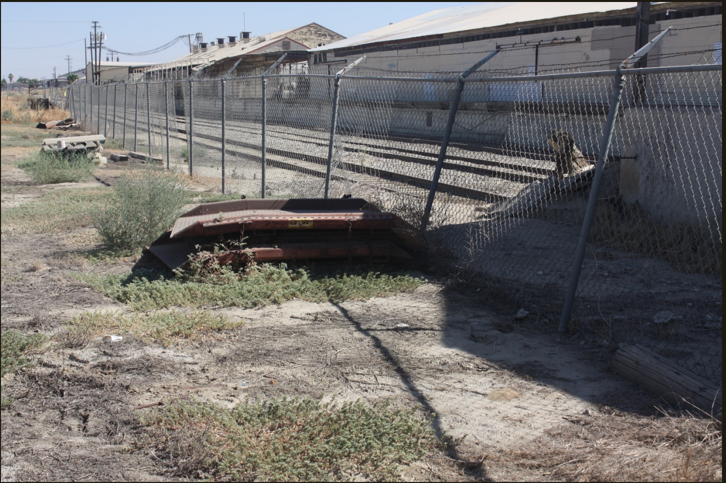
Northward view of the SP Arvin Branch (1923), a quarter mile south of the previous location and 0.5 miles south of the split in the track. The end of track is within the fenced area in the shadow at the right. The agricultural warehouses and loading facilities on the right are now a reclamation facility. The Gold Ribbon Potato Company warehouses and loading facilities of the Gold Ribbon Potato Company are just out of view on the left and appear to be out of business.
