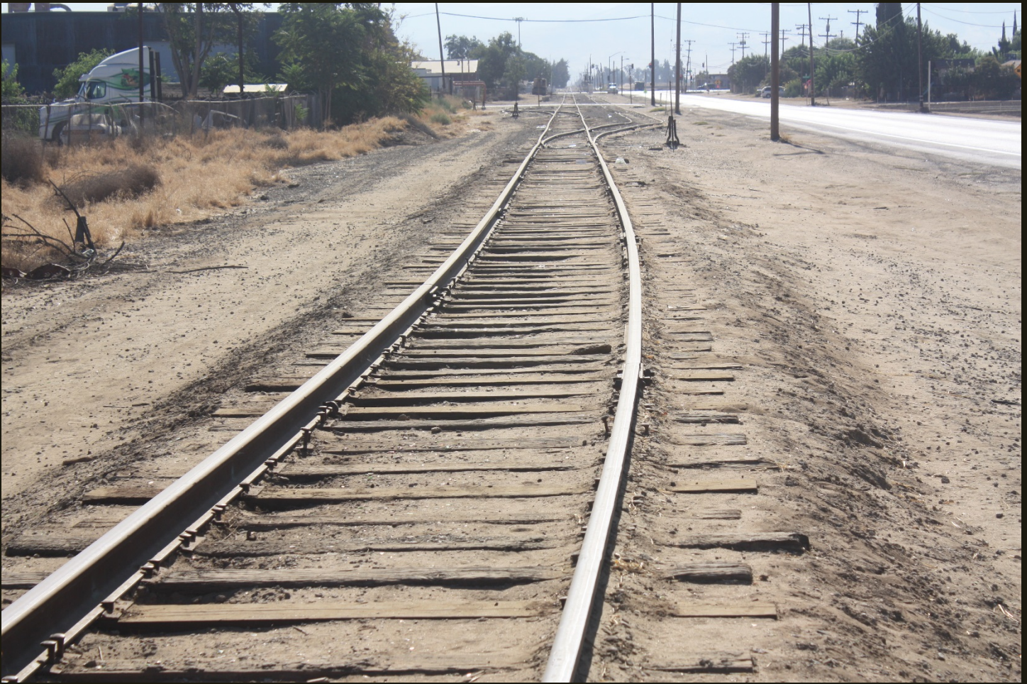
Eastward view of the SP Arvin Branch (1923), same location as previous, where the 90-degree curve ends and the line straightens out to a due east alignment.
