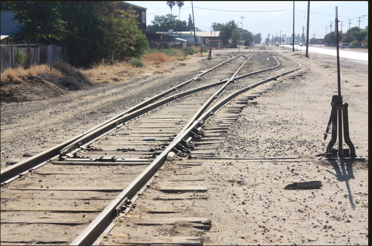
Closer eastward view of the sidings in the previous photo.
