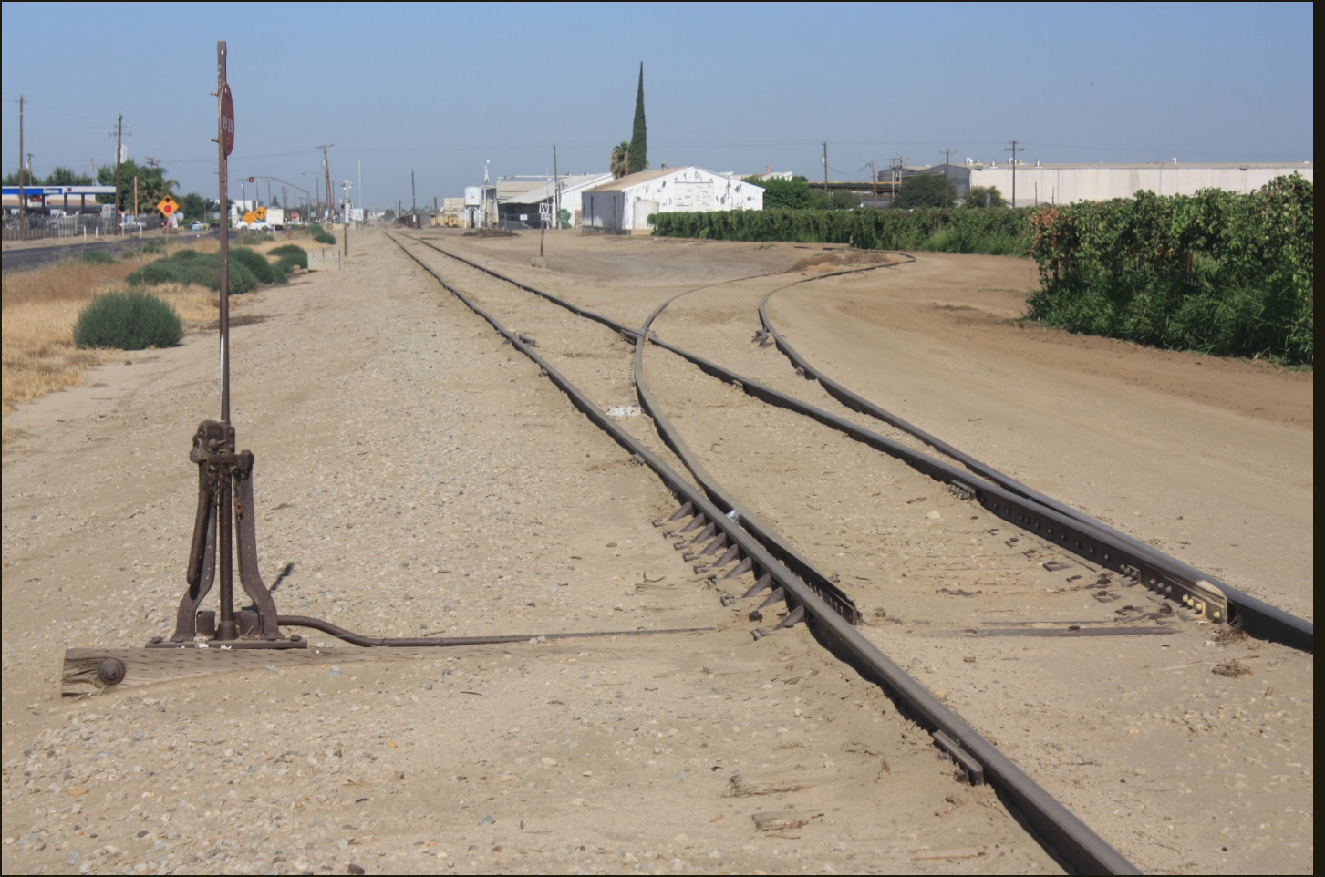
Westward view of the SP Arvin Branch (1923), 3.4 miles east of the previous location. The orchard to the right (north) makes way for yet another agricultural siding.
