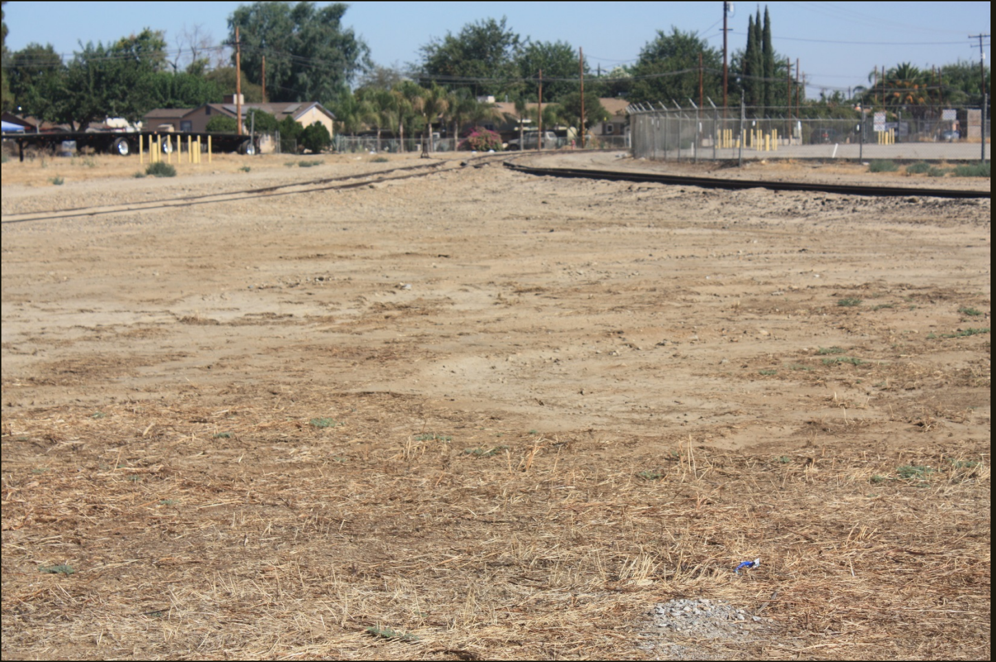
Northward view of the SP Arvin Branch (1923), 3.5 miles south of previous location, on the south side of Arvin. There's a switch and the track splits; the track on the left continues due south for 0.5 mile and the track on the right turns due east for 0.5 mile then due south for 0.5 mile, all three alignments still following the property-boundary grid. First, we'll look down the left branch.
