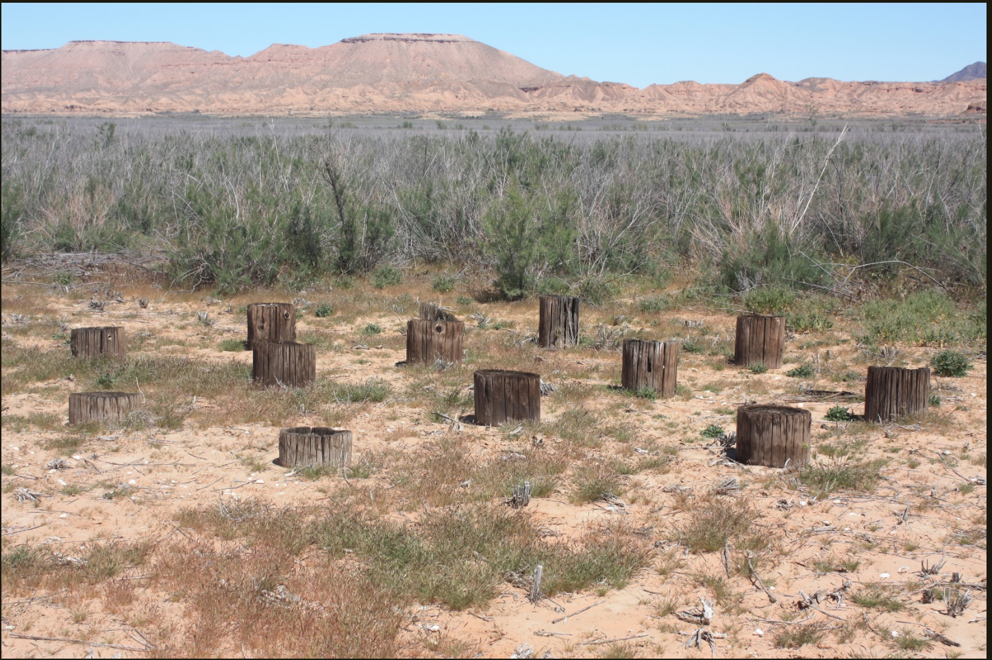
Northeastward view of some wooden piles, 300 feet northwest of the foundation, the only other structure of any sort along the SPLA&SL St. Thomas Branch (1912) at St. Thomas.
