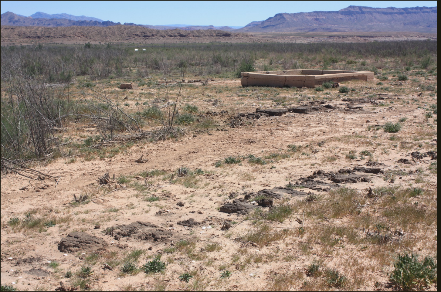
Eastward view of the same foundation and oil-soaked dirt. The darker dirt in the foreground has particularly convincing tie impressions.
