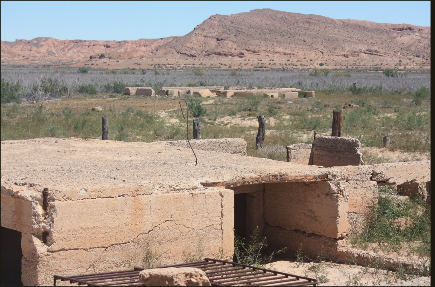
Old foundations in St. Thomas. Note the contrast in vegetation on the relatively verdant floodplain of Muddy River and the drier mountain slopes.
