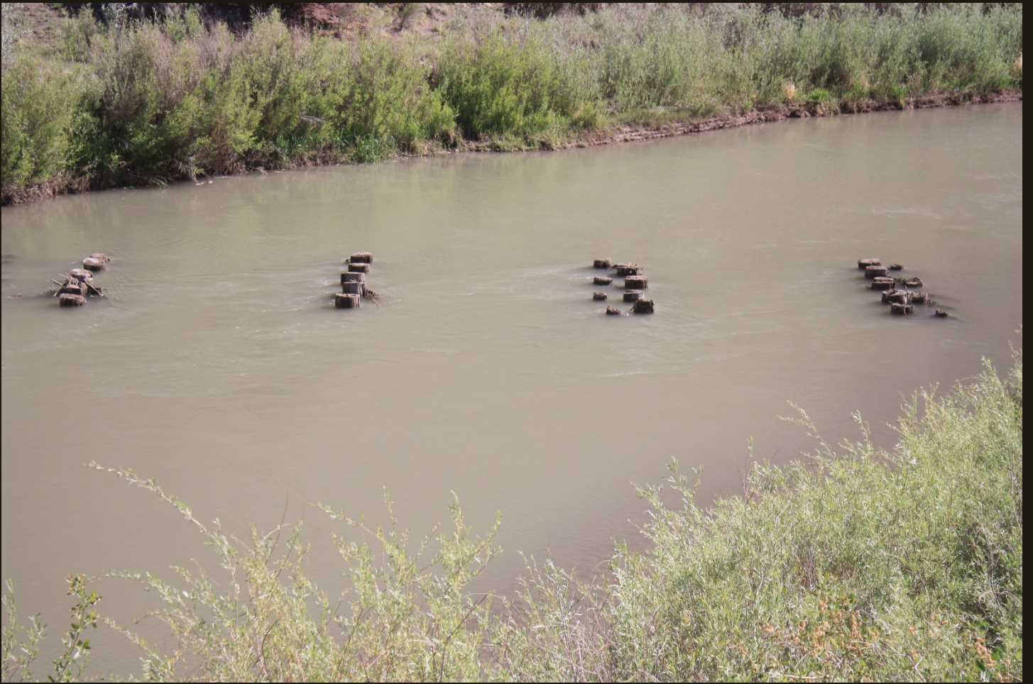
Closer view of the cut piles.
