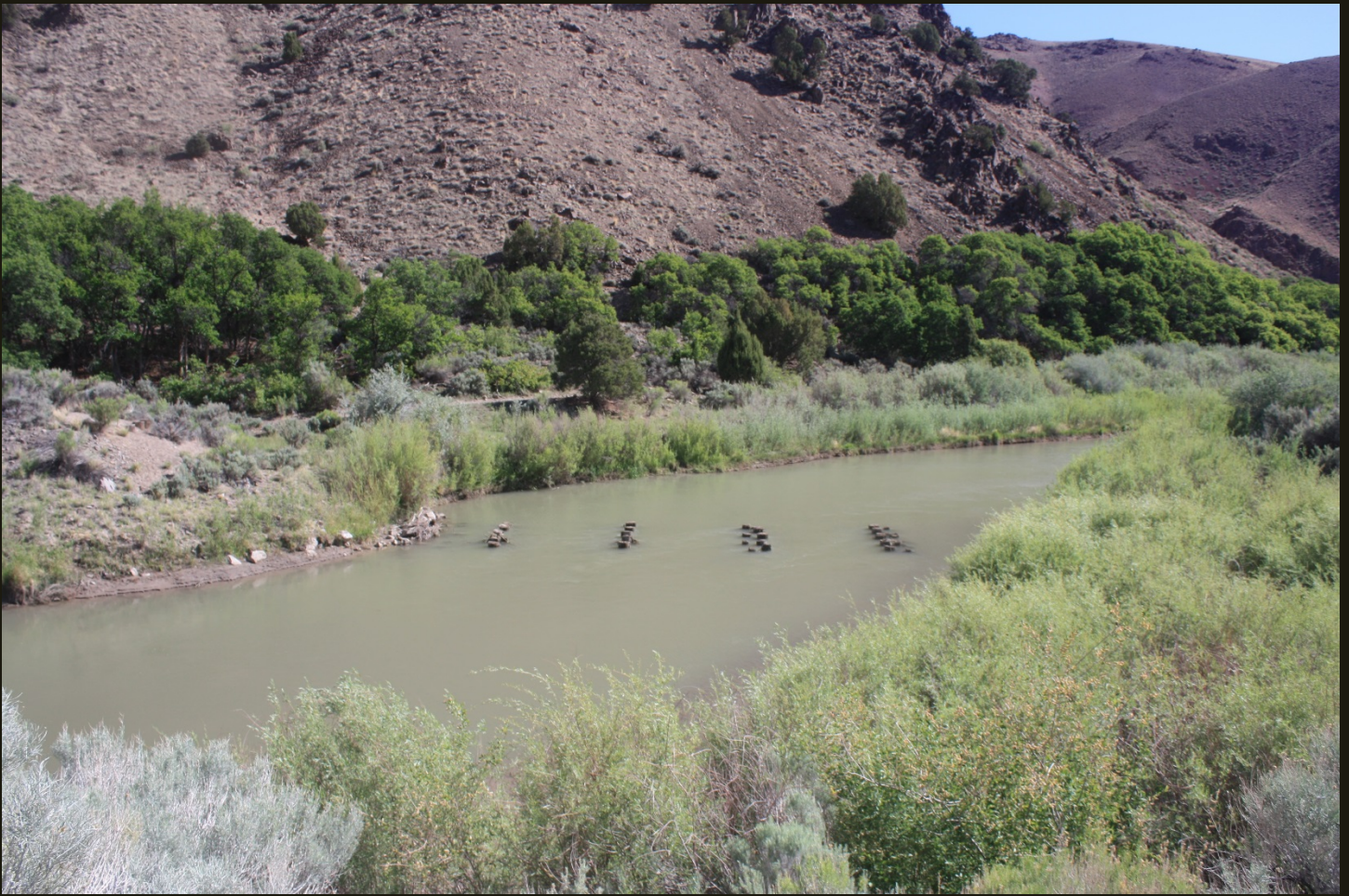
Eastward view of the SV (1900) 2 miles south of Caboose Village and 3 miles north of the end-of-the-line at Marysvale. Wooden piles that once carried the SV (1900) over the Sevier River were cut at the water line during abandonment.
