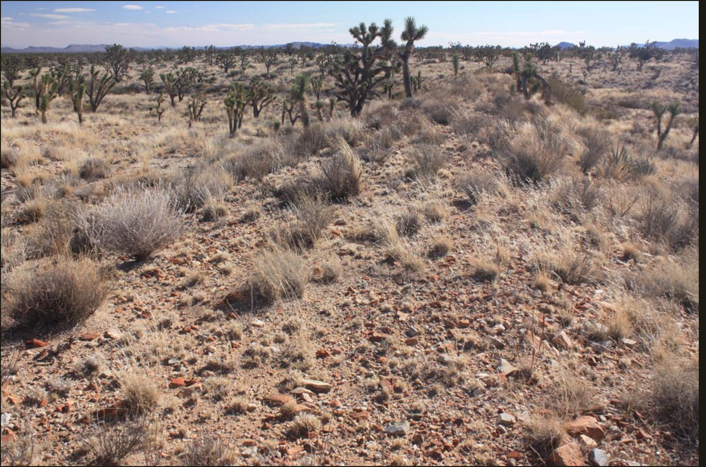
NS fill grade 1 mile north of Lanfair. The gravel appears to be original ballast.
