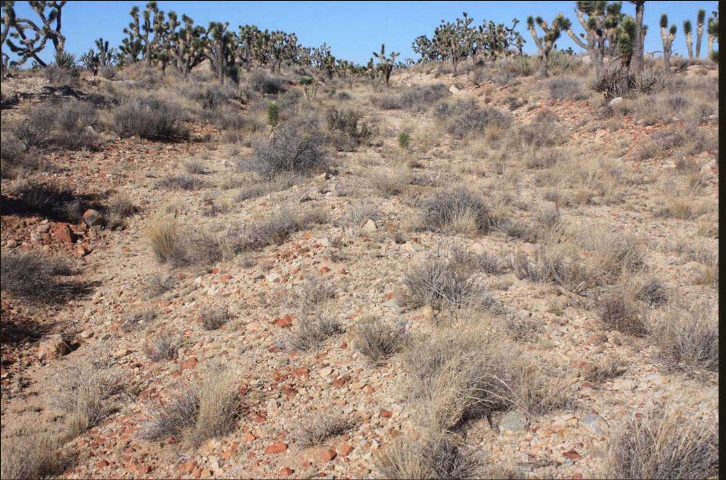
NS cut grade 1 mile north of Lanfair.
