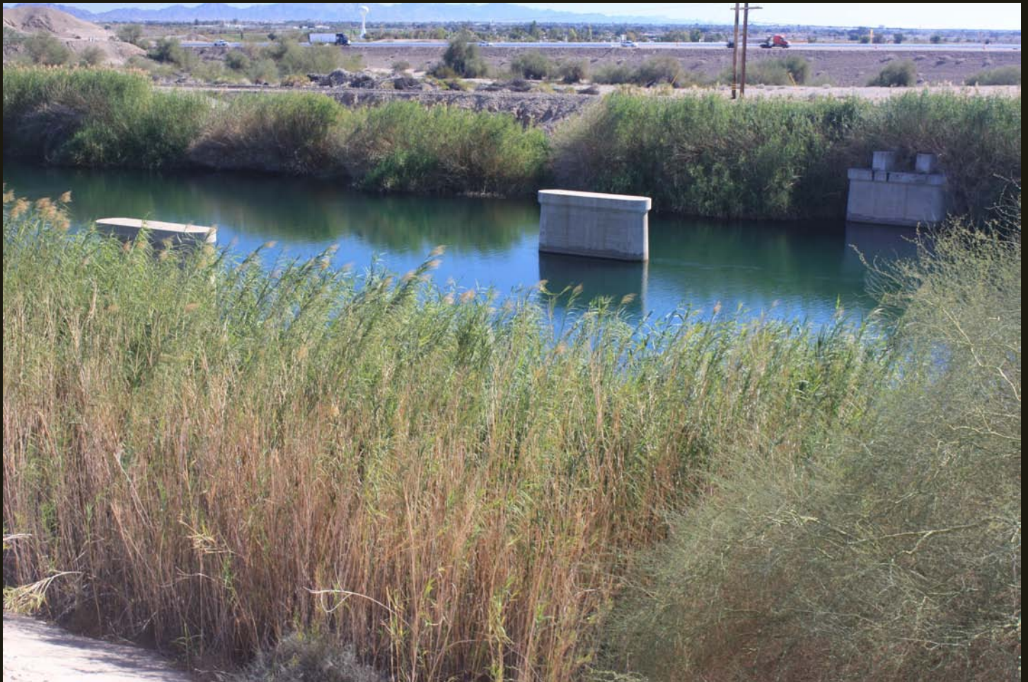
Southward view 500 feet south of Araz Junction, showing supports for a bridge that once carried the SP Inter-Cal (1904) over the All American Canal. The canal is a primary conduit of diverted Colorado River water for irrigation. The Araz Junction wye splits into its two branches about 100 feet north of the canal.
