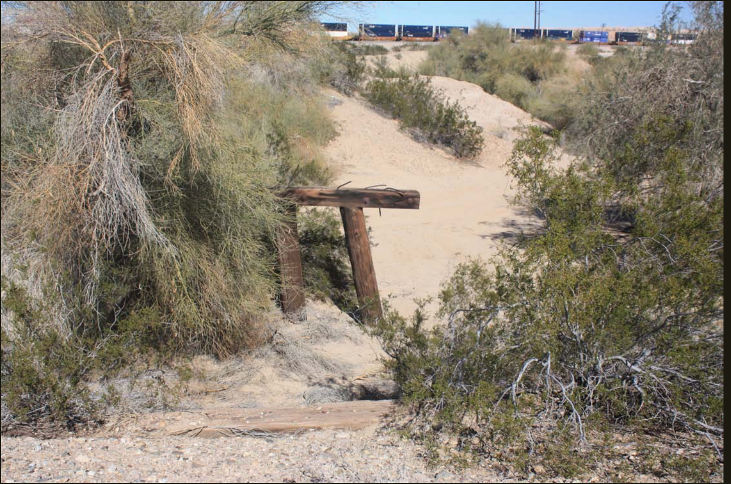
Northward view of a trestle that once carried the SP Inter-Cal (1904) to Araz Junction. The container train is on the SP Sunset Route (1881).
