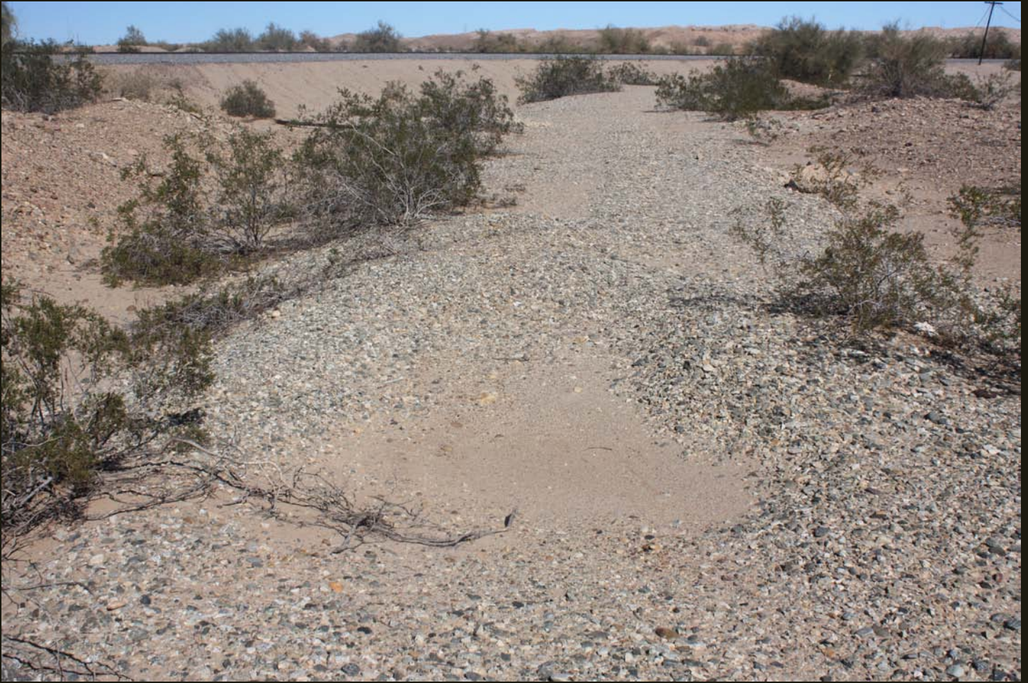
Northward view of the fill grade (foreground) for the east branch of the Araz Junction wye for the SP Inter-Cal (1904). The tracks of the SP Sunset Route (1881) are visible in the distance.
