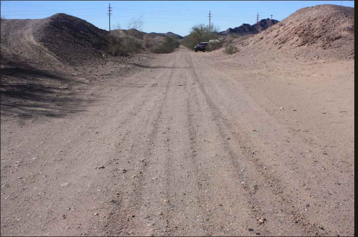
Southwestward view of the SP Inter-Cal (1904) grade, same location as the previous photo.
