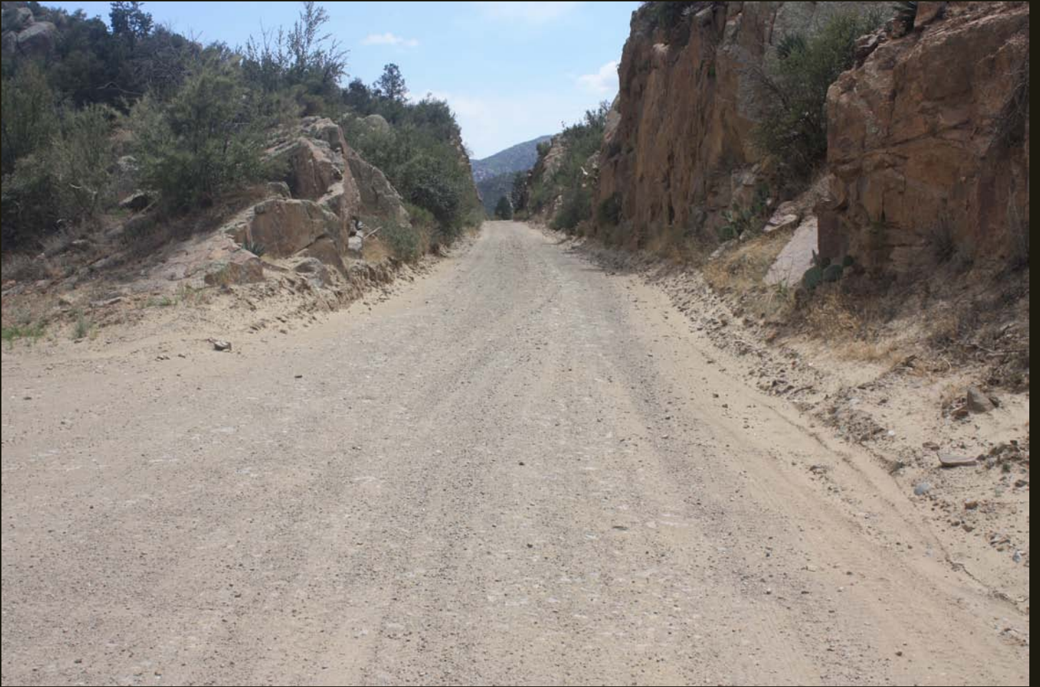
Crown King Road uses the BM grade to climb up to Crown King from Cleator.
