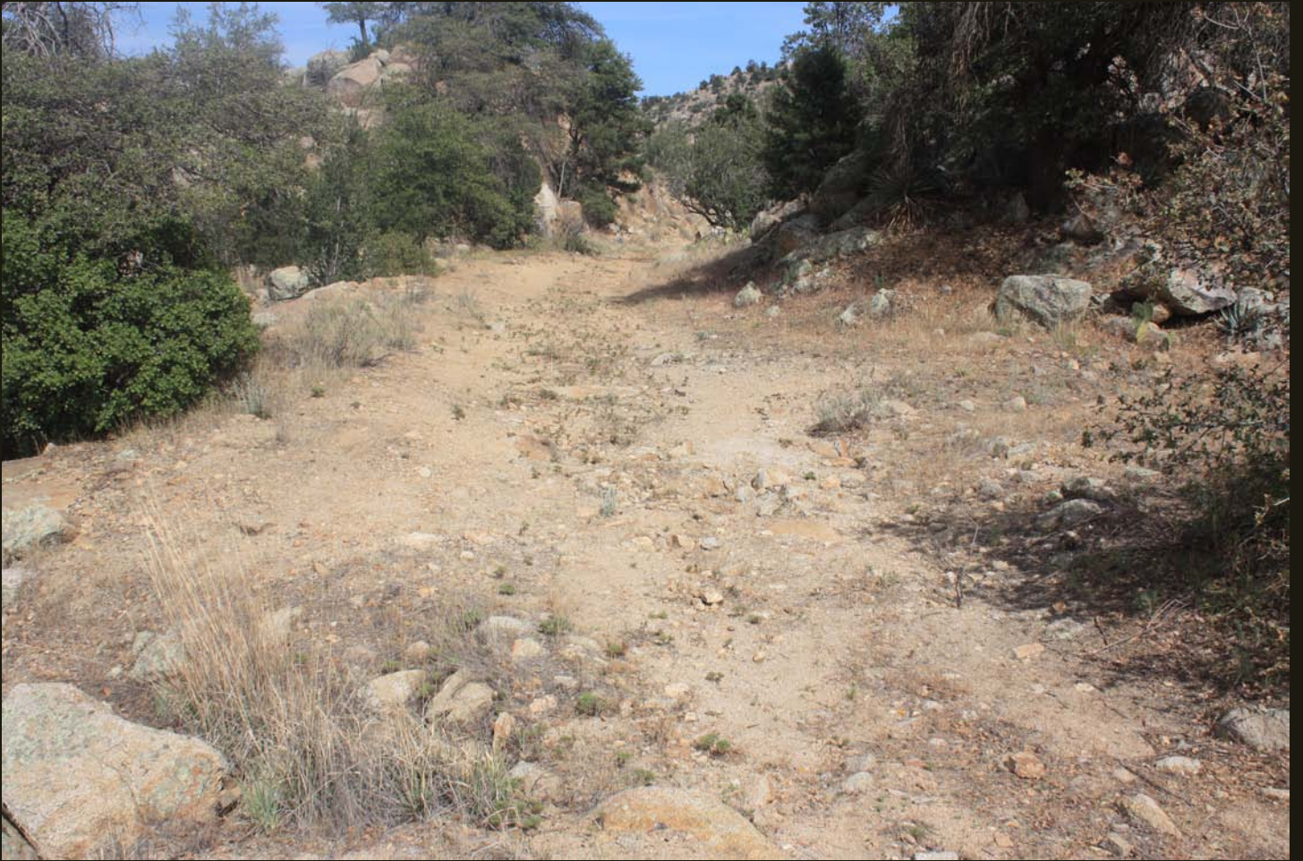
Cut grade for a switch and single track switchback.
