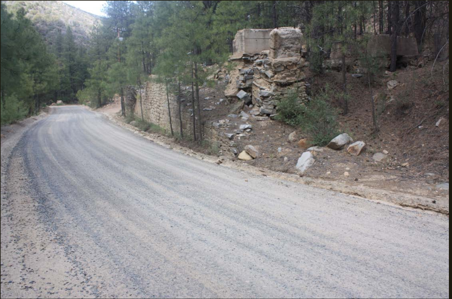
Crown King. The road is still on the BM grade, here close to the former end-of-track, and the structure is an old loading facility.
