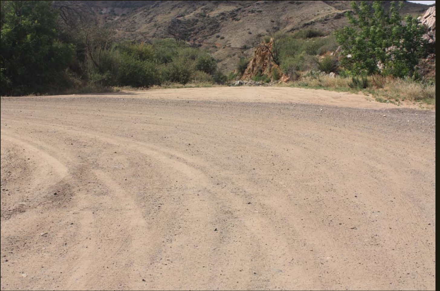
Closer view of a switchback. The re-graded U-turn is in the foreground and the cut beyond is for a switch and single track.
