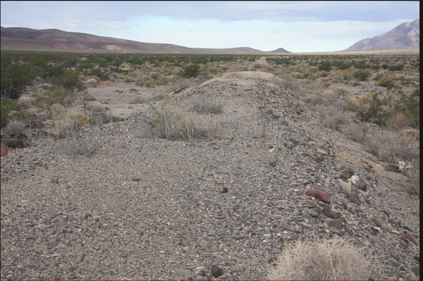
Northwestward view of the grade of the DV (1914n) at the same location as previous. Note the breach in this fill grade in the middle distance and the curve to the right beyond the breach.
