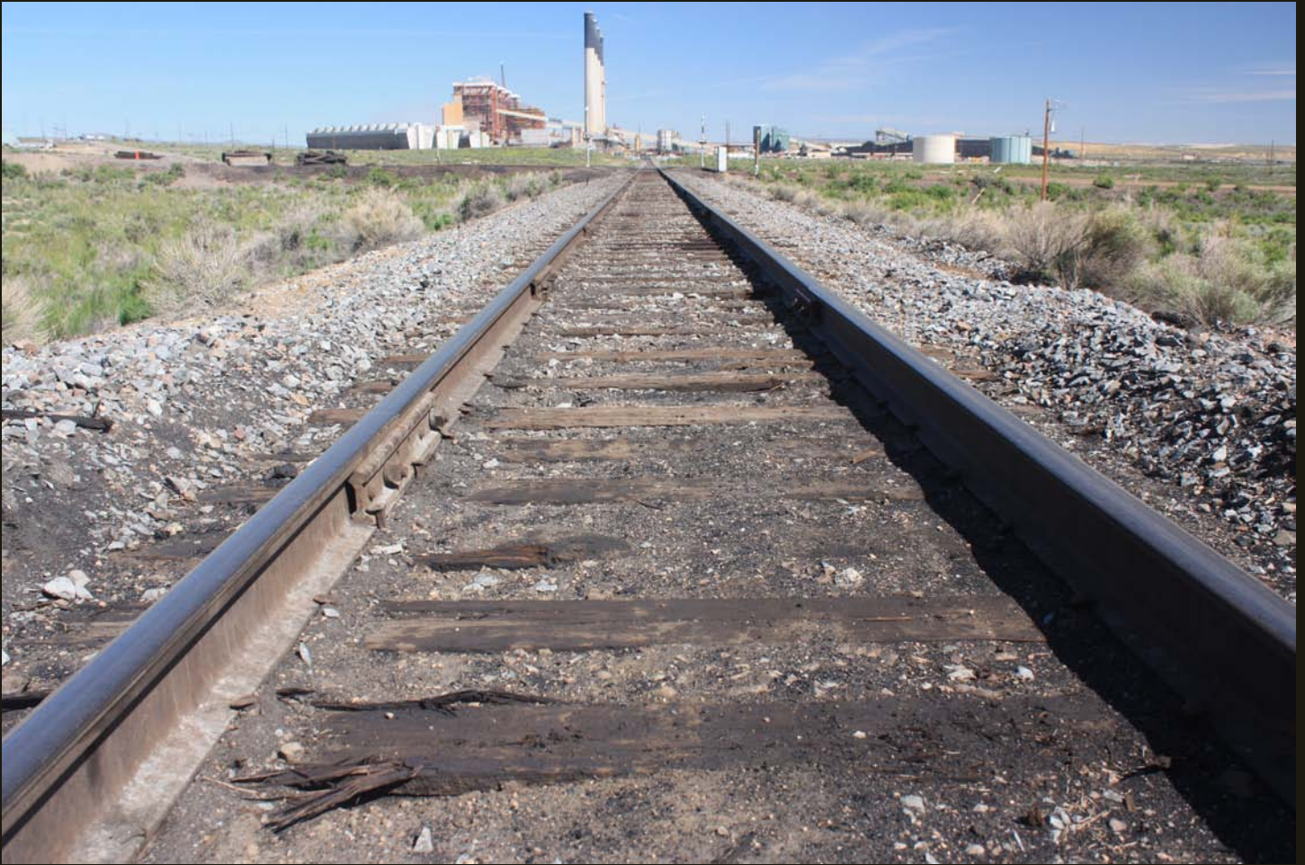
The coal-burning Jim Bridger Power Plant was built in 1974 on the Bridger coal spur. The coal is transported on a four-mile-long conveyor belt from the Bridger Mine to the plant and on this railroad from the Black Butte Mine.
