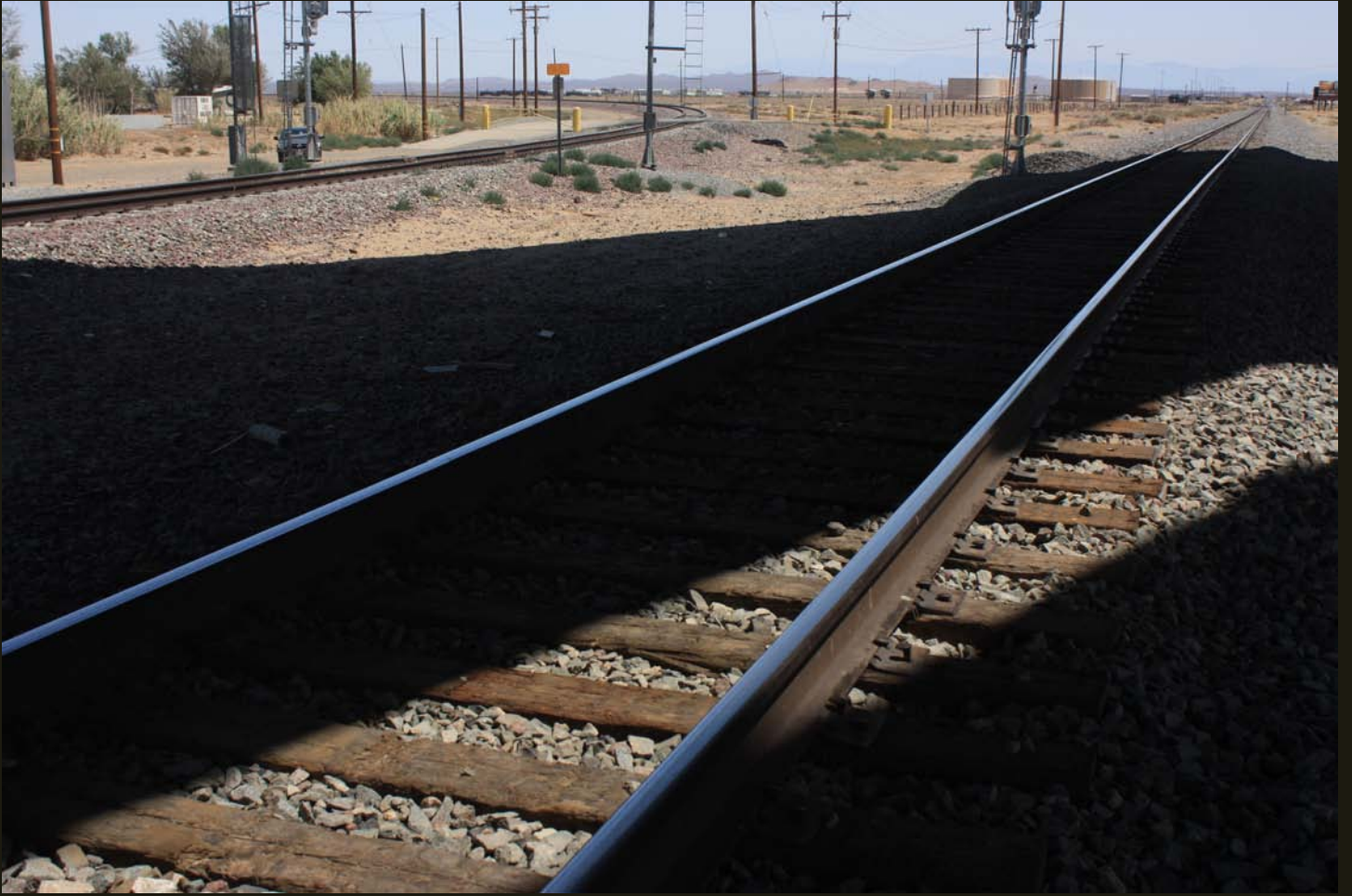
Another southward view of the SP mainline (1876) in the foreground beneath California Highway 14 and SP Needles Branch (1883) to the left.
