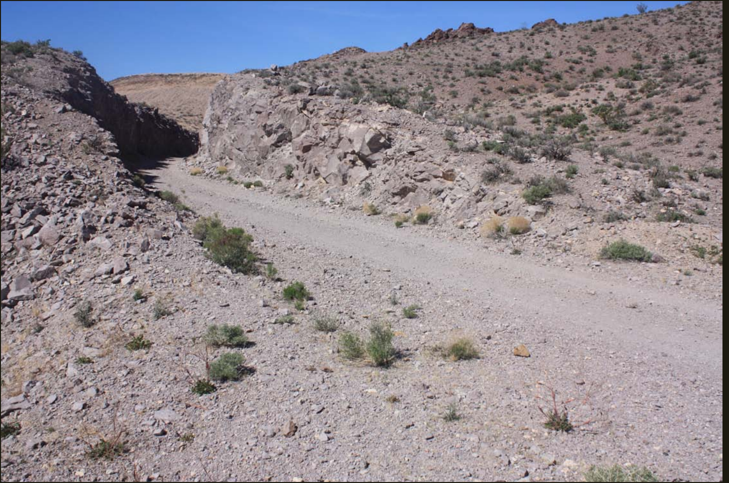
Closer view of the cut grade in the previous photo.
