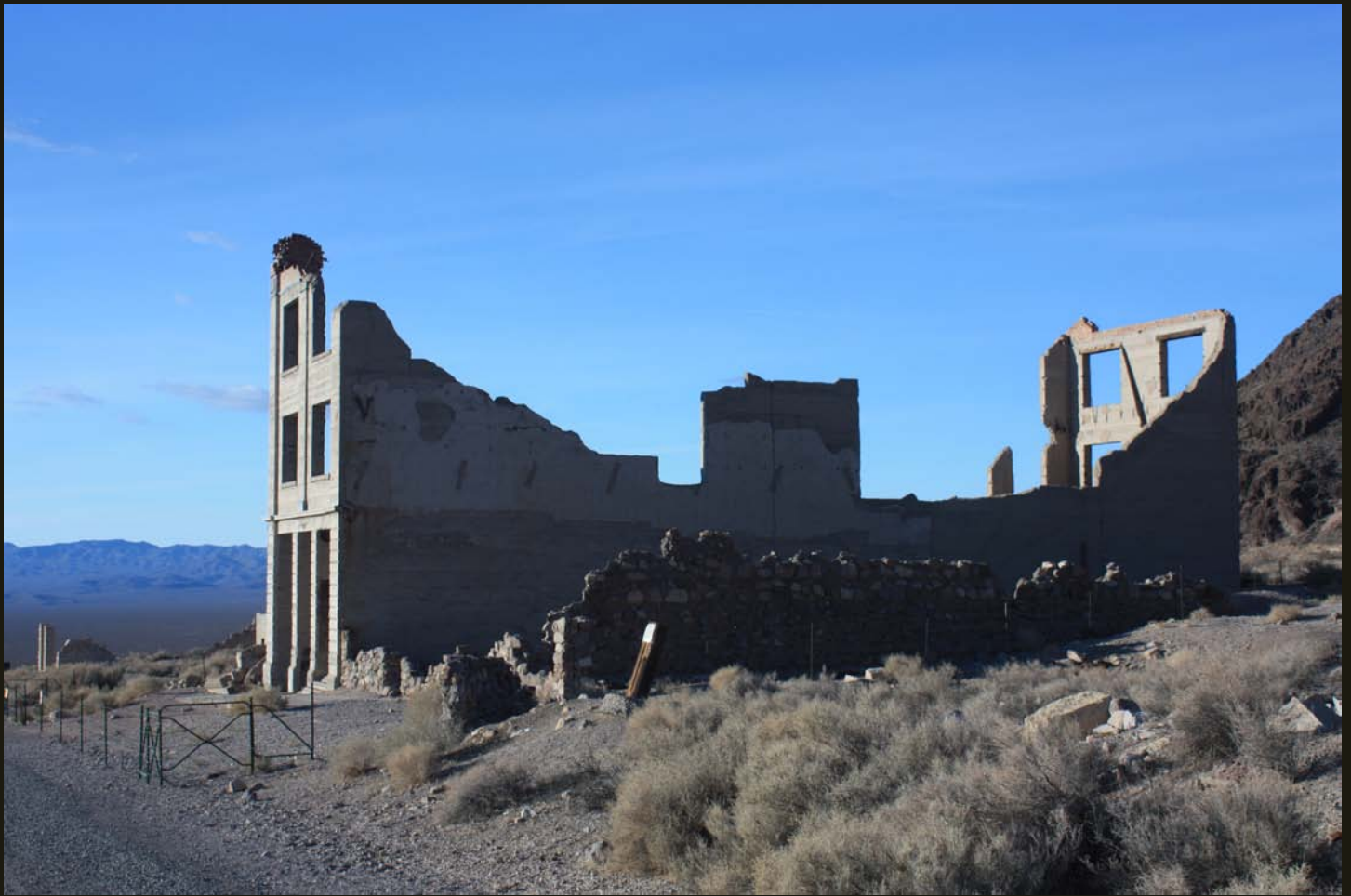
The three-story John S. Cook and Co. Bank on Rhyolite's Golden Street was built in 1908 and epitomized Rhyolite's opulence, featuring Italian marble stairs and imported stained-glass windows, all brought in by rail.
