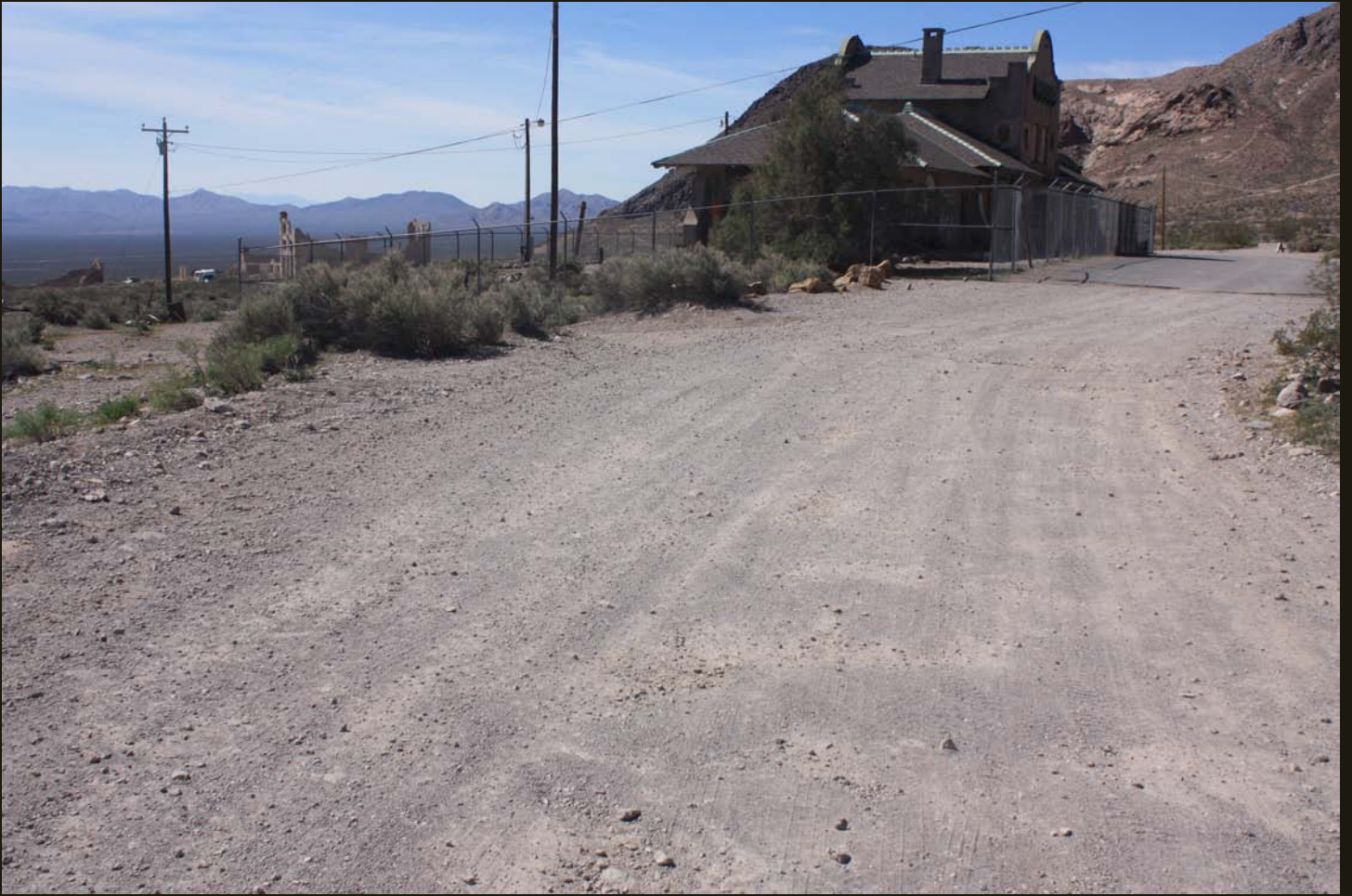
Westward view of the LV&T (1907) grade (foreground) and the LV&T Rhyolite Depot.
