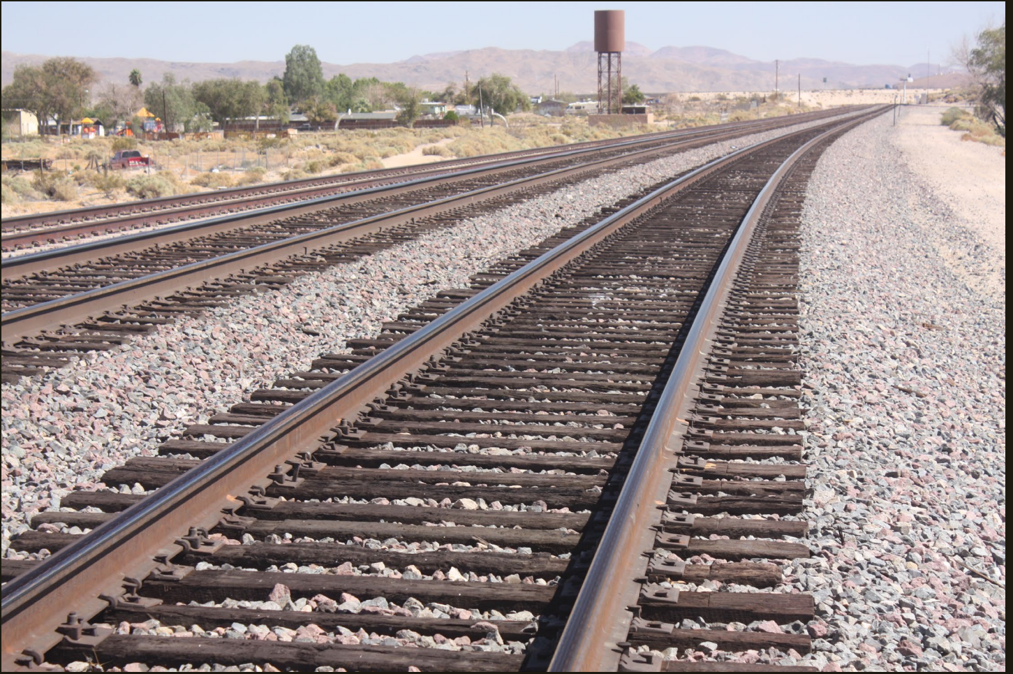
Northeastward view of the CS (1885) alignment, one mile west of previous location.
