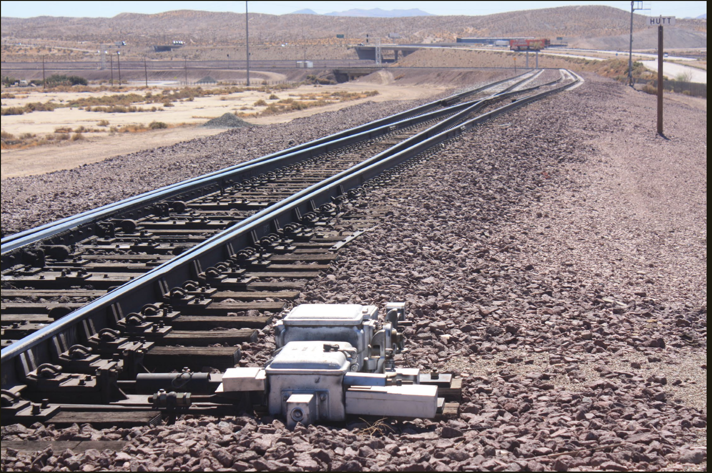
Southward view of the 1976 re-alignment, same location as previous. A switch splits the single wooden-tie track into a double concrete-tie track, which curves to the left (east) as it approaches the "new" (presumably 1976) junction with the CS (1885) alignment.
