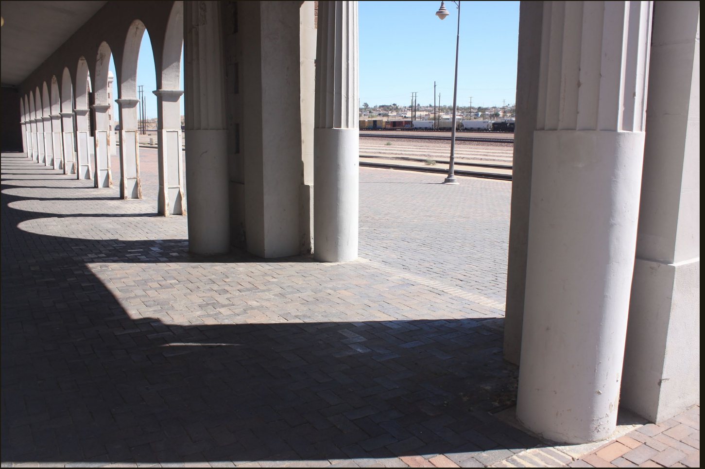
Southeastward view of the passenger loading tracks and the "old" yard from Casa del Desierto.
