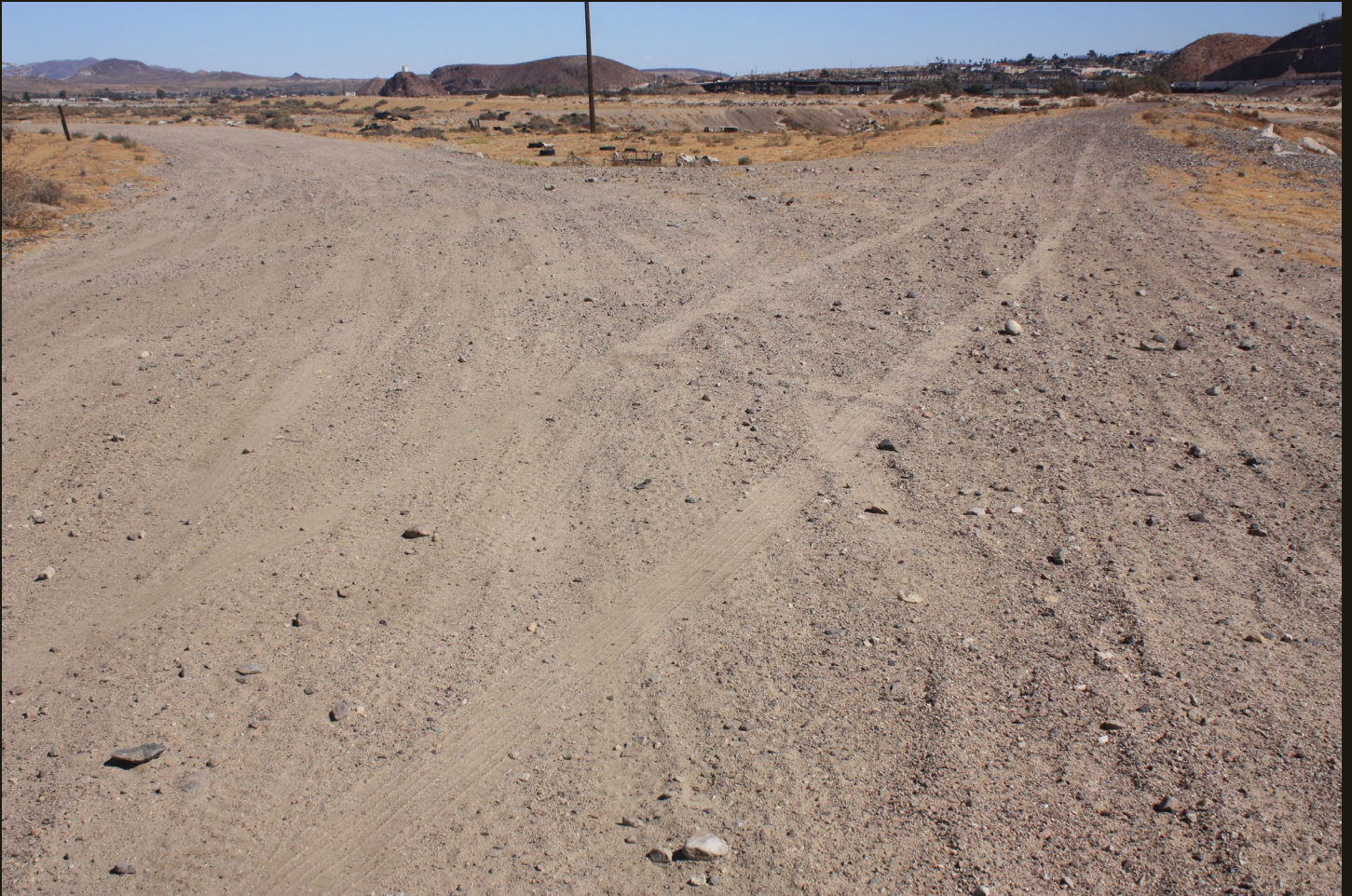
East-southeastward view, 500 west-northwest of the previous location. The grade on the right is the SP Needles Branch (1883), which was operated by the AT&SF since the time it was built, and the curved grade of the left is the northwest branch of an abandoned turning wye.
