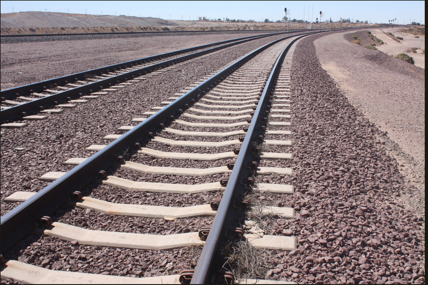
Southwestward view of the west branch of the new wye, a few steps northwest of the previous location. The CS (1885) alignment is visible to the left.
