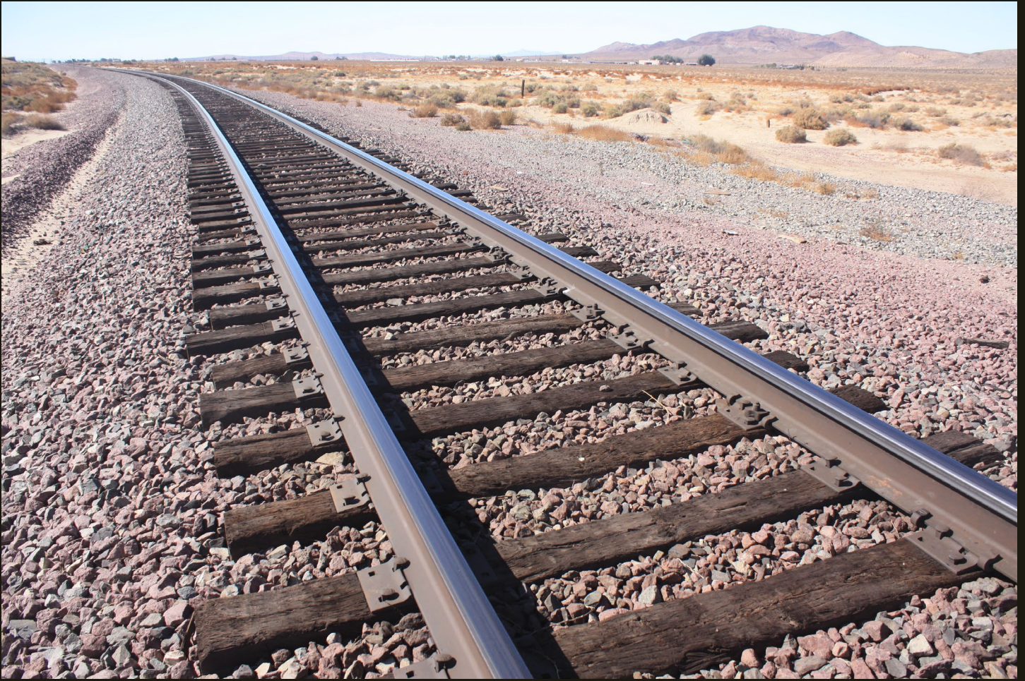
Northwestward view of the SP Needles Branch (1883), a few steps west of the previous location. The straight track in the left distance is on the original 1883 alignment, the gray (not pink) gravel in the right middle-ground is the abandoned continuation of the 1883 alignment, and the curved track is the 1976 re-alignment. This location is 4 rail miles west of Casa del Desierto and the former junction with the CS (1885).
