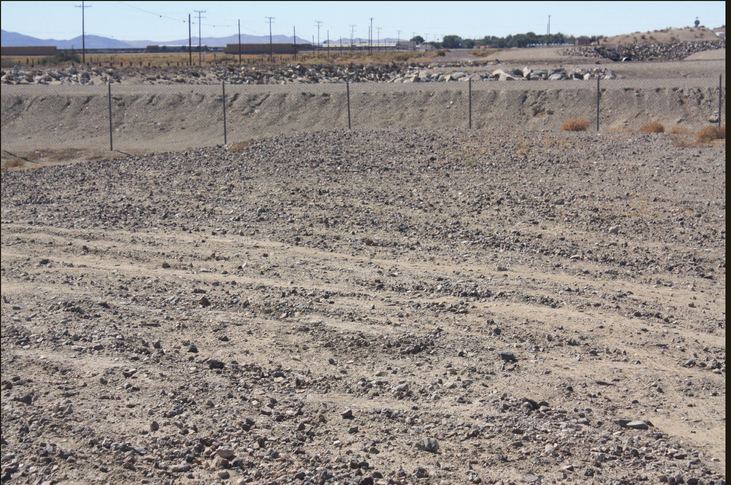
Westward view of the SP Needles Branch (1883), 1 mile west of the previous location. The grade ends at a wash, then picks up on the other side where it turns slightly to the right (a bit north of west). Whatever bridge or culvert that was once here is now gone without a trace.
