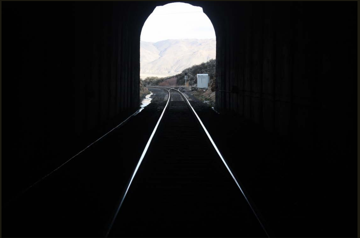
Eastward view from the Chilcoat Tunnel. Note the groundwater draining from the east end of the tunnel. The range in the background is Petersen Mountain, just across the state line in Nevada and the first of many normal-fault-bounded mountain ranges that extend across Nevada and into Utah.
