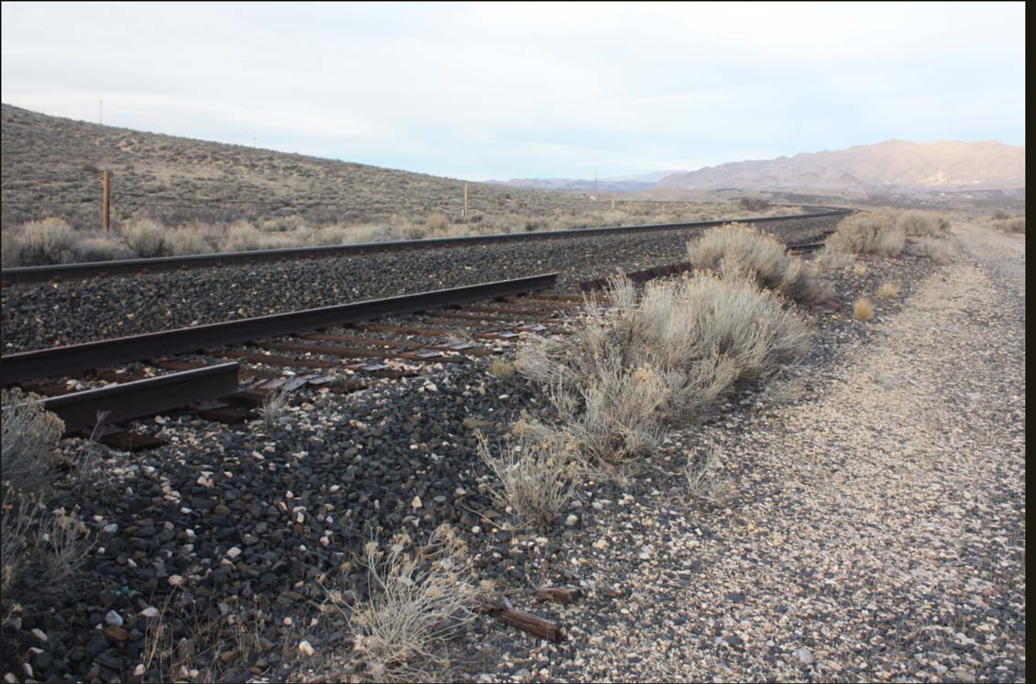
The end of the siding tracks, a few feet beyond the previous picture and the bundle of ties.
