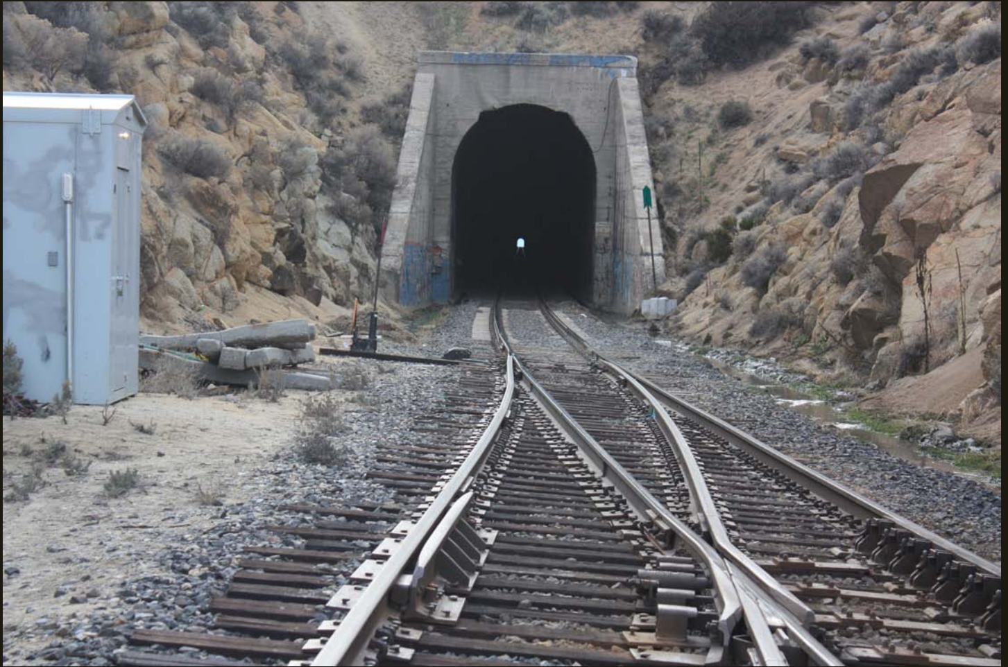
Closer view of the Reno Junction switch between the WP mainline and the siding for the Reno Branch. The original Chilcoot Tunnel was shored with timbers, which burned in 1912. A temporary “shoofly” track was constructed over the pass in 10 days and served as the mainline crossing until the current tunnel was completed in 1913.
