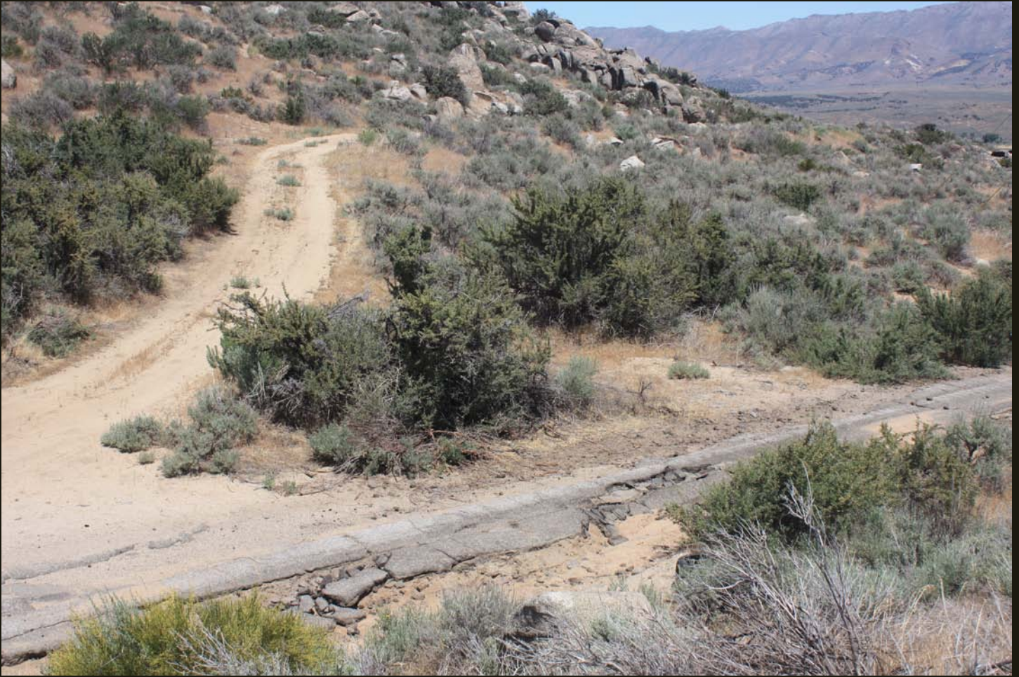
Northeastward view at the northern shoulder of Beckwourth Pass. The dirt road to the left is the WP shoofly alignment used 1912-1913 while the Chilcoot Tunnel was being repaired below the pass. The pavement is an earlier version of California Highway 70, which used the shoofly alignment at the pass but took a steeper grade to the east.
