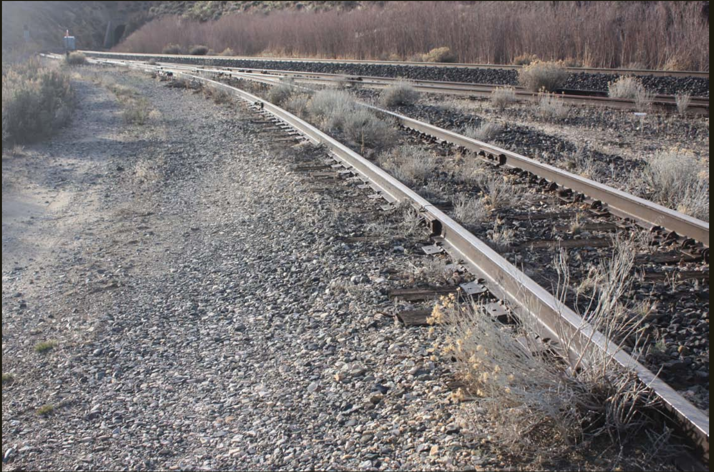
In this westward view at Reno Junction, the west branch of the wye for the WP Reno Branch is in the foreground, it connects to a siding, and the WP mainline is behind and higher than the siding. The Chilcoot Tunnel carries the WP mainline under Beckwourth Pass in the distance.
