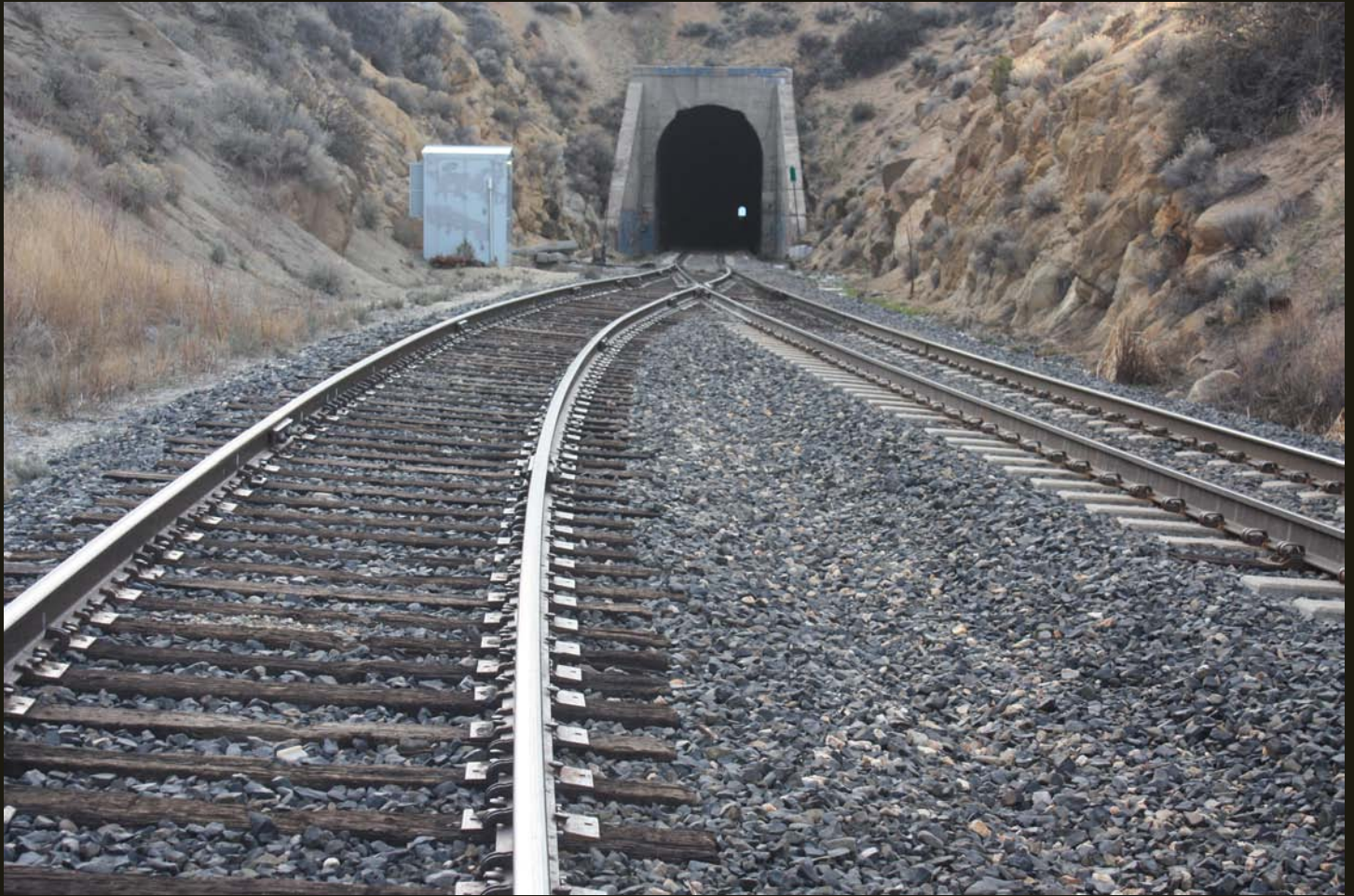
In 1906, the WP built the Chilcoat Tunnel beneath Beckwourth Pass at the high point of its Feather River Route. In this view of the east entrance to the Chilcoat Tunnel, the 1906-1907 WP mainline is on the right, with upgraded welded rails and concrete ties, and the 1917 siding is on left with bolted rail and wooden ties.
