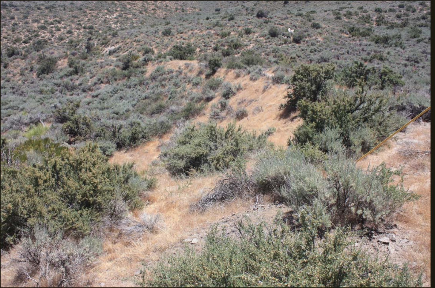
Southeastward view of the SV (1896) fill grade on the hillside on the southern shoulder of Beckwourth Pass.
