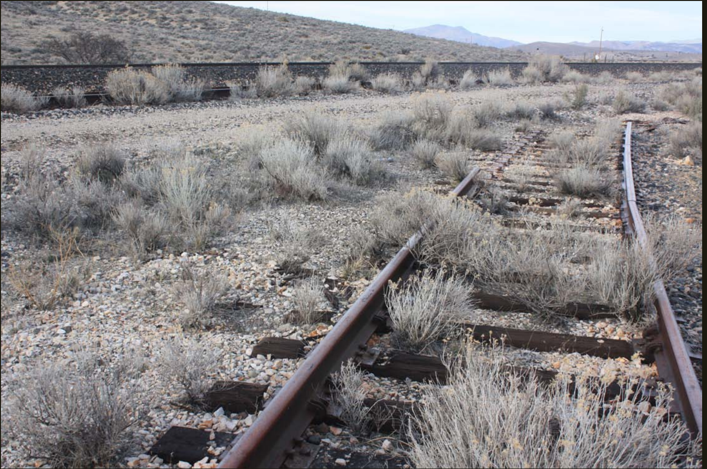
This is the east branch of the Reno Junction wye, which once connected with the WP siding here. This switch has since been removed; note the end of the siding in the brush to the left (seen better in the previous photo). The active WP/UP mainline towers above all.
