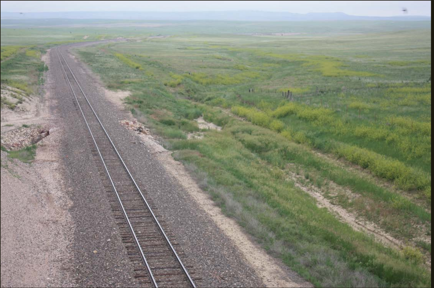
Southward view of the C&N line (now BNSF) at same location as previous photo.
