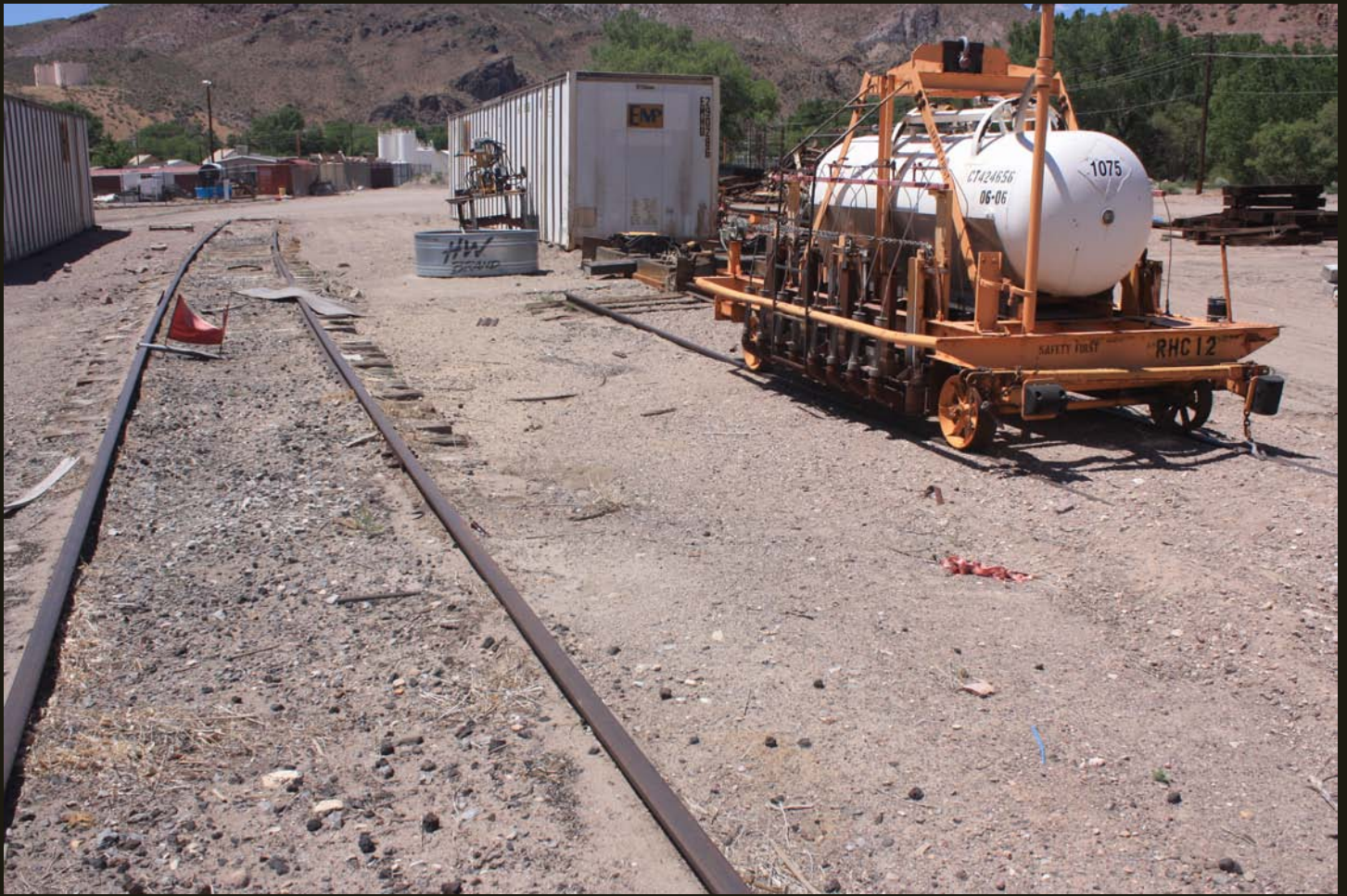
Northwestward view of the C&P (1907), same location as previous, showing the current end of track. The north tip of a wye may have once been present in this view.
