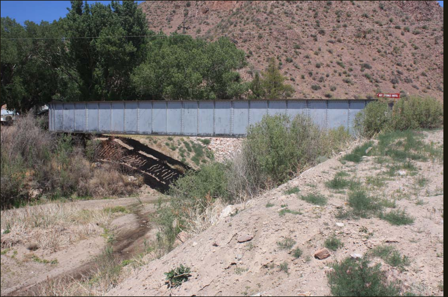
Another view of the bridge over Clover Creek.
