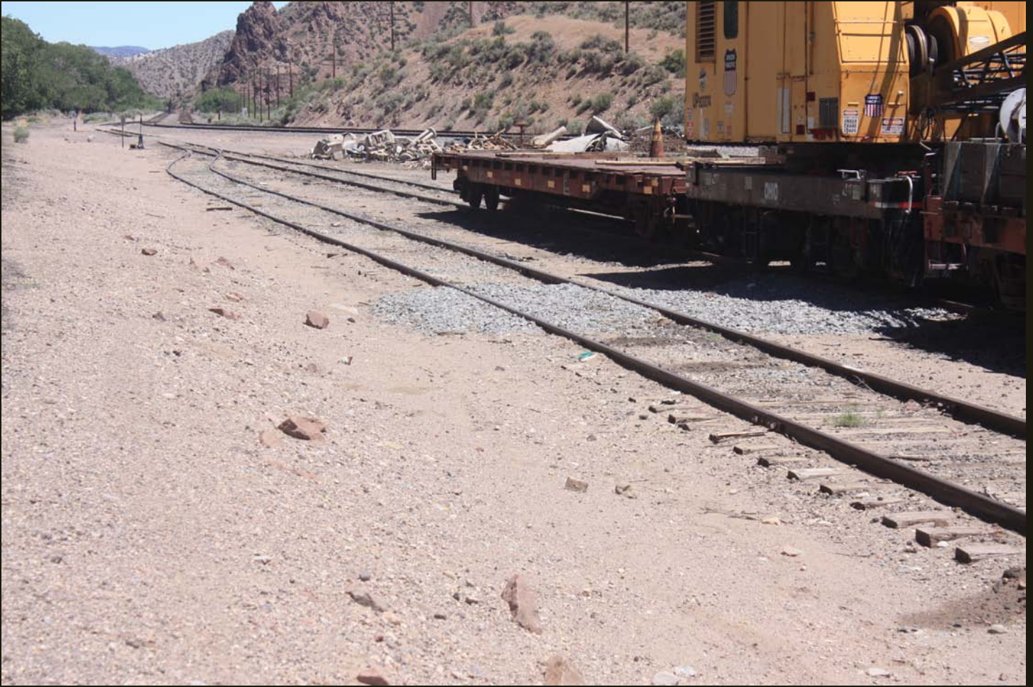
Eastward view of the C&P (1907), showing the switch and siding in the foreground. The junction with the mainline is in the left distance.
