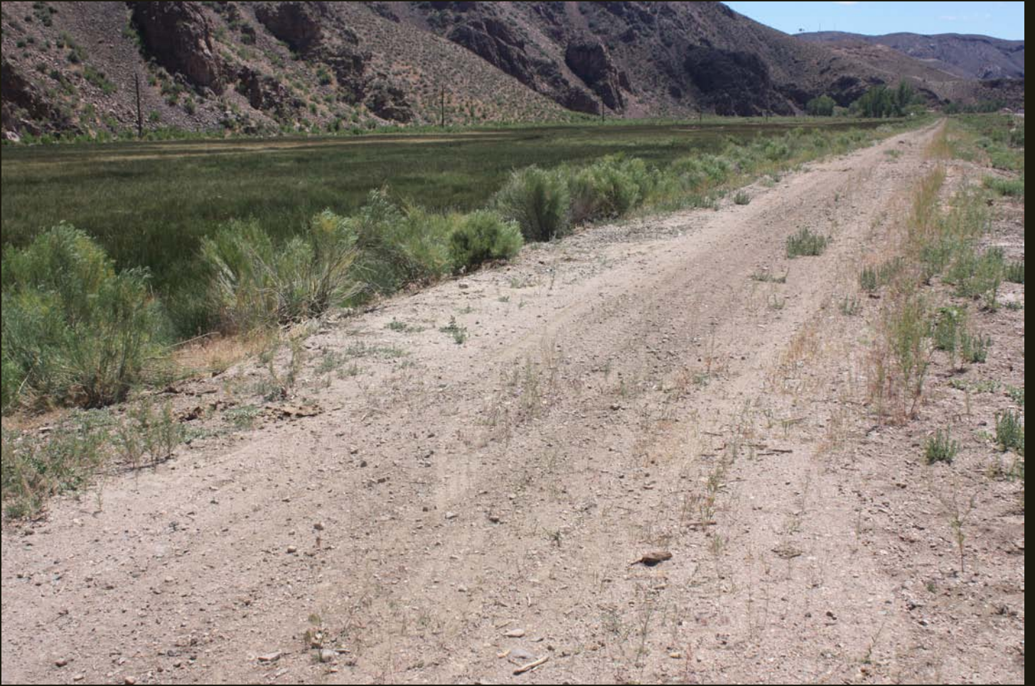
Southward view of the C&P (1907) alignment, one mile north of Caliente. The green area is Meadow Valley Wash, which the railroad follows almost all the way to Pioche.
