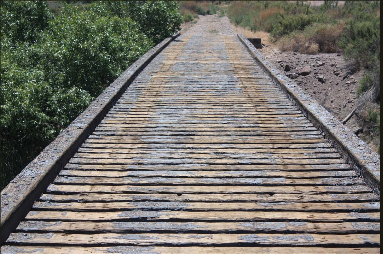
Northeastward view a quarter mile northeast of previous location, showing a small bridge over Meadow Valley Wash on the C&P (1907). The bridge still bears the scars of the rails and spikes that were removed in 1985.
