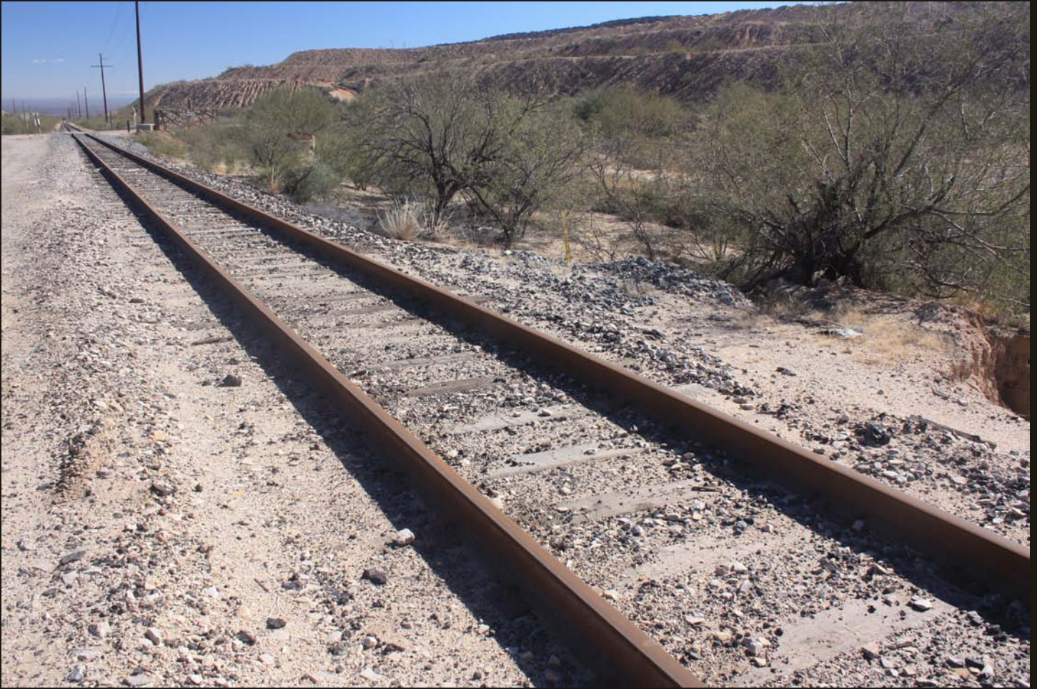
Eastward view of the Pima Spur, 5.5 miles west of the junction with the TB (1906) line at Pima and less than a mile shy of the end of track. The stored tank cars of the previous photo are barely visible in the distance, and the tailings are piled high to the right (north) of the line.
