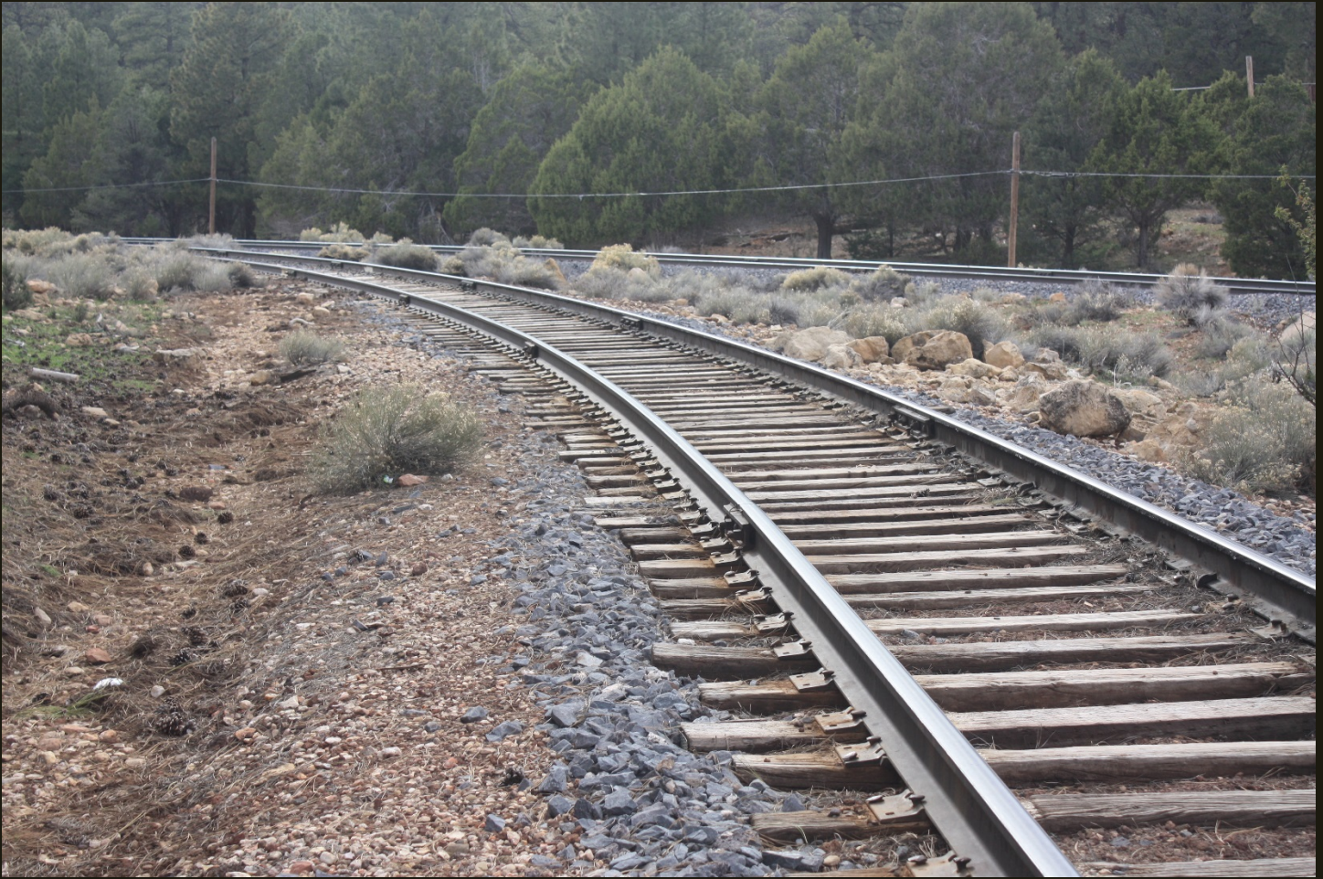
Northwestward view 800 feet northwest of the tip of the wye (previous location). The west branch of the wye is in the foreground and the GC (1901) mainline is in the distance.
