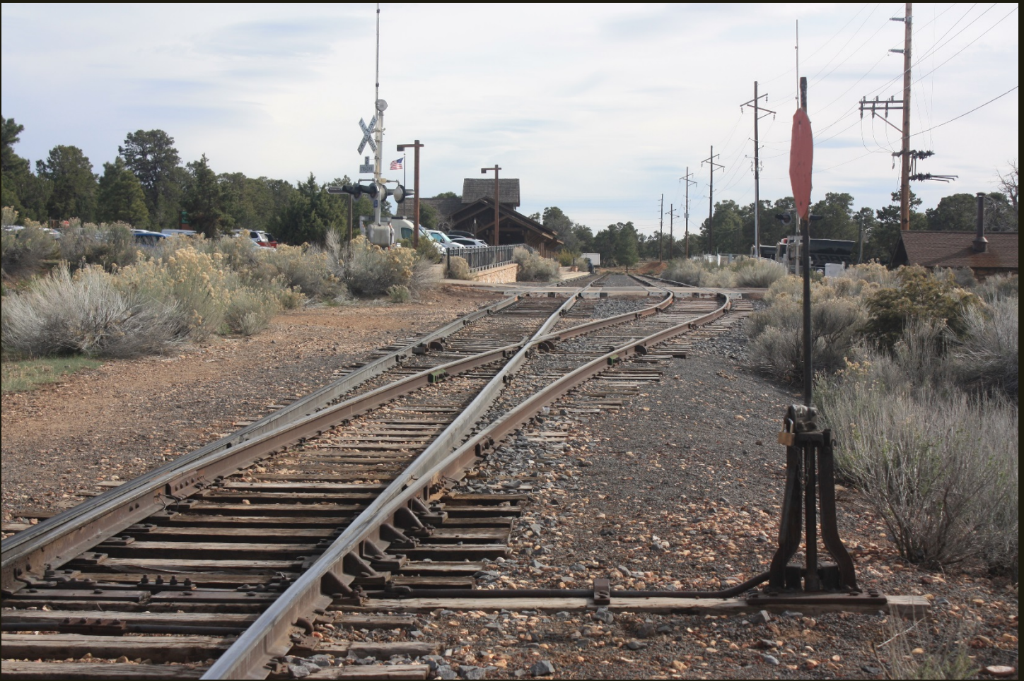
Southward view, 300 feet south of the tip of the wye (previous photo), where the track splits off a siding. Same building as previous photo to the left (east) of the track. The end of the turning wye track is 1,500 feet in the distance.
