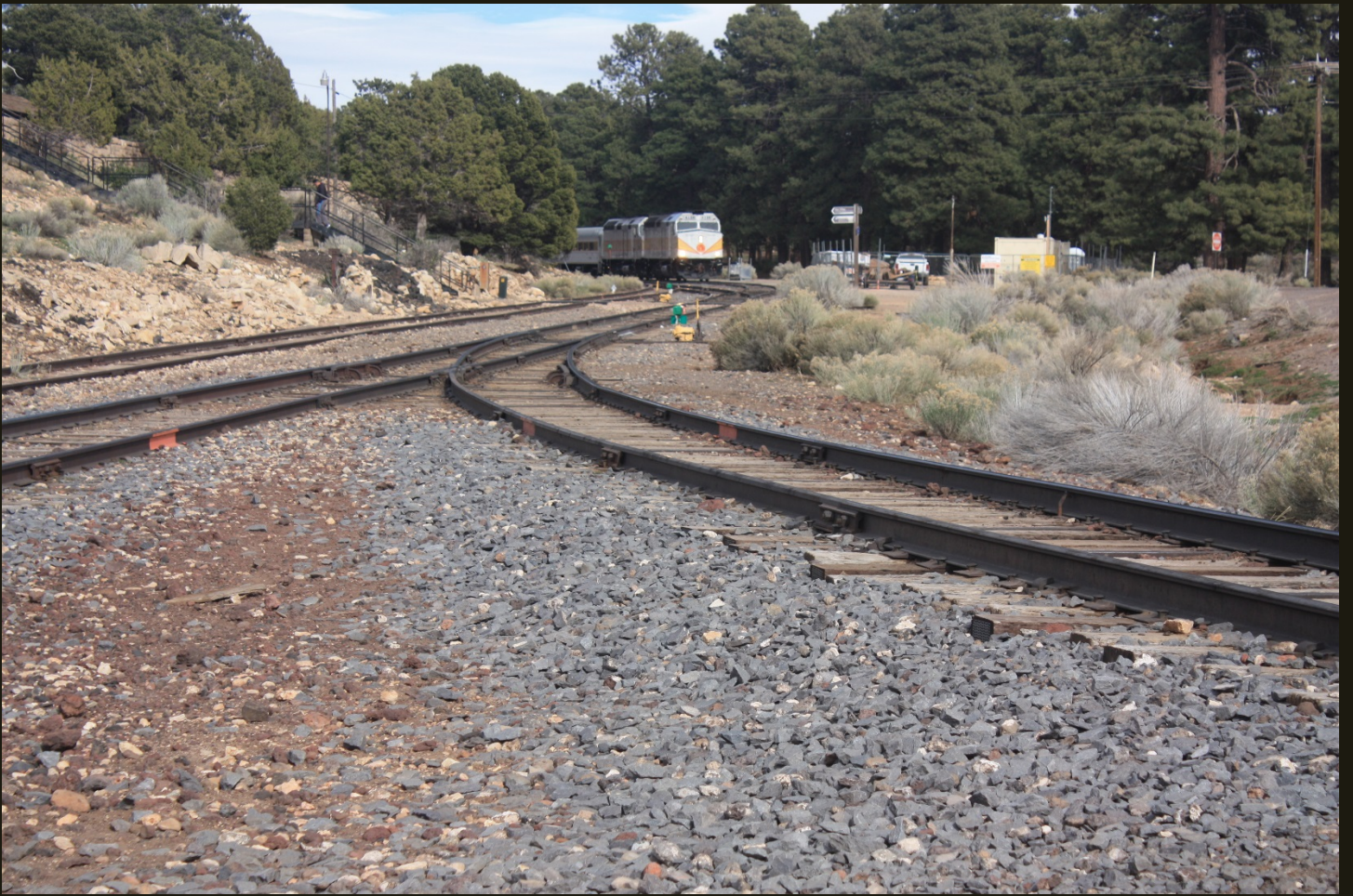
Eastward view of the switch for the east branch of the turning wye. The yellow and green switch is the same one seen in the first photo
