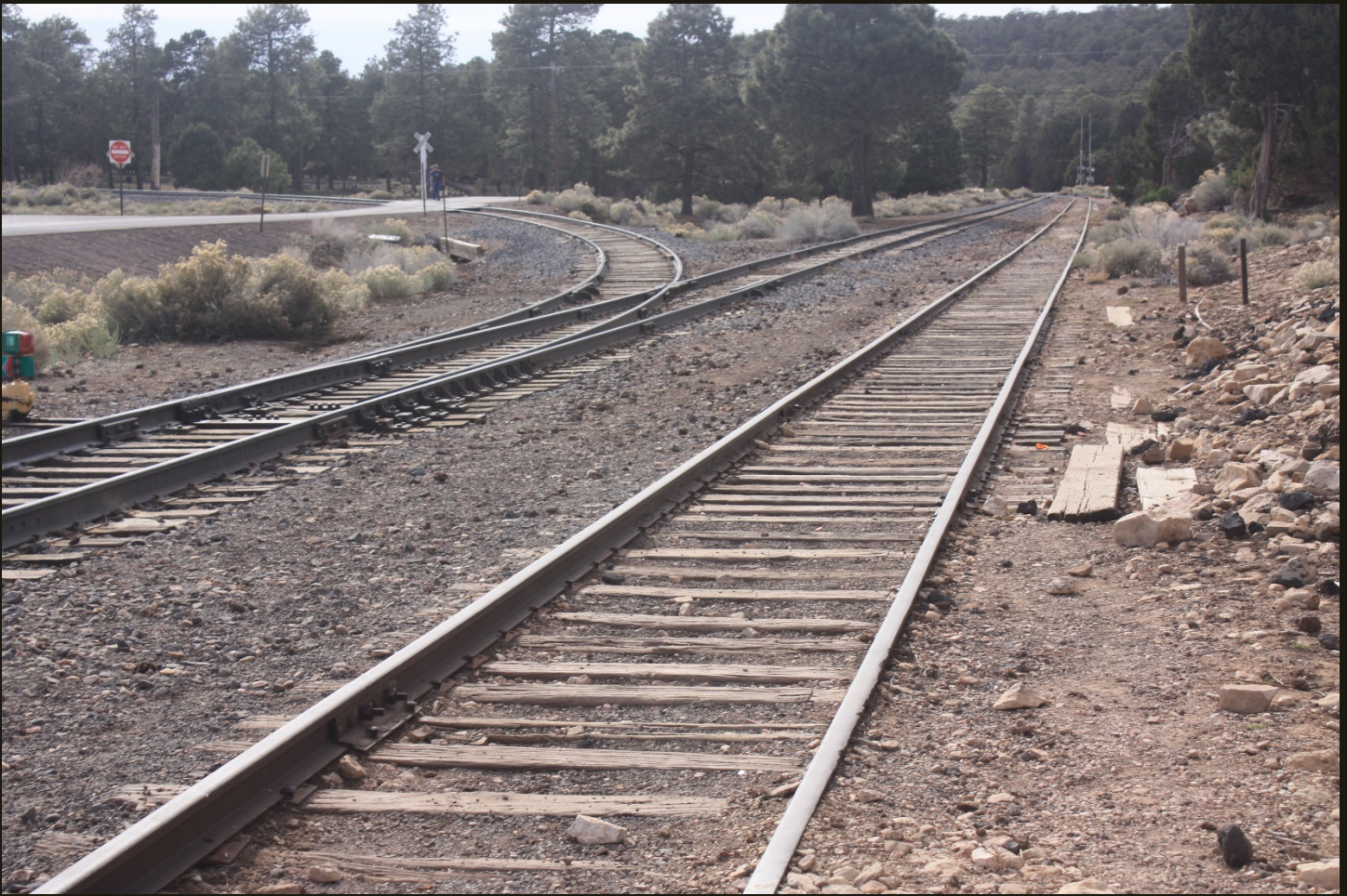
Westward view at the same location as the first photo. The switch for the east branch of the turning wye is on the far left. The wye is on the south side of the GC (1901) alignment, which runs east-west (parallel to the canyon rim) here and turns southward toward Williams in the distance.
