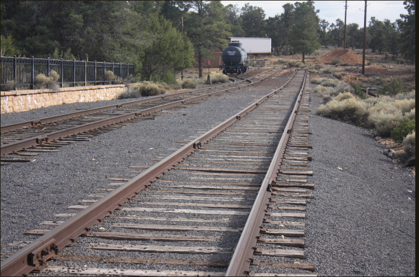
Southward view of the turning wye end-of-track, same location as previous.
