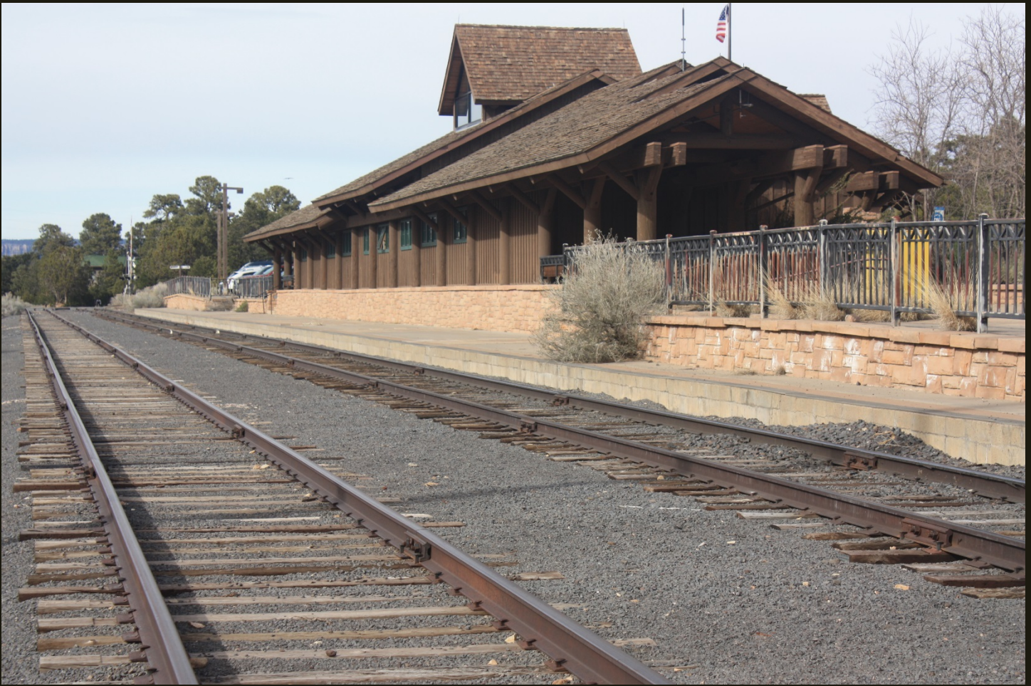
Northward view of the building noted in the previous two photos. This building houses the Grand Canyon National Park River Permits Office and Backcountry Information Center. It appears to be a historic building for railroad loading, but I could find no information on its history.
