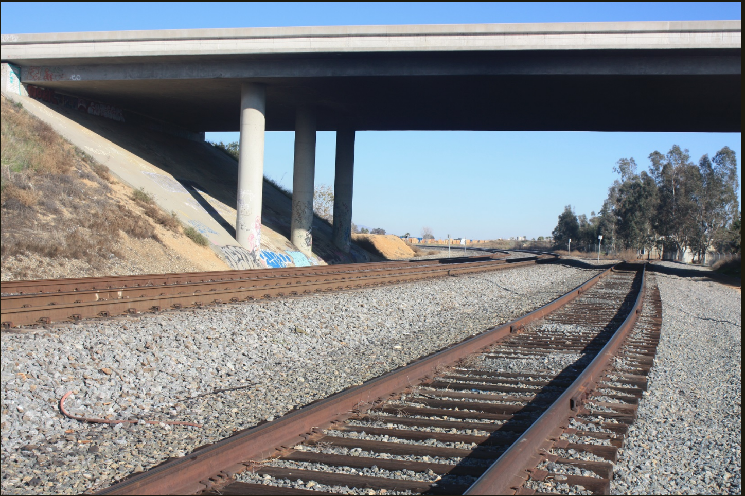
Eastward view of the SP Sunset Route (1881) at its summit in the San Geronio Pass area, same location as previous. The welded double track with concrete ties is on the left and the bolted siding is in the foreground. The east branch of the turning wye was within this view to the right (south) of the siding. Again, there is no trace of the wye, which was used to turn helper steam locomotives at the top of grade. In the right distance, the siding curves to the right to serve a (former?) customer. The overpass is for California Highway 79, which in 1942 was a level grade crossing.
