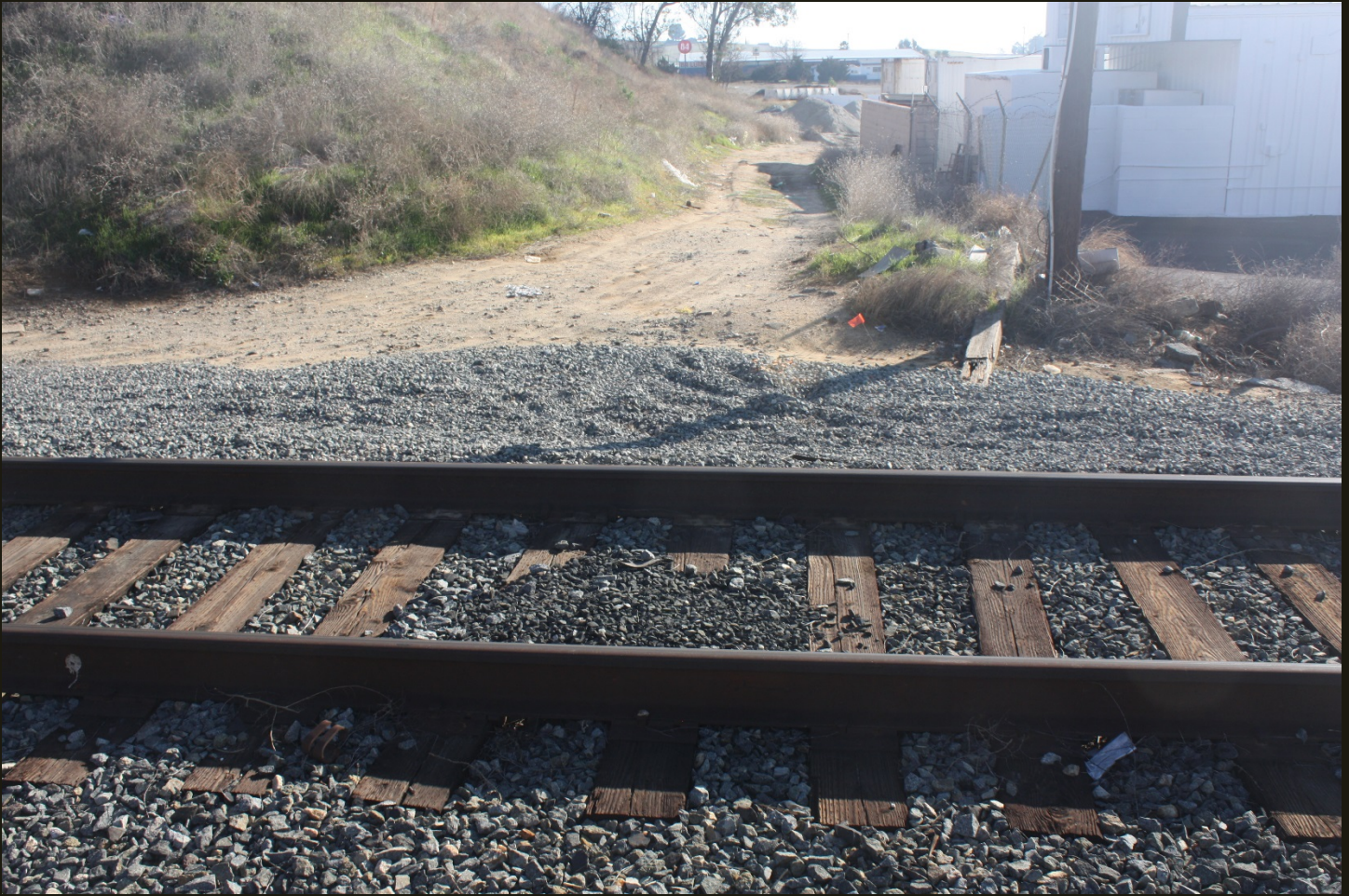
Southward view of the bolted siding on the SP Sunset Route (1881), same location as previous. The dirt path in the center is on or within a few feet of the center of the turning wye; the two wye branches once converged at the far end of the path and the straight track beyond ran just feet west of California Highway 79 (the embankment to the left of the path is for the current Highway 79 overpass). Just when I thought there was no evidence whatever of the turning wye, I noticed the discarded tie on the ground just to the left of the utility pole; we'll take a closer look at that tie in the next photo.
