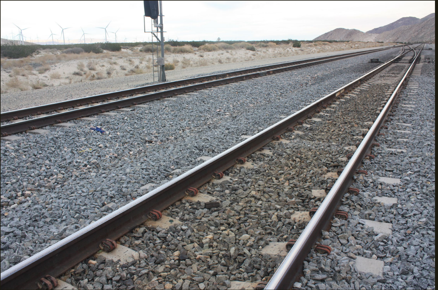
Eastward view of the SP Sunset Route (1881) same location as previous. The signal to the left of the track is the closer of the two signals in the previous photo. The switch and crossover track are in the right distance. The grade continues downward to the Salton Trough, where the SP grade descends below sea level about 30 miles down the line.
