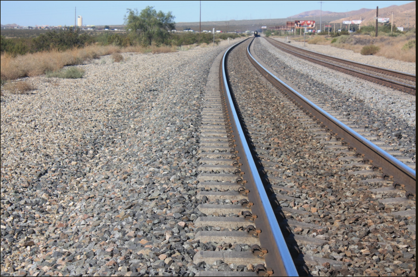
Westward view of the SP Sunset Route (1881) 16 miles east of grade summit at San Geronio Pass. There is welded double track with concrete ties, just like at the summit. The tall building in the left distance is the Morongo Casino, the billboards to the right of the tracks are along Interstate 10, and the Big Boy is steaming toward us on the nearer of the two tracks. Note the desert vegetation, on the rain shadow side of the Pacific Crest, very different from the grassland and chaparral at the pass.
