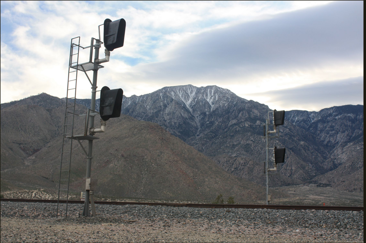
Southward view of the SP Sunset Route (1881) 3 miles east of the previous location and looking southward at 10,834-foot Mount San Jacinto. Mount San Jacinto is the north end of the Peninsular Range geologic province, which extends southward to the tip of Baja California, and borders the south side of San Geronio Pass. These signals guard a switch for a crossover track on the UP double-tracked mainline.
