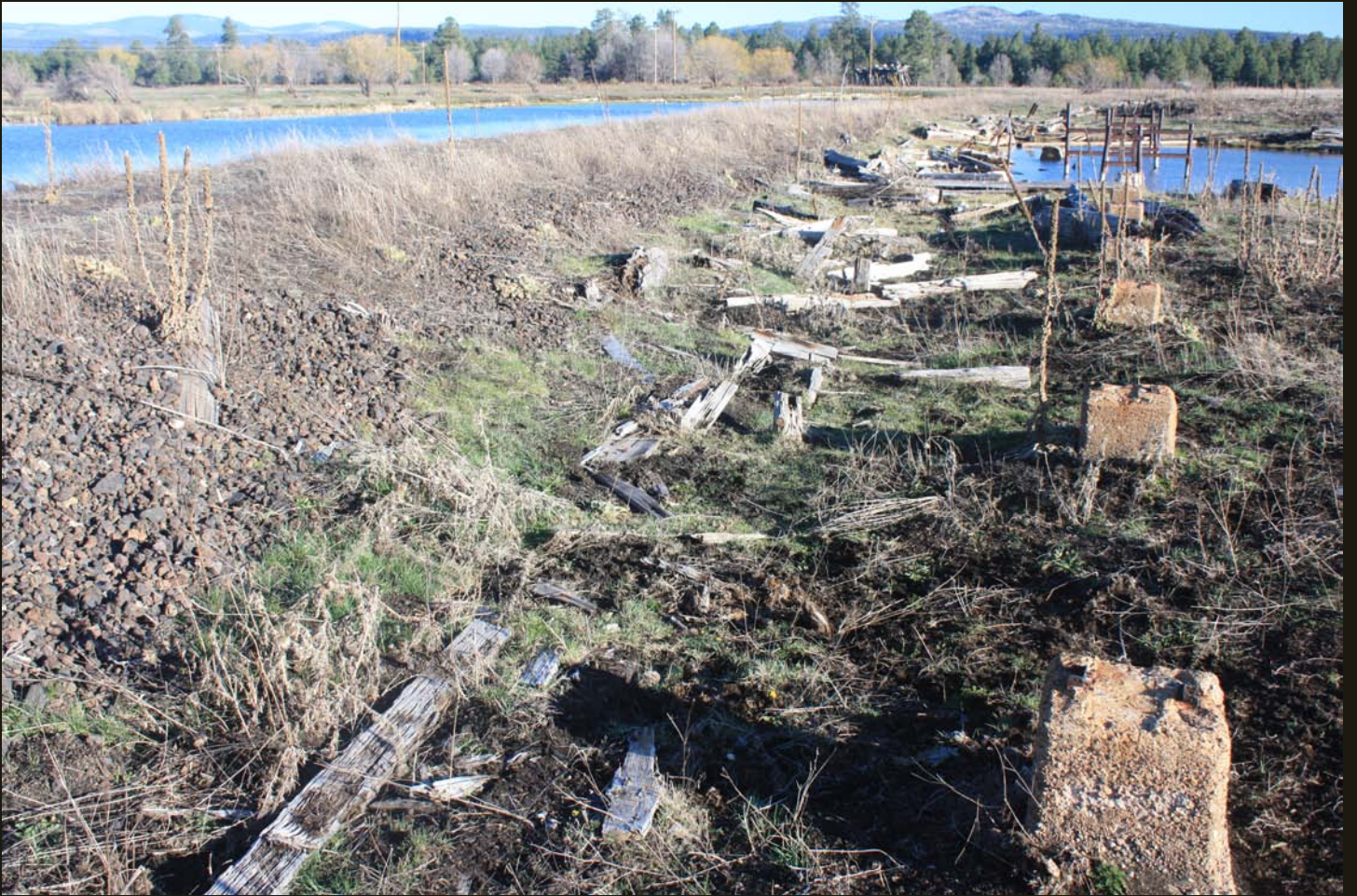
Closer view of discarded ties and foundations for a loading facility along the abandoned Apache Railway at its 1920 end-of-track at McNary.
