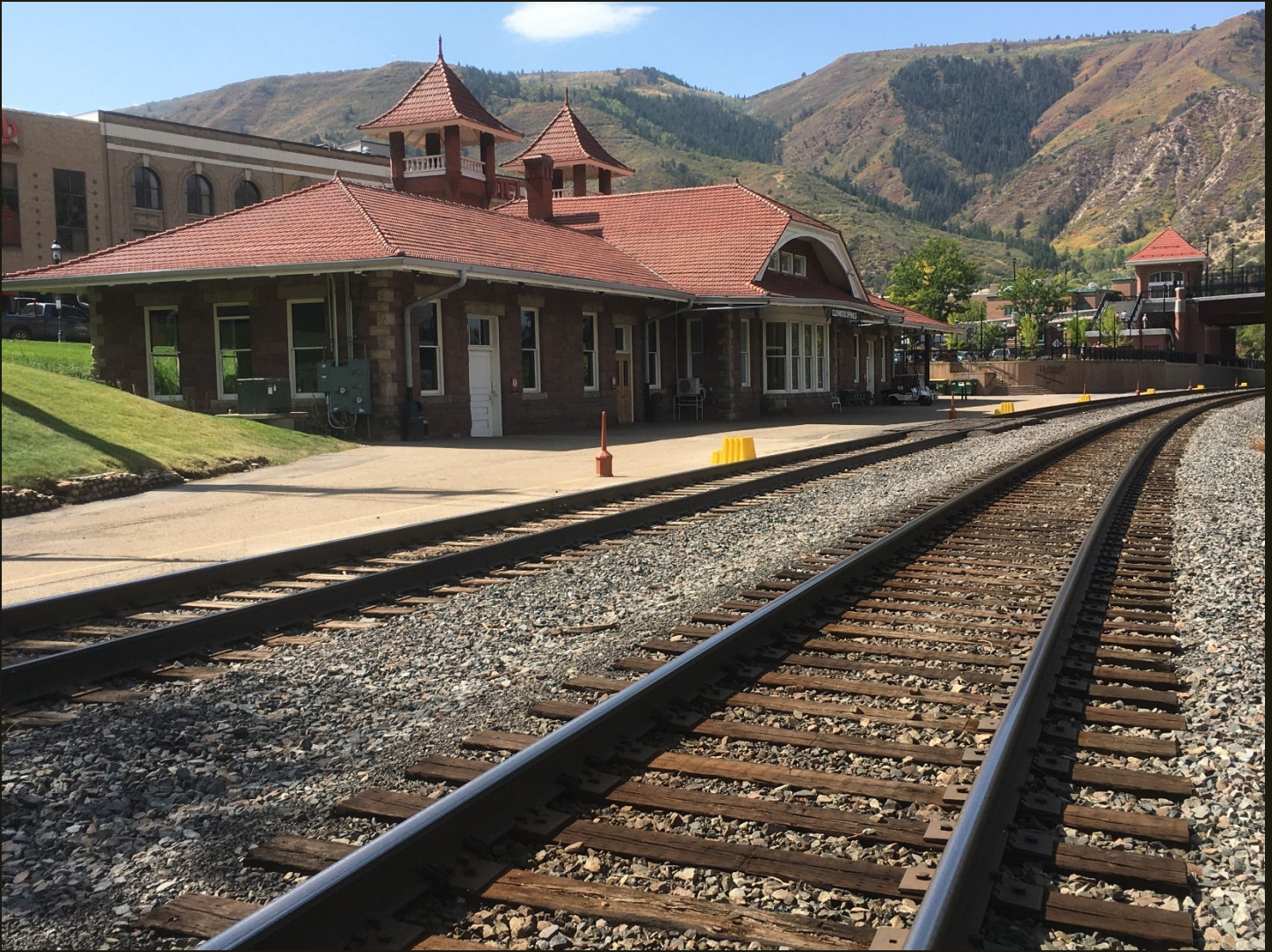
Westward view of the D&RG Aspen Branch (1887n) at the Glenwood Springs Depot. The D&RGW built the Depot in 1904. The building is composed of brick and red sandstone, the entrance is flanked by medieval-inspired brick towers with pyramidal roofs, and the Glenwood Railroad Museum now occupies the former Ladies' Waiting Room. The Depot is served by several Amtrak trains, including the California Zephyr, which runs between Chicago and the San Francisco Bay Area, and also by Greyhound busses. According to the Amtrak Fact Sheet (Colorado), Fiscal Year 2016, Glenwood Springs was the second busiest of the nine Colorado stations served by Amtrak. The track on the right is the mainline and the track on the left is a siding that serves the Depot.
