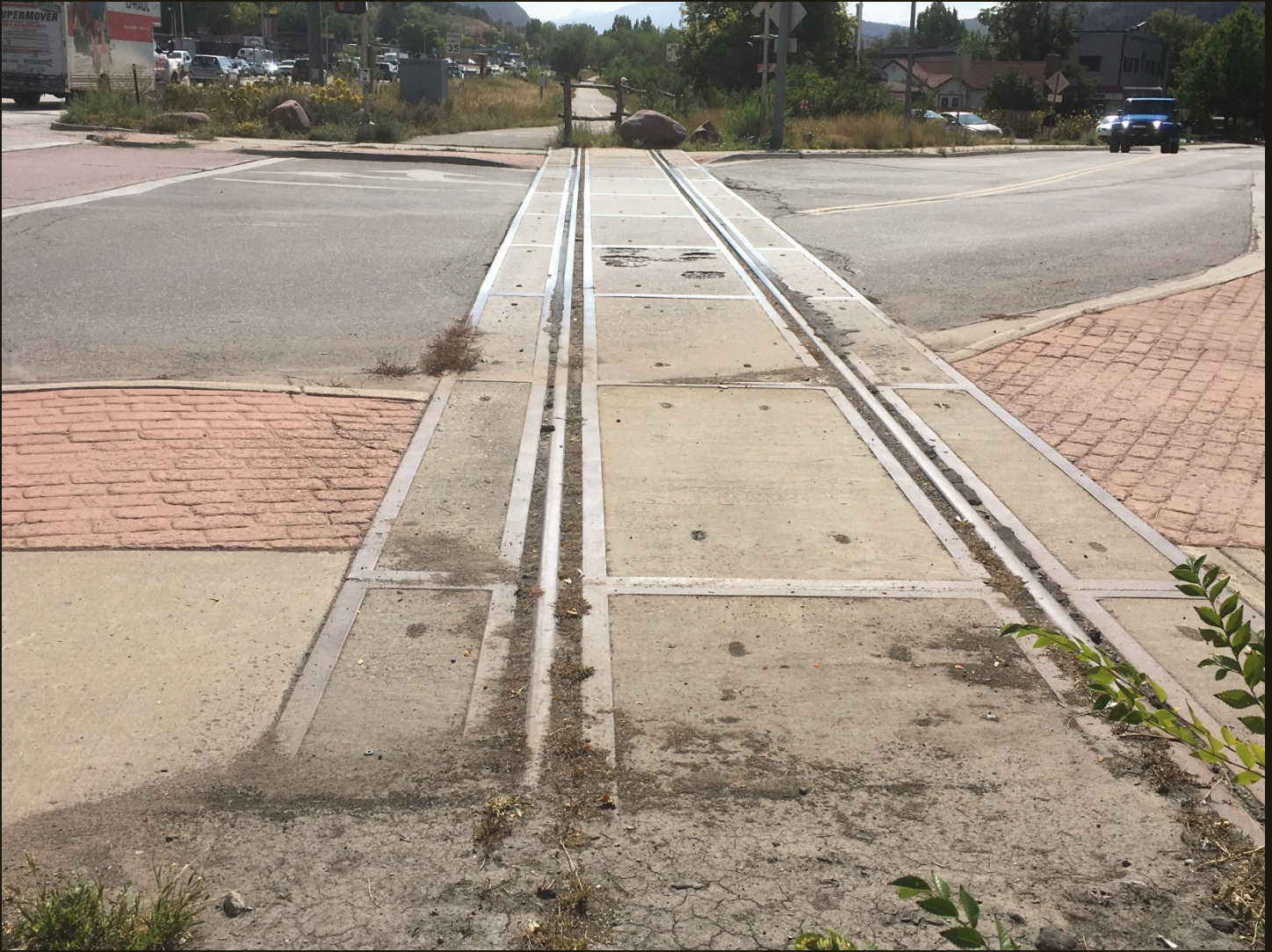
Southward view of the D&RG Aspen Branch (1887n) and Rio Grande Trail 100 feet south of the previous location. The tracks in the roadbed are still in place and are the southernmost tracks. Across the street, the Rio Grande Trail is on the railroad grade and continues to be from here to Aspen.
