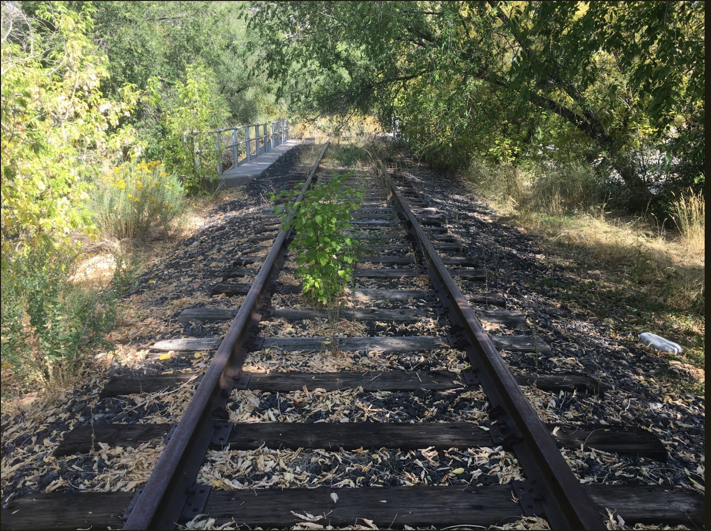
Northward view of the west branch of the wye for the D&RG Aspen Branch (1887n) at the same location as previous. The bridge carries the grade over 7th Street.
