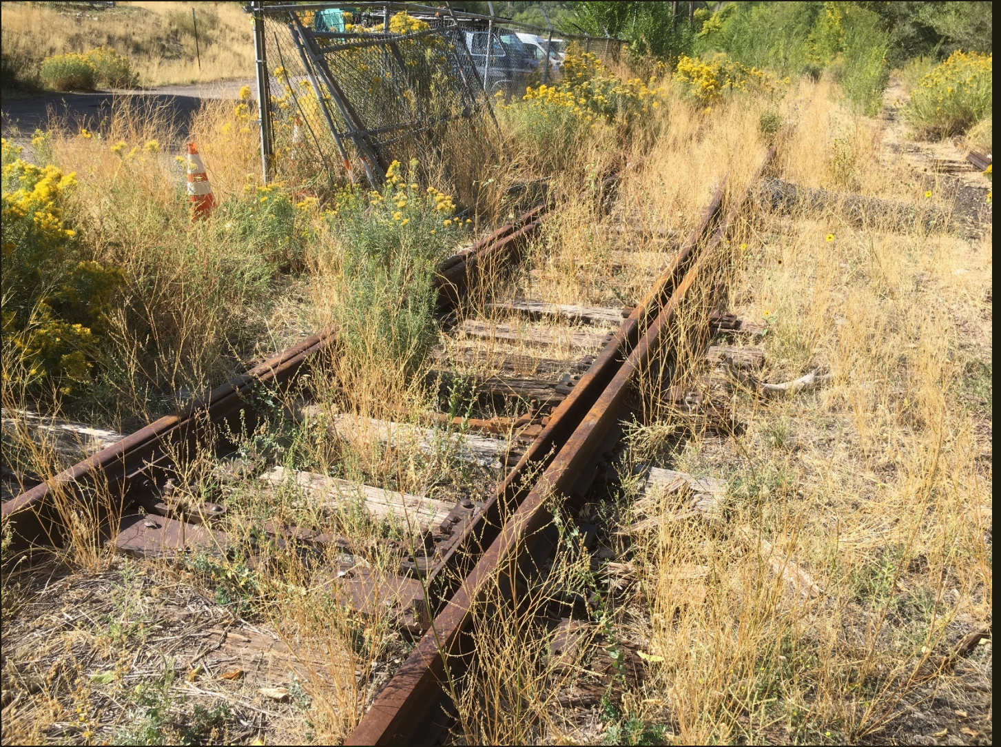
Southwestward view of the east branch of the wye for the D&RG Aspen Branch (1887n) 100 feet southwest of the previous location, where the line splits into three tracks.
