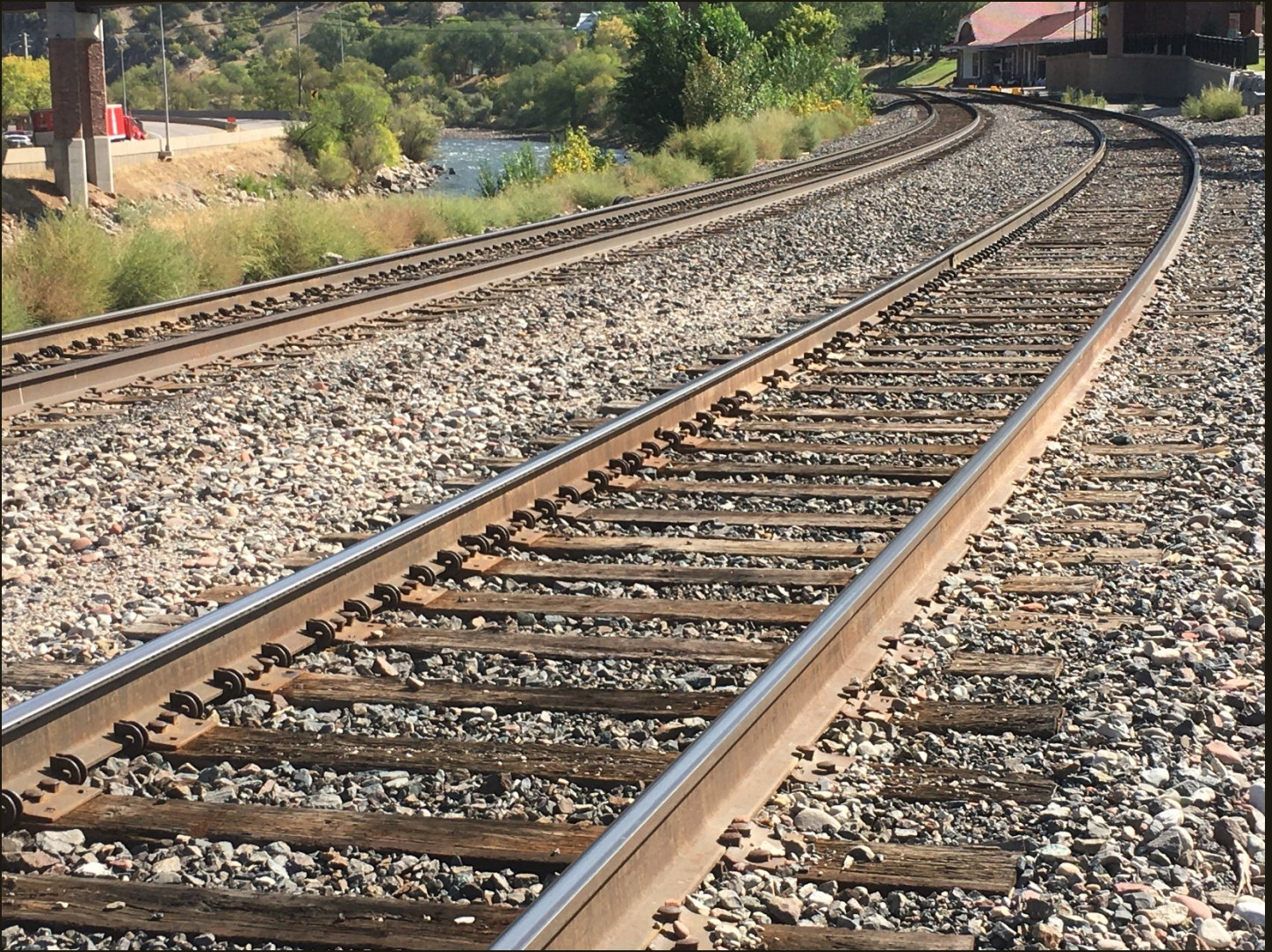
Eastward view of the D&RG Aspen Branch (1887n) 500 feet west of the Glenwood Springs Depot, which is visible to the right of the tracks in the distance. The Colorado River is to the left of the tracks.
