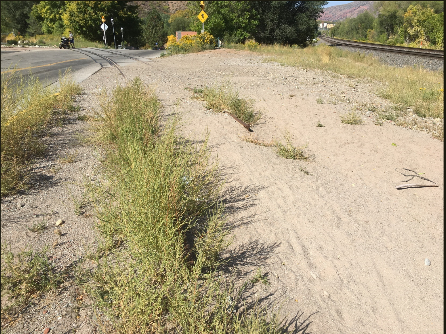
Westward view of the D&RG Aspen Branch (1887n) a few steps south of the previous location. The east branch of the wye for the line to Aspen is in the foreground and the mainline is in the upper right portion of the photo. In 1995, all operations ceased on the D&RG Aspen Branch and around 2006 the 42-mile grade from Glenwood Springs (this location) to Aspen was converted into a rail-to-trail called the "Rio Grande Trail" in honor of the D&RG. Tracks remain only at the wye, which as seen here is now completely detached from the mainline.
