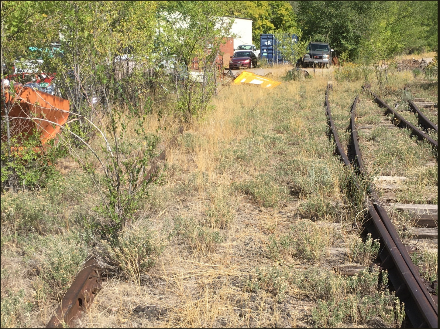
Northward view of the D&RG Aspen Branch (1887n) 200 feet north of the tip of the wye (previous location). The track in the foreground is the west branch of the wye and the track on the far right is the east branch; the two tracks have been virtually parallel from the tip of the wye (previous location) to here. A crossover track connects the two branches of the wye.
