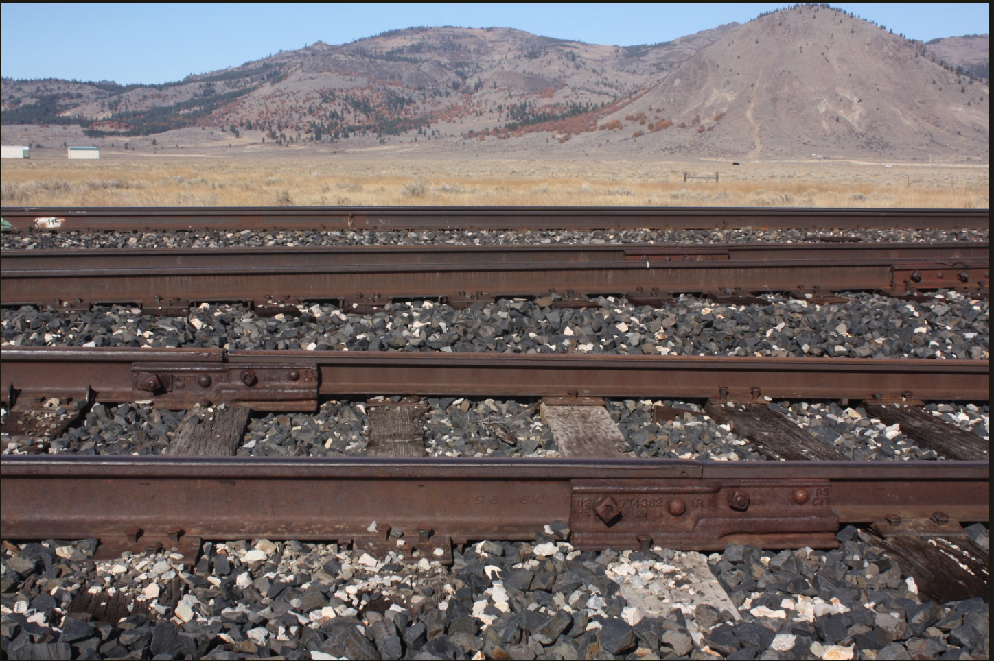
Northward view, same location as previous. The tracks from nearest to farthest are the B&L (1901)/WP Loyalton Branch, the siding for the branch, and the WP (1909) mainline.
