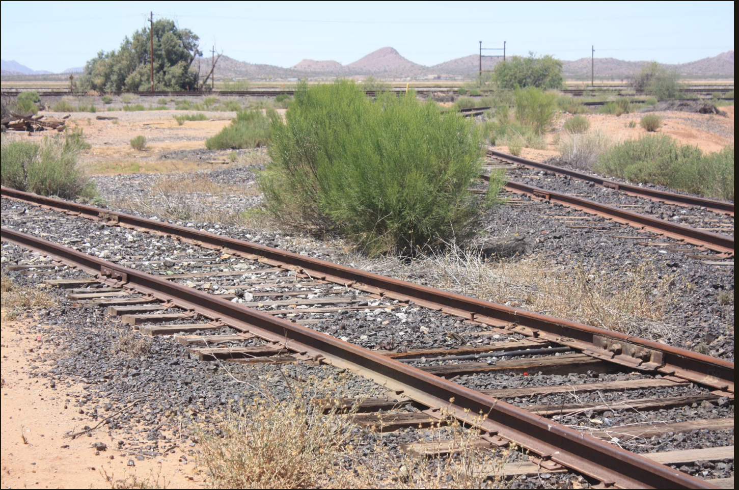
Both legs of the MA wye at Magma, with the MA siding and P&E mainline and siding in distance.
