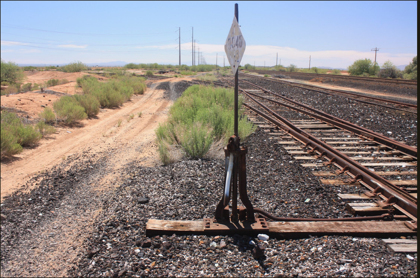
A few steps back from the previous, showing the switch for the northern leg of the MA wye, where it joins the eastern of the two MA sidings. The P&E siding and mainline are to the far right (west).
