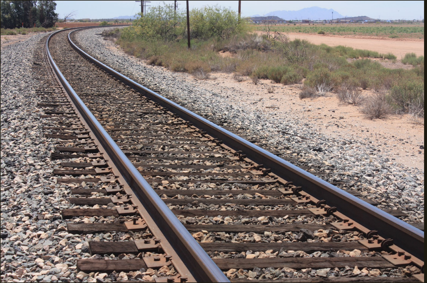
Southward view of the SP (1924) Phoenix connection where it veers south. Note the fresh granite ballast, rust-free welded rails, and clips (in addition to spikes) of a modern, active line. From here, the 1924 SP route continues 30 miles to the SP (1881) mainline.
