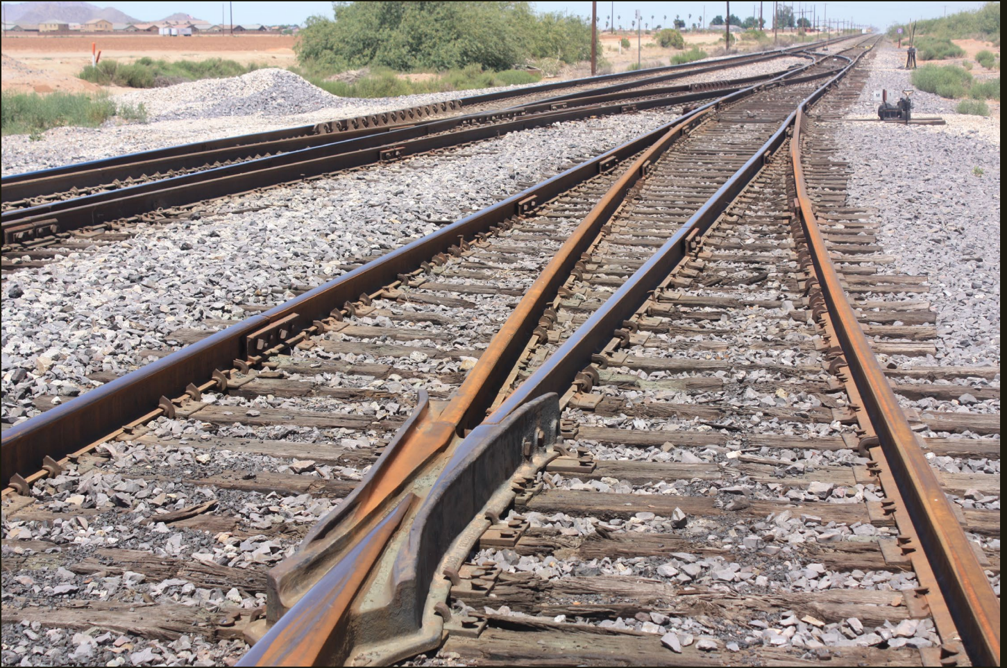
Now we are just north of the stored cars, looking north. In the foreground, the rusty P&E siding joins the P&E mainline (with the stored cars just behind the viewer), and on the far left the 1924 SP Phoenix connection has a double switch to the P&E.
