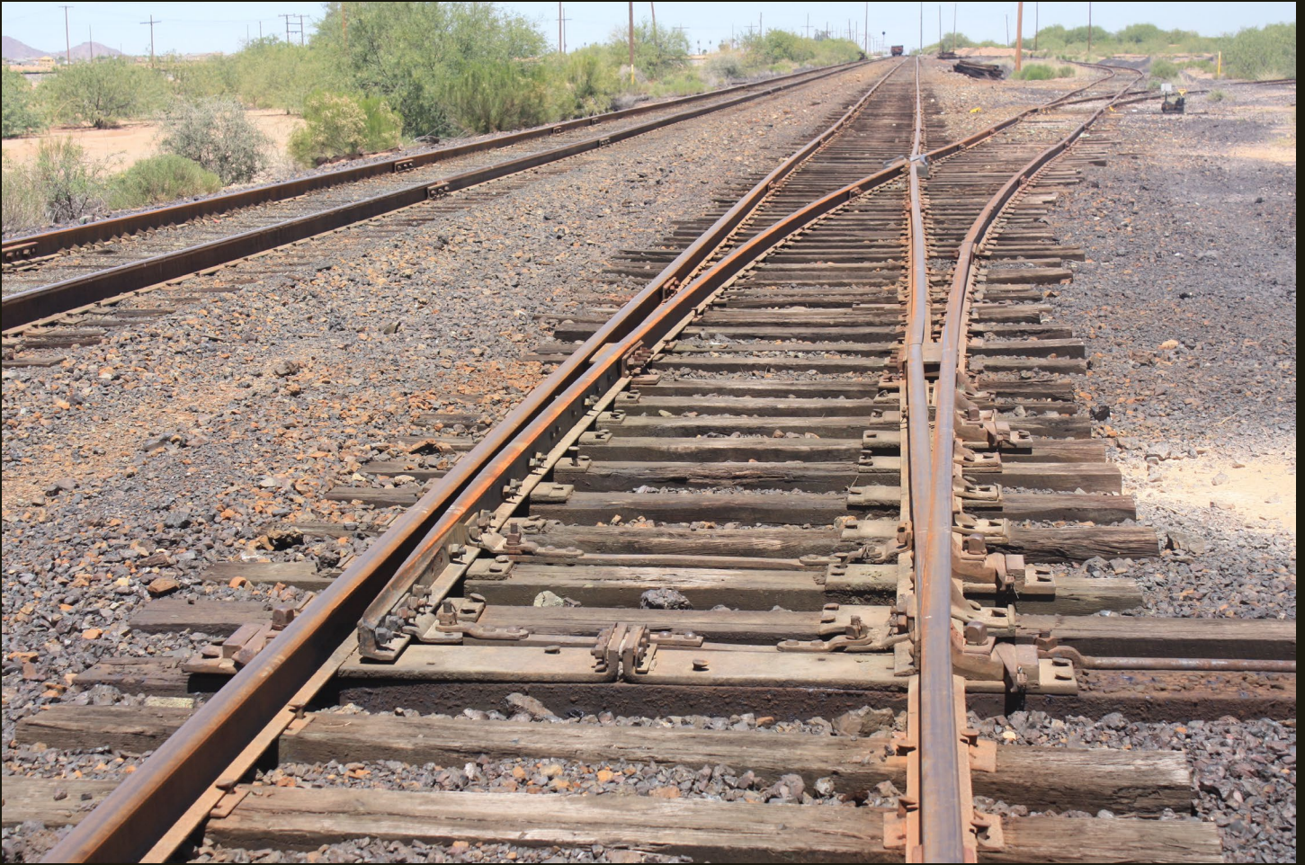
Another northwestward view of the MA wye. The P&E siding is in the foreground and the MA siding veers right to a switch with the southern leg of the MA wye.
