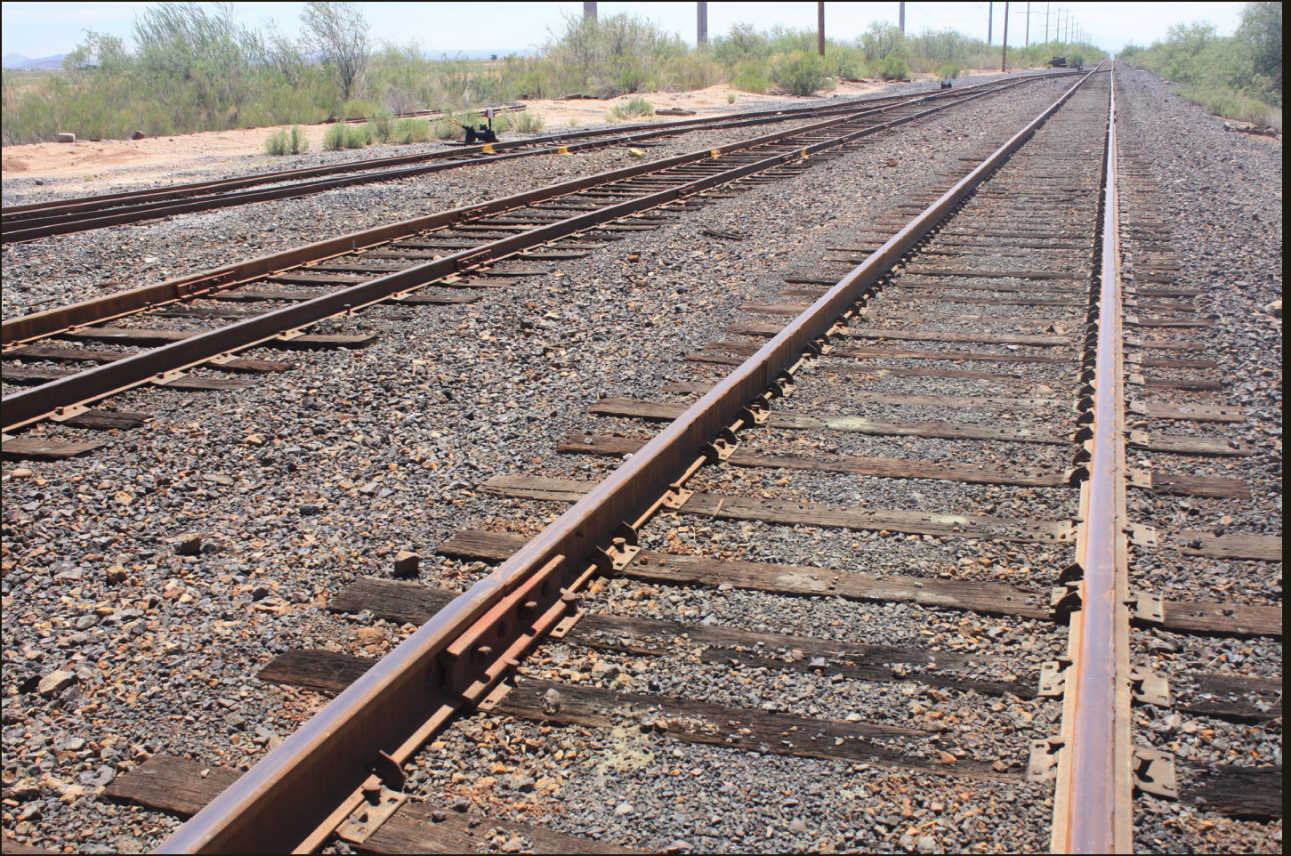
Southeastward view at about the same location as previous, from right to left the P&E (1904) mainline, the P&E siding, and the MA (1915n) siding with a switch to the south leg of the MA wye.
