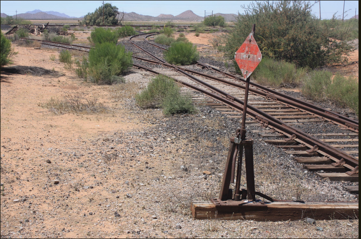
The apex of the MA wye, with the MA siding and P&E mainline and siding in distance.
