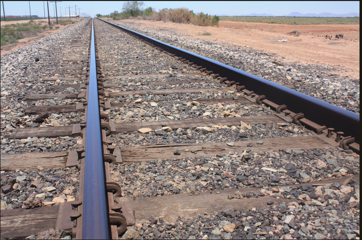
Northward view, same location as previous 2 miles north of Magma. From here, the P&E (1904) grade, sporting its 1924 and subsequent SP upgrades (the welded rail came later than 1924), continues 40 miles to Phoenix.
