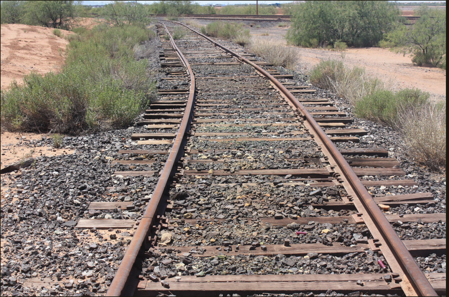
Southward of the south leg of the MA wye. In 1923, these rails were either moved farther apart to standard gauge and or replaced with heavier rail on standard gauge. Note the slight dog-leg in the track, not great construction.
