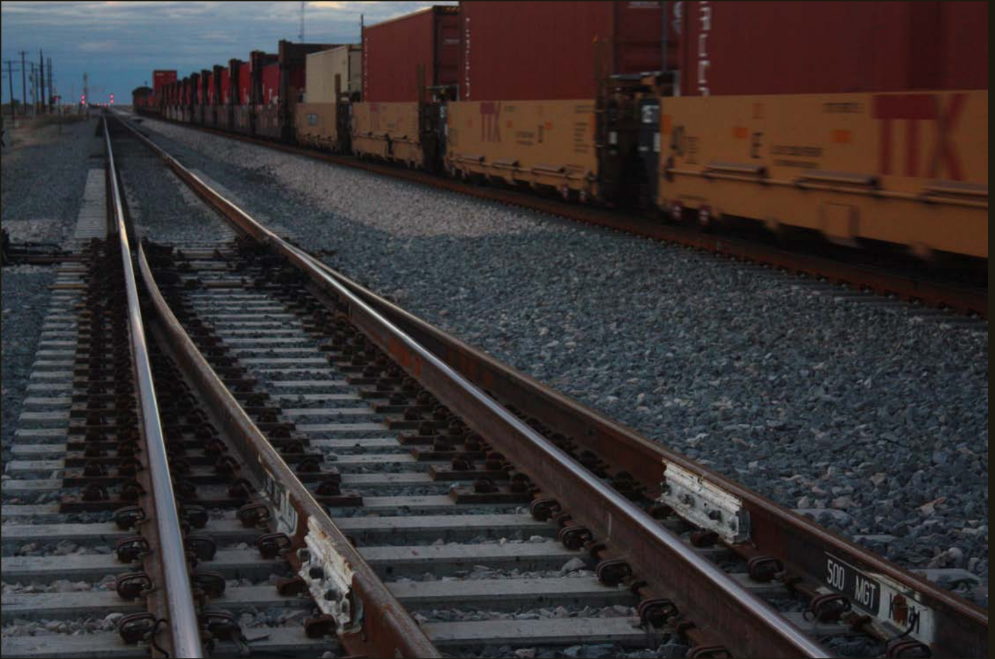
As the train speeds past Niland on the new track, note the older track ties are wooden just past the cross-over.
