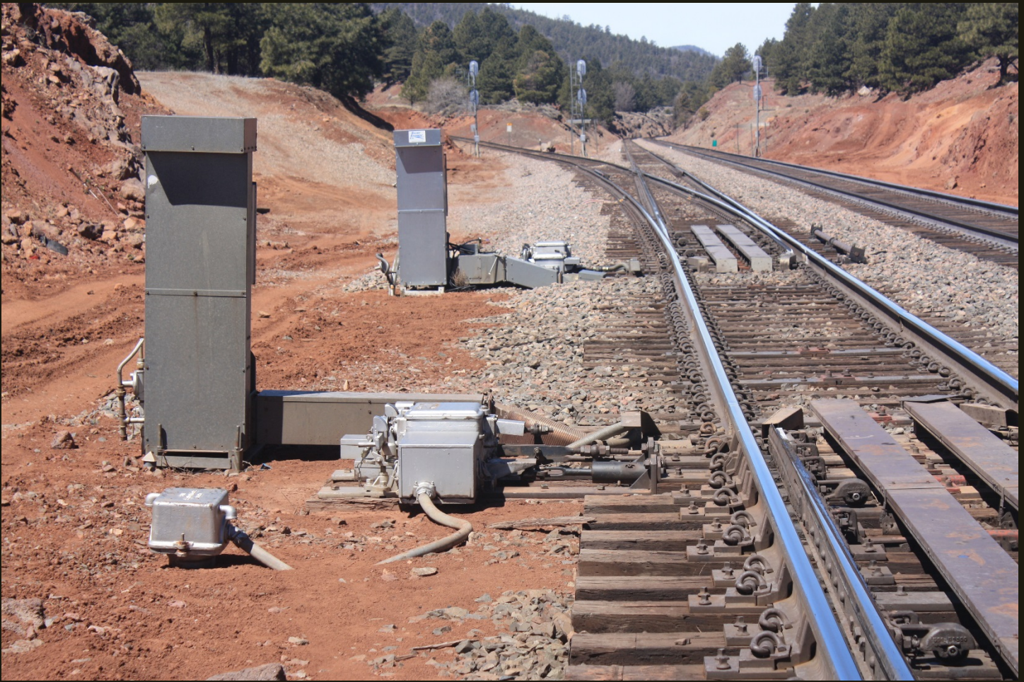
Westward view of West Williams Junction 100 feet west of the previous location. The closer of the two switches is for the crossover track and the second switch is West Williams Junction, the 1960 connector to the A&P (1883) and the SFP&P (1895).
