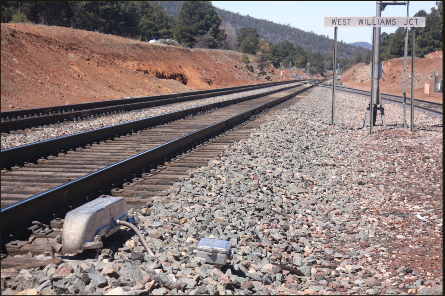
Westward view of the AT&SF (1960) a few steps north of the previous location. The double-track mainline is on the left and the siding that connects to the mainline is behind and just to the right to the sign. Barely visible just beyond the switch for the siding is a junction with a track that curves to the left; that is West Williams Junction, which connects with the A&P (1883) for trains headed to Ash Fork to continue onto the SFP&P (1895).
