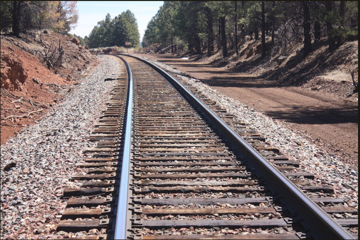
Eastward view 100 feet west of the previous location. The 1960 connector is straightening out in the foreground, meaning it is just about on the A&P (1883) alignment and the dirt road to the right is a service road just off the 1883 alignment.
