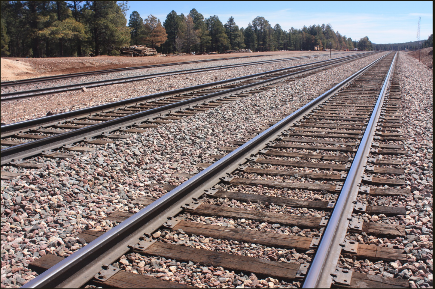
Eastward view of the AT&SF (1960) 800 feet west of the previous location. Note the same tower in the upper right for reference. The tracks are, from right to left, the two mainline tracks, the siding that connects to the mainline, and the outer siding (foreground of first two photos). All these tracks are on the 1960 new alignment; the abandoned stretch of the A&P (1883) is out of sight 100 feet to the right (south).
