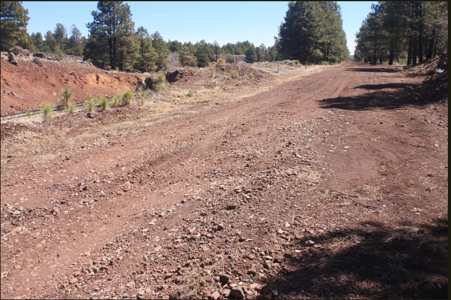
Eastward view 200 feet west of the previous location. The dirt road in the right foreground and extending into the right distance is the A&P (1883). The track on the left is the 1960 connector to the A&P (1883) and the SFP&P (1895).
