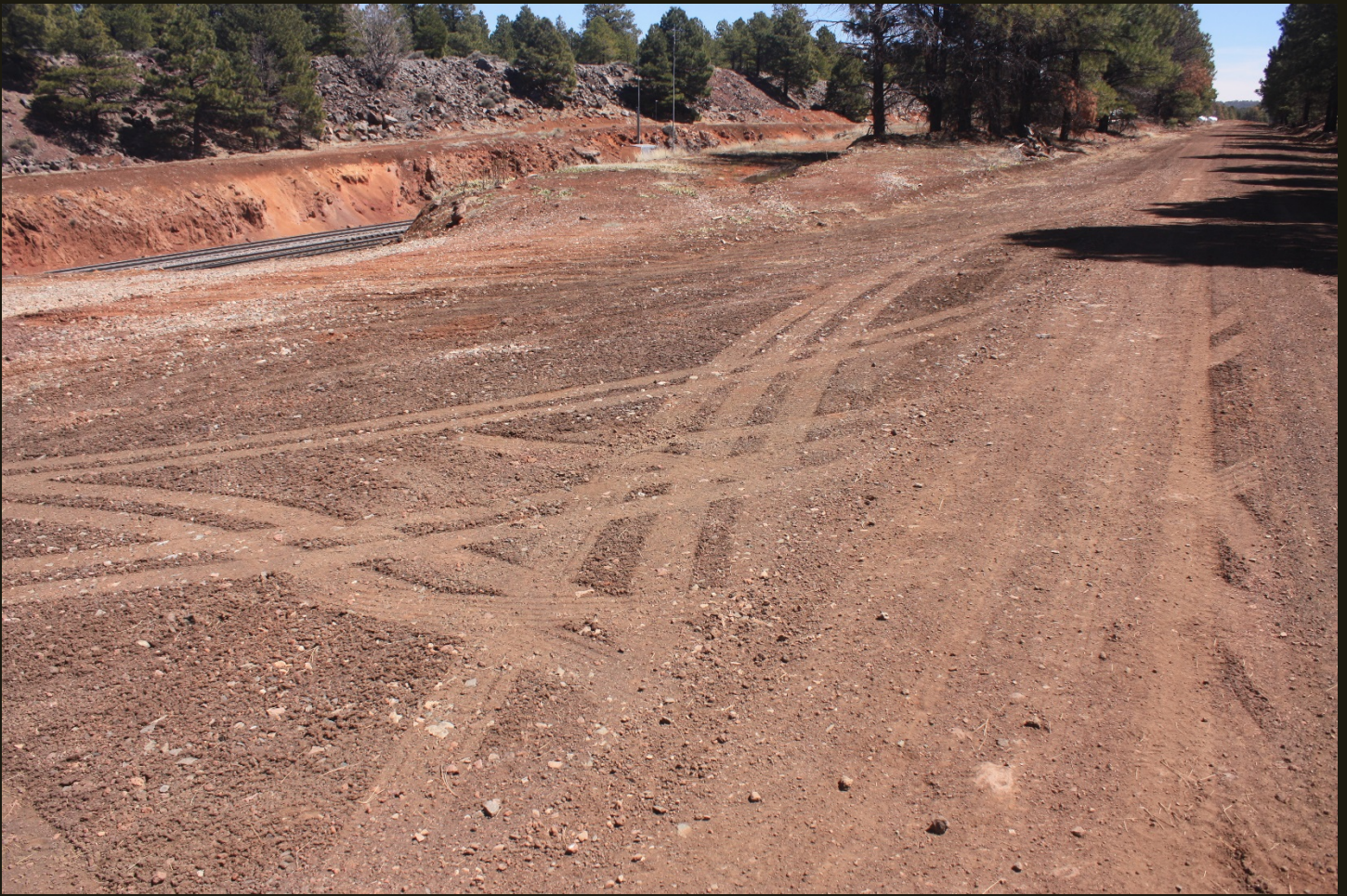
Eastward view 500 feet west of previous location. The dirt road in the right foreground and extending into the right distance is the A&P (1883). The double-track AT&SF (1960) is visible in a cut grade on the left at West Williams Junction; the switch to connect the 1960 mainline connector to the A&P (1883) and the SFP&P (1895) is barely visible in the closer of the two tracks.
