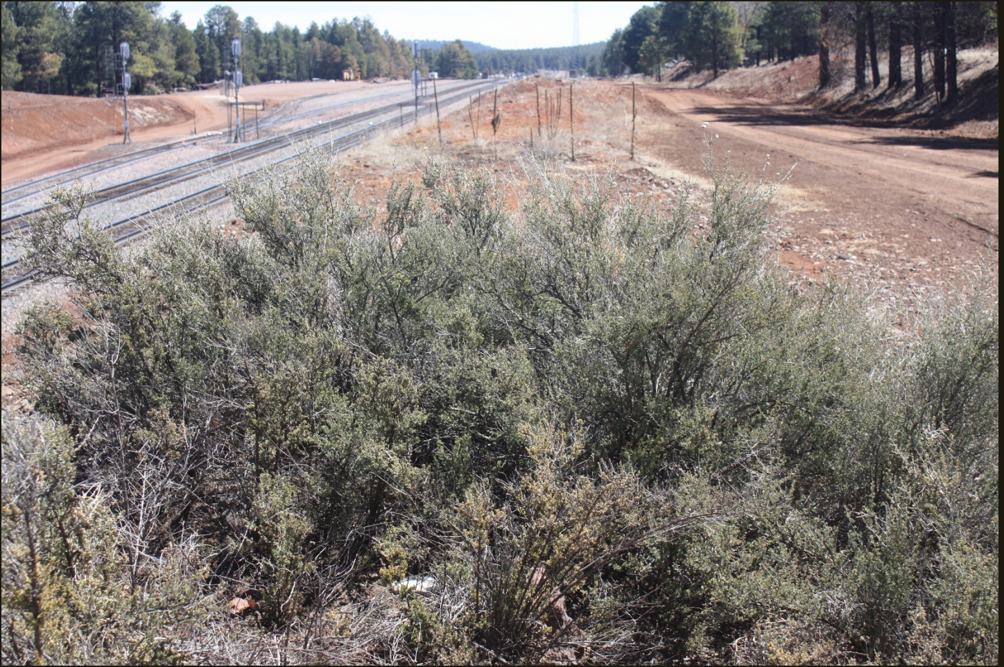
Eastward view 400 feet west of the previous location; the sign for "West Williams Jct." (previous photo) is just on the other side of the center of the three signals in the upper left. The tower is barely visible against the sky just right of center. The tracks on the left are on the AT&SF (1960) alignment and include, from right to left, the two mainline tracks, the siding that connects to the mainline at a switch just out of sight on the left, and the junction with the outer siding (near the signals). The dirt road on the right is the abandoned A&P (1883).
