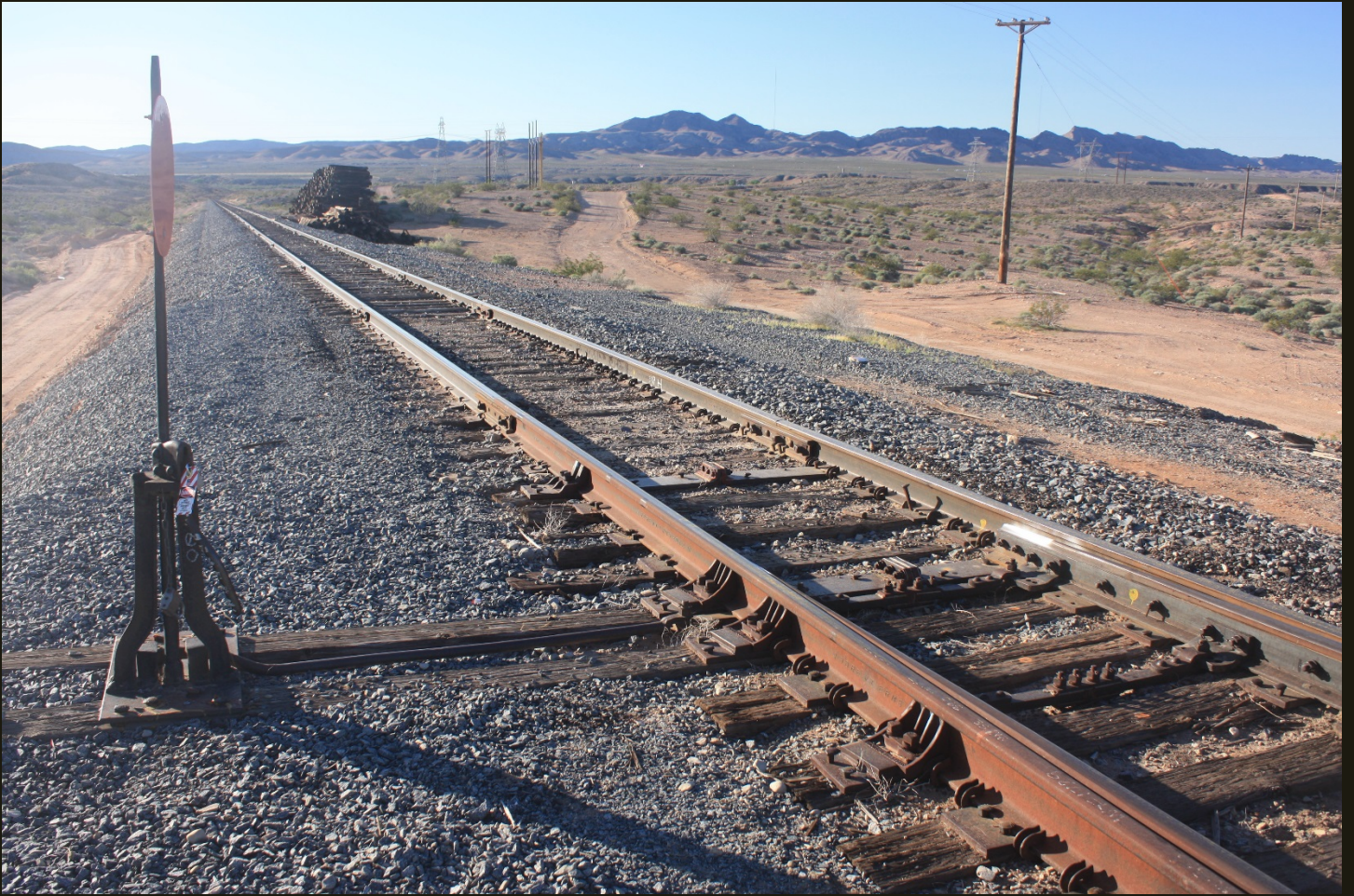
Southeastward view of the switch at the tip of the wye, where the SPLA&SL St. Thomas Branch (1912) heads southeast toward Overton and St. Thomas. The pile of ties testifies to recent tie replacement work.
