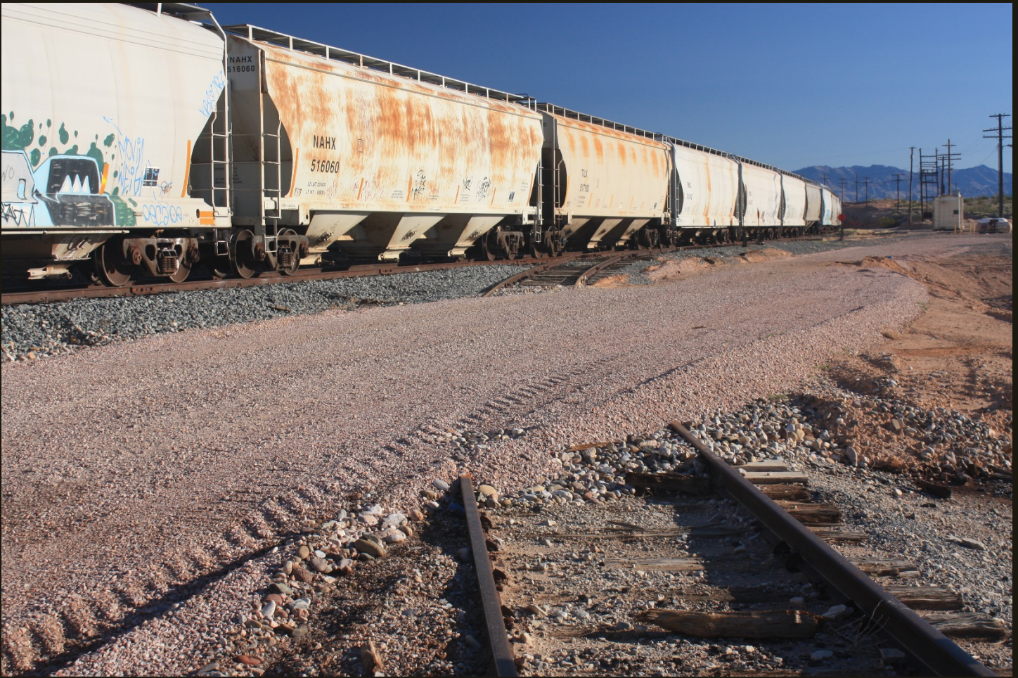
Northward view of the east branch of the wye for the SPLA&SL St. Thomas Branch (1912) where it joins the siding for the SPLA&SL (1905). I think the gravel covering of the track is temporary.
