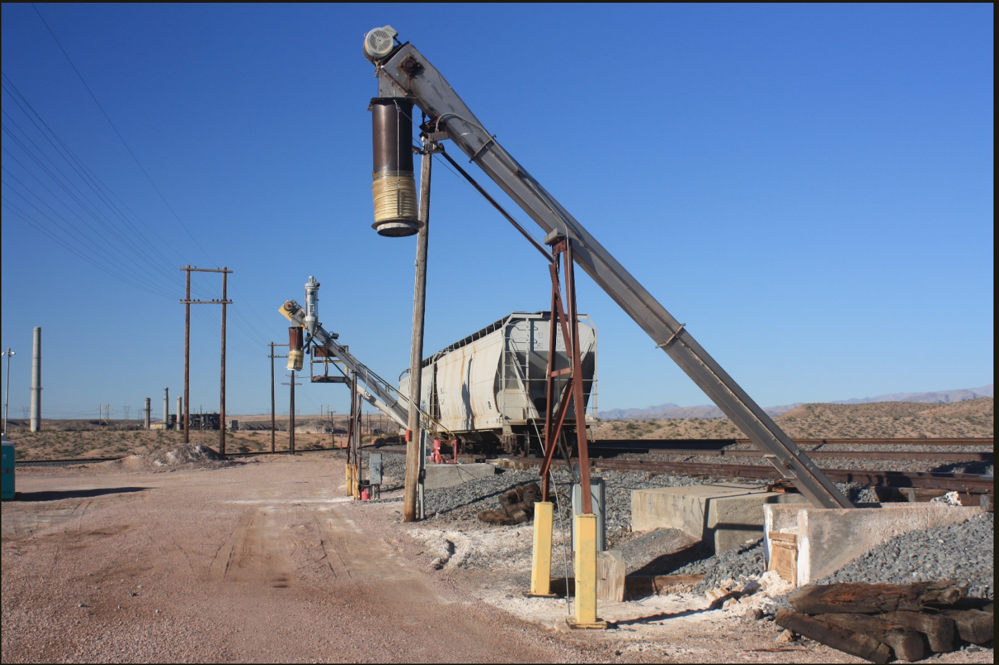
Southwestward view of the SPLA&SL (1905), 600 feet northeast of the previous location. The west branch of the wye for the SPLA&SL St. Thomas Branch (1912) is at the far end of the dirt area on the left. The same line of cars is on the siding, with rail-to-truck loading facilities.
