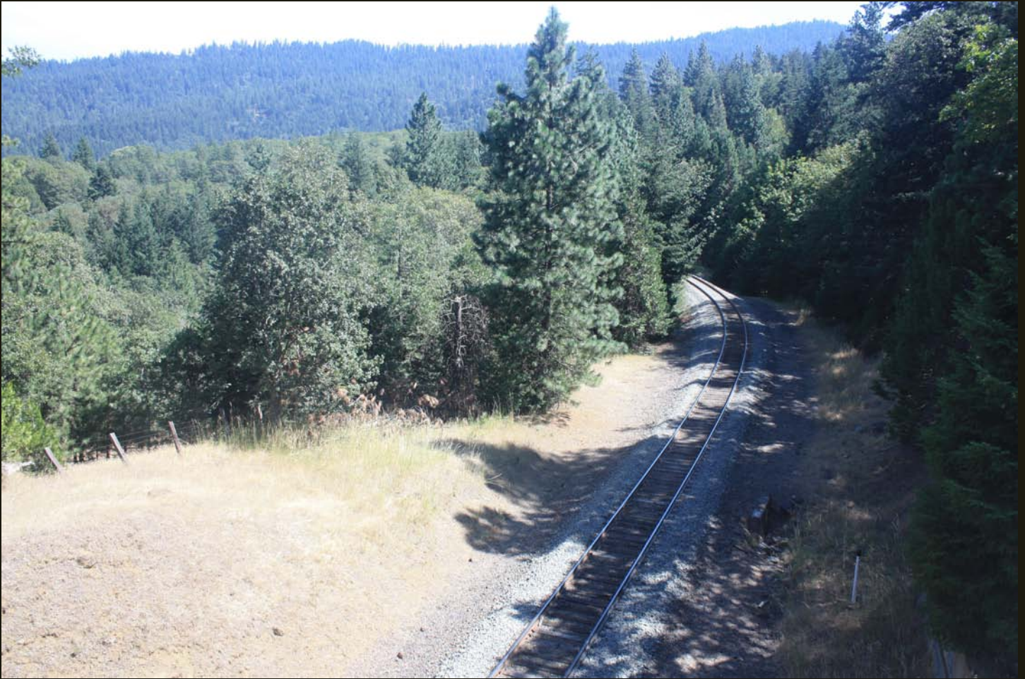
Northward view of the C&O (now CORP) line, 4 rail miles north of the pass and one switchback closer to the pass than the previous location.
