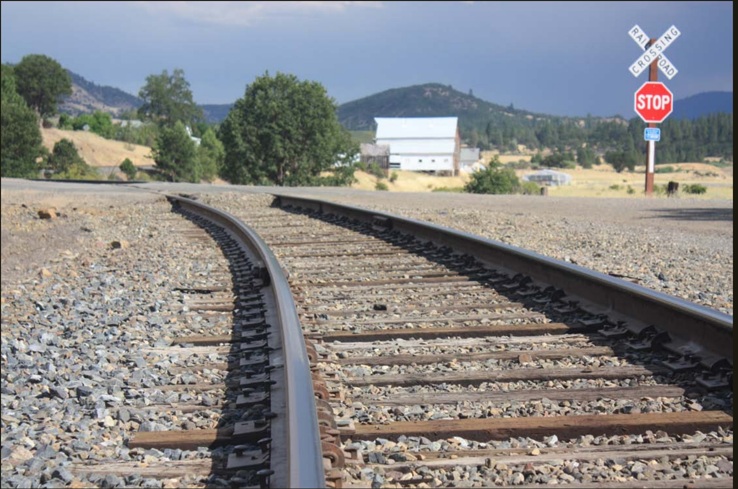
Southward view of the C&O (now CORP) 5 miles south of the summit tunnel, as the crow flies, at the California state line.
