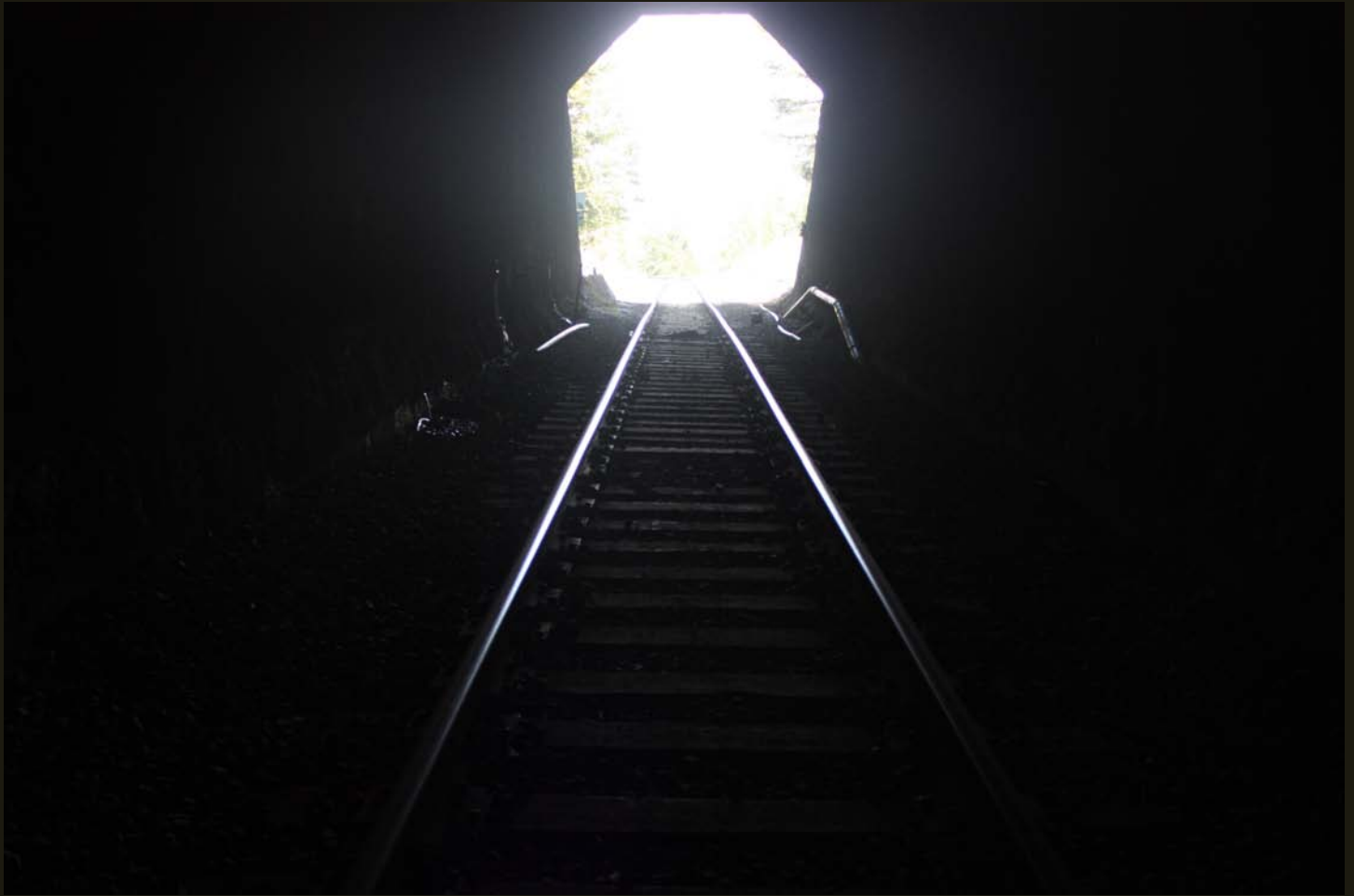
North entrance to the Siskiyou Summit Tunnel. The Pacific Crest National Scenic Trail passes overhead.
