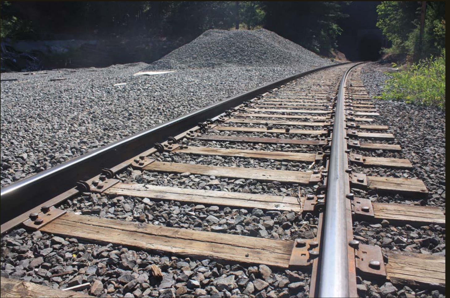
North entrance to the Siskiyou Summit Tunnel.
