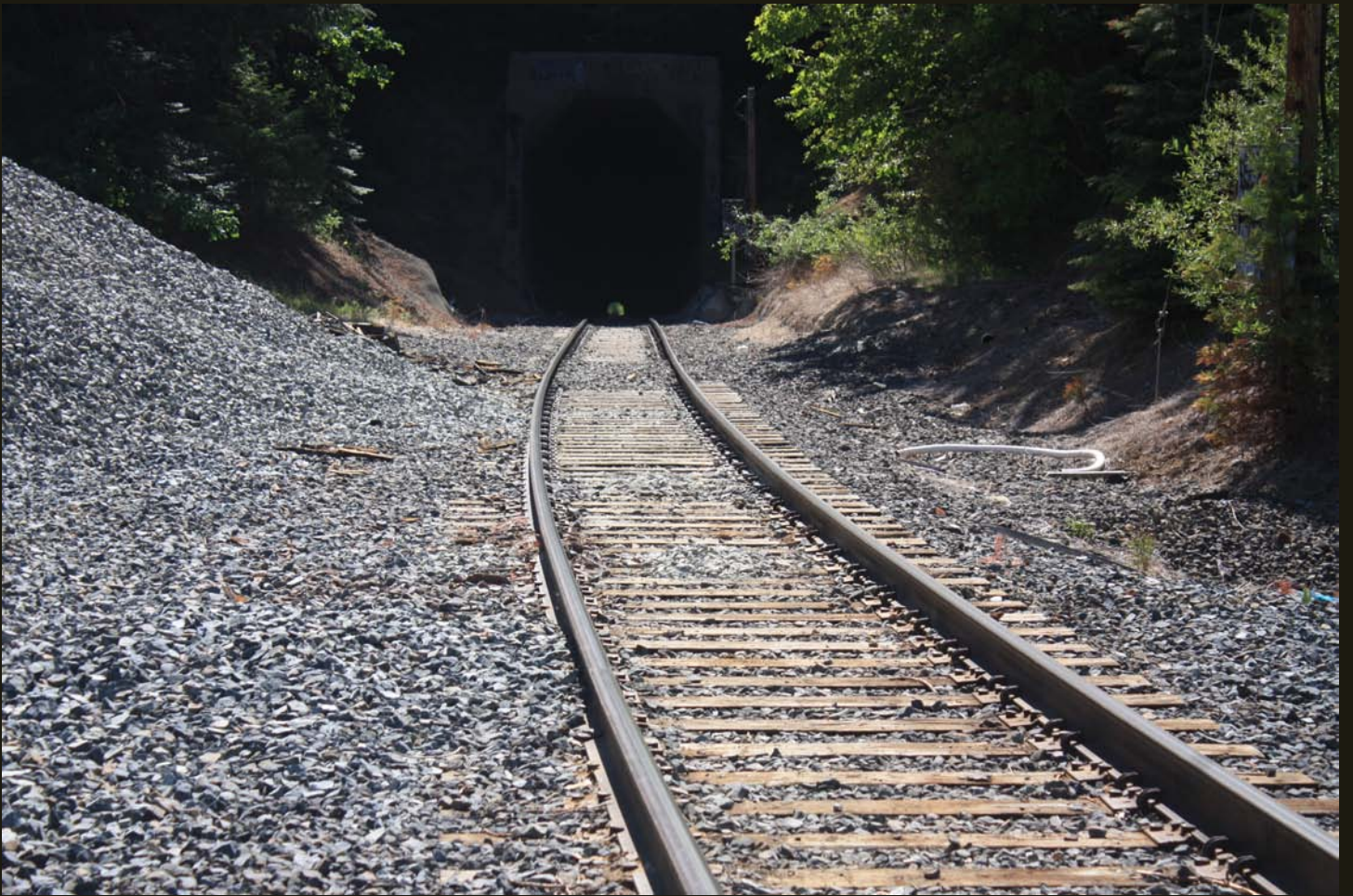
North entrance to the Siskiyou Summit Tunnel.
