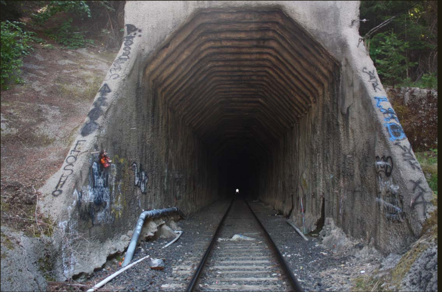
North entrance to the Siskiyou Summit Tunnel.
