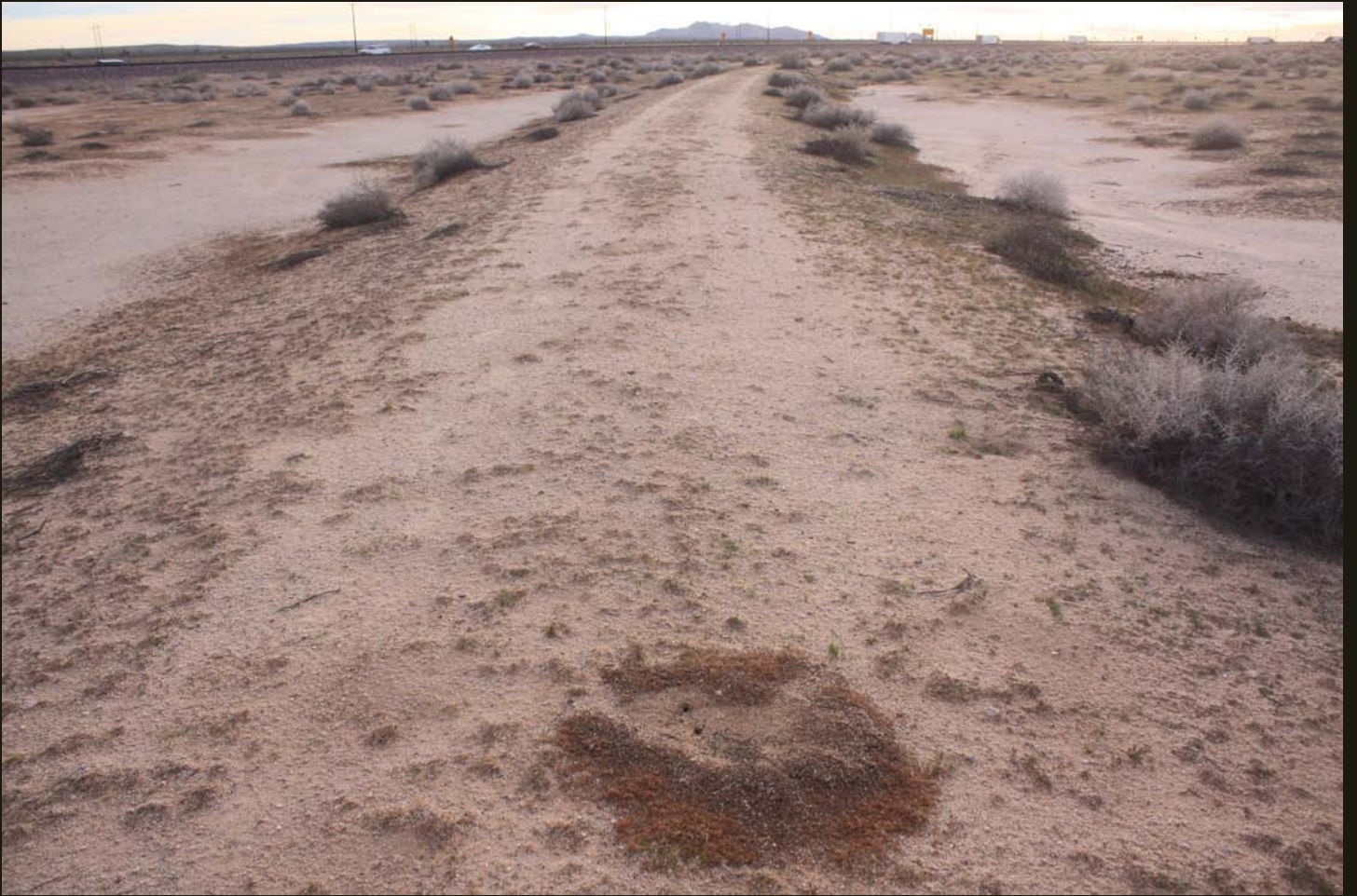
Southwestward view of the west branch of the RR junction wye. The BNSF main line is in the distance with cars on California Highway 58 just beyond.
