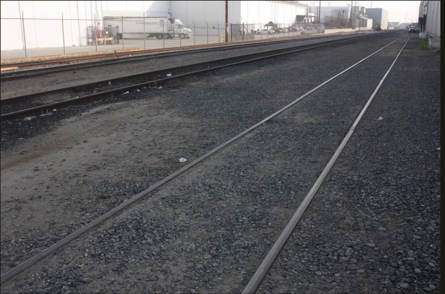
LAJ active line and sidings.
