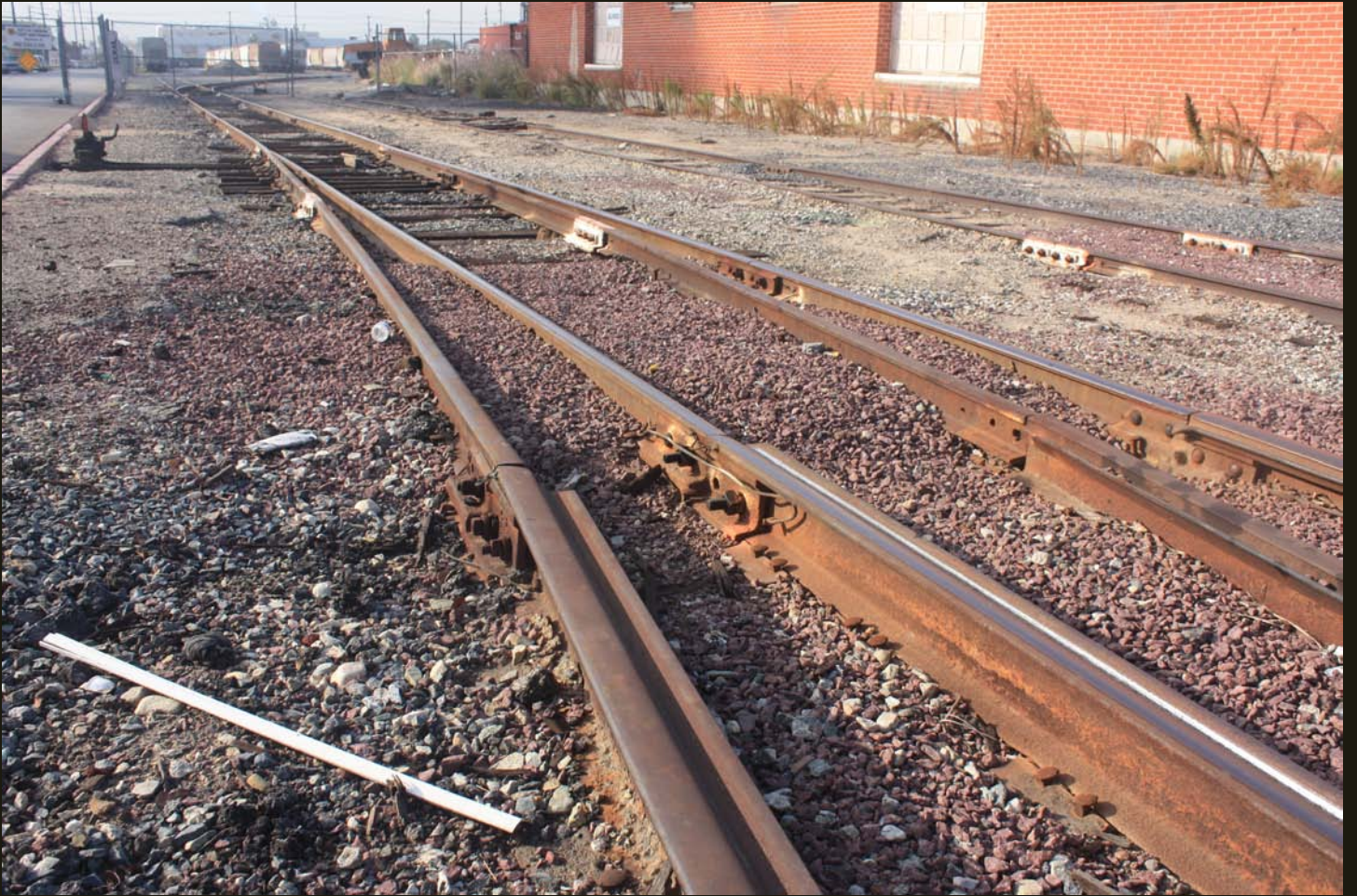
LAJ spur to an industrial classification yard.
