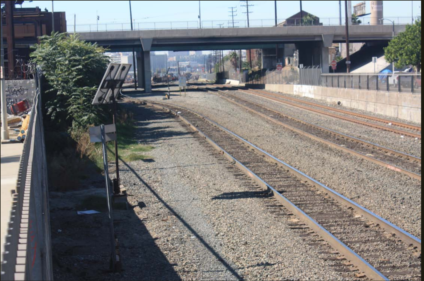
Westward view of the east end of the SP/UP yard in east LA, 3/4 mile east of the SP bridge in the first photo. The nearest, bolted track is the only remaining siding and continues about one mile east from here, after which the double, welded track of the SP/UP main line continues to points east.
