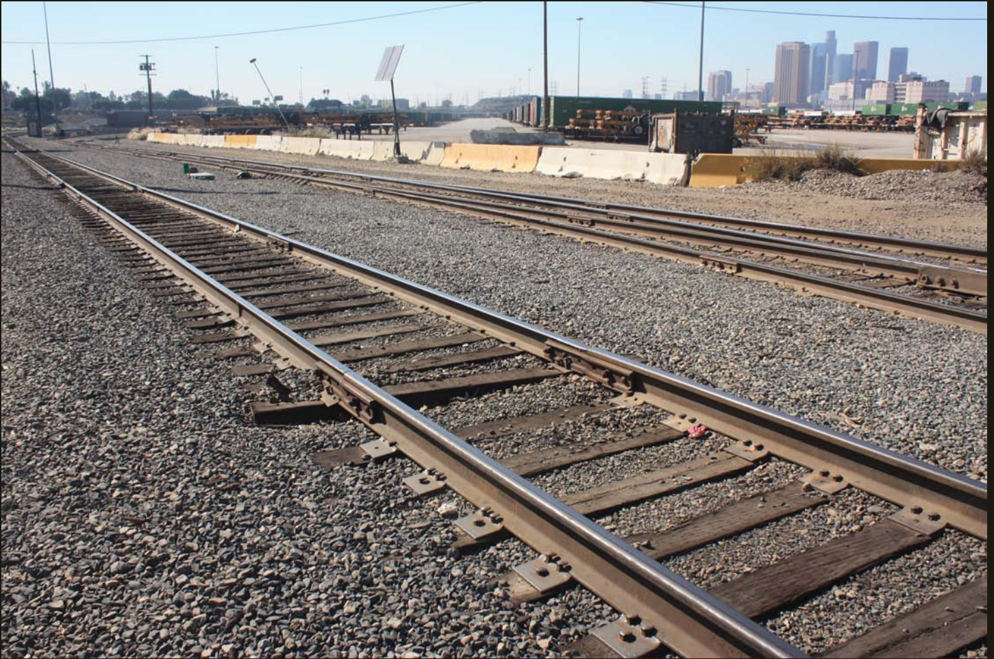
Westward view of downtown LA, a half mile east of the SP bridge in the first photo. This bolted track is not the SP main line, but rather is part of a huge yard used to assemble container trains.
