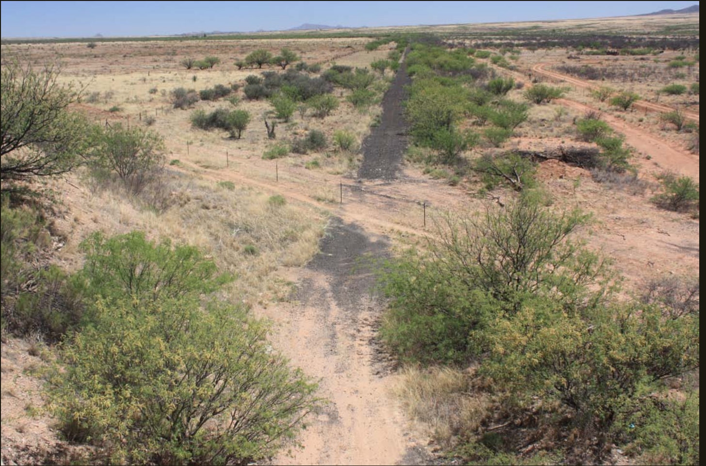
Southeastward view of the EP&SW (1904) taken from the same location as previous. Note the typical EP&SW black slag ballast.
