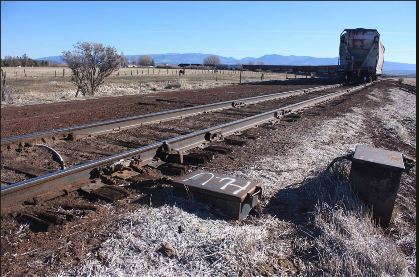
The train curves left (north) onto the former N-C-O grade. Note that the second leg of the wye curves right (south) where the tracks are still in place for about 10 miles south of Alturas. Track oiling equipment is in the foreground.
