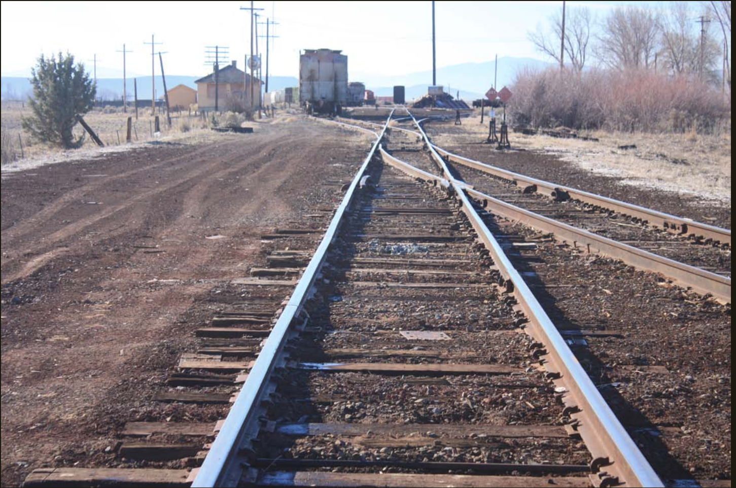
This southward view of the former N-C-O grade shows the switch with southbound leg of the wye in the foreground and some sidings for rolling stock storage.
