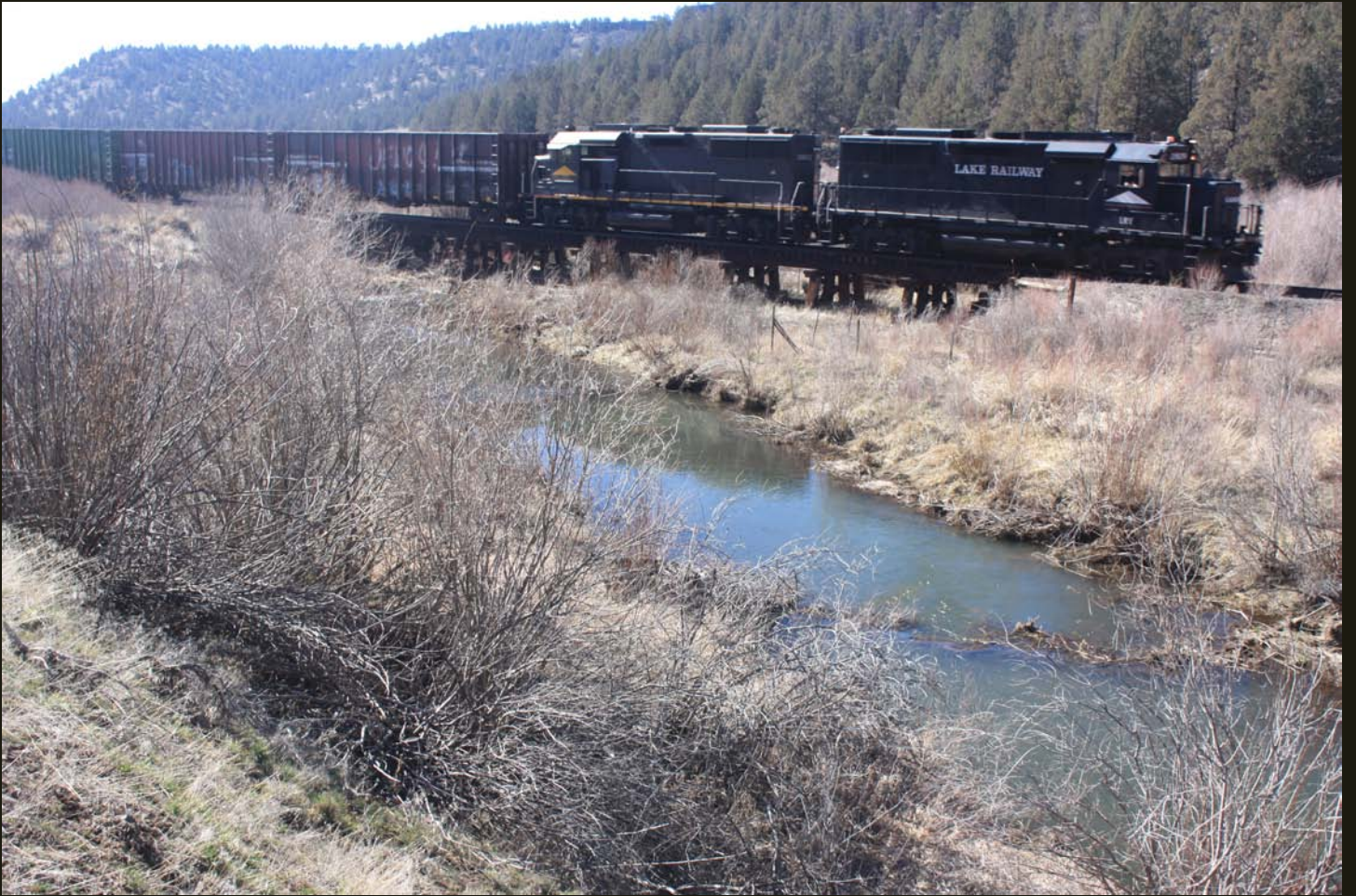
The N-C-O grade follows the North Fork of the Pit River, a tributary of the Sacramento River, to the divide between the Pacific Slope and Great Basin.
