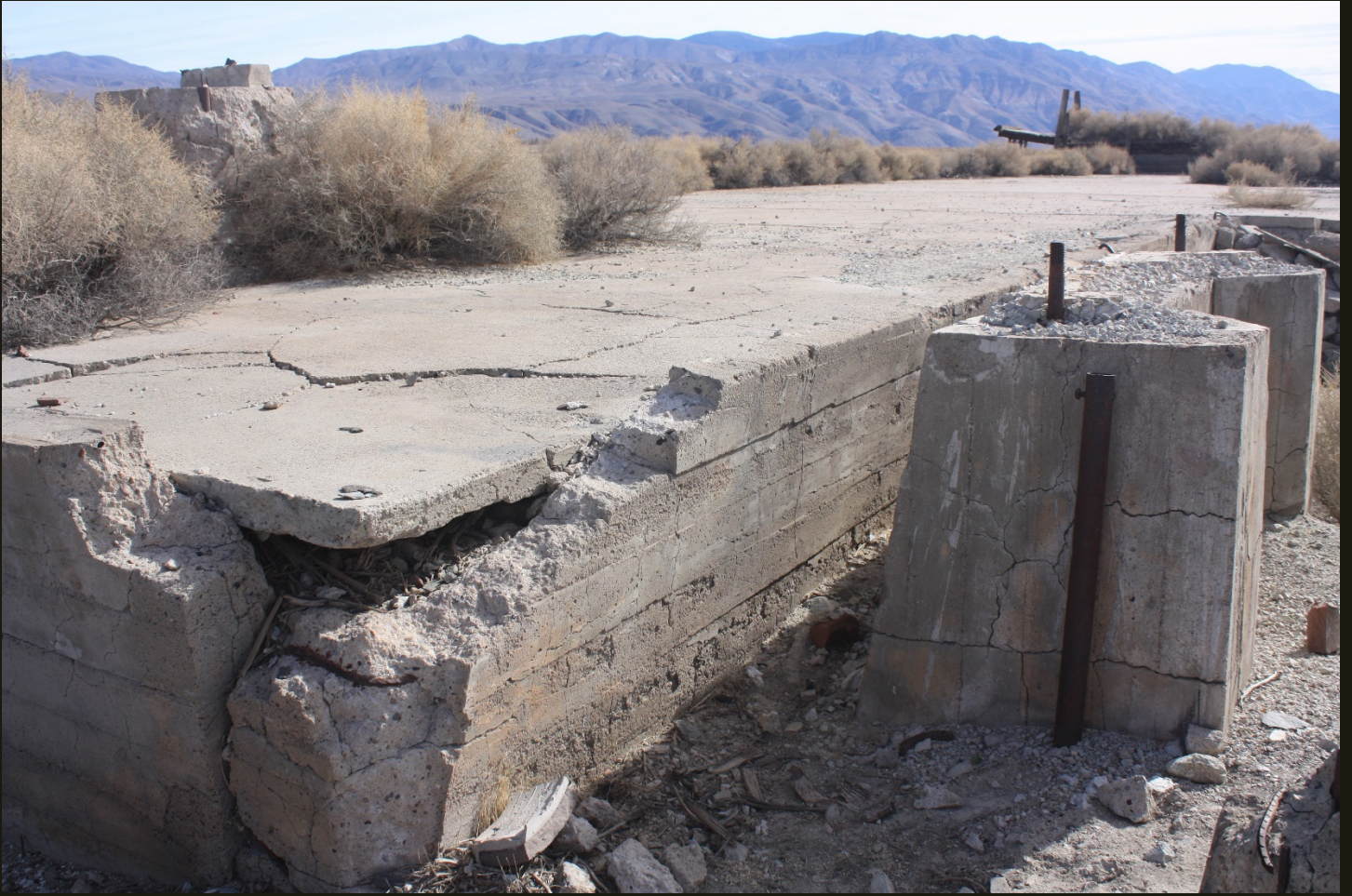
Southeastward view of the foundation of the depot building at Zurich, California. The same post-1960 loading ramp is visible right of center.
