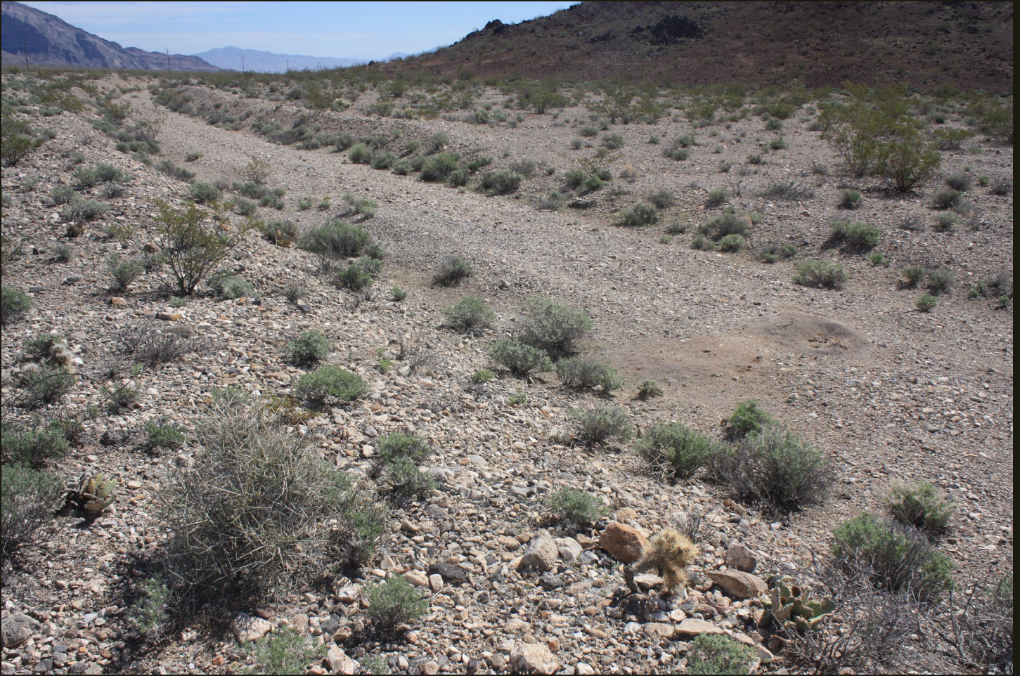
Eastward view of the grade of the DV (1914n), 300 feet east of the previous location. The fill grade in the previous photo has turned to a cut grade to negotiate the mountain promontory visible to the right.
