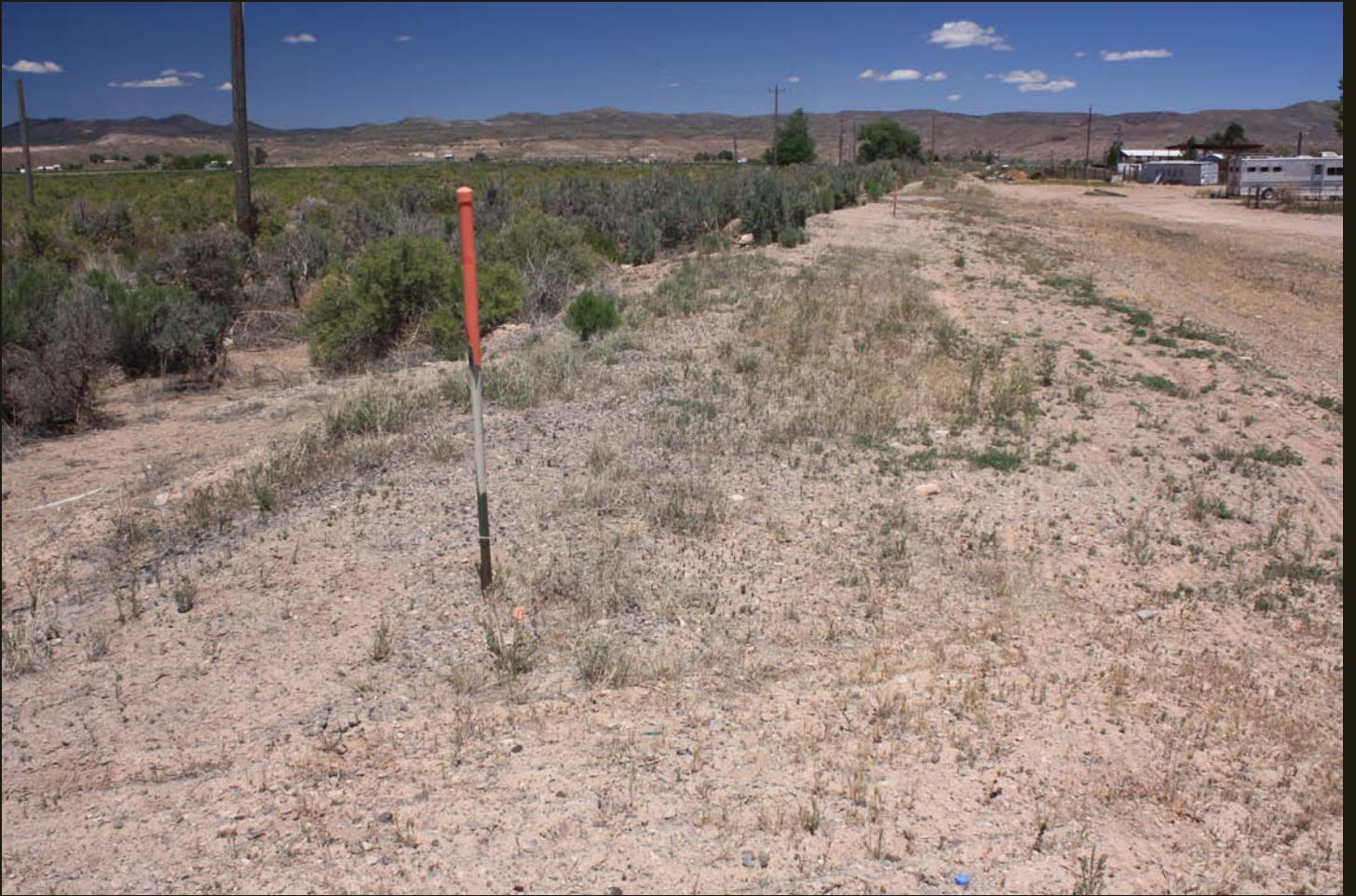
Northward view of the C&P (1907), a slight fill grade, a half mile south of previous location.
