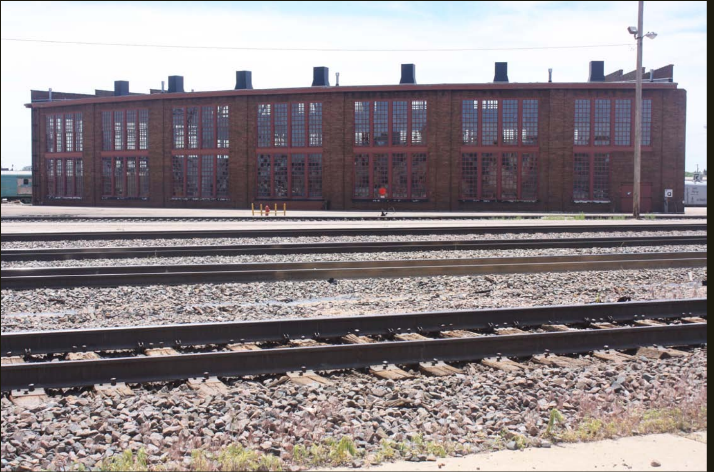
An old industrial building across the tracks from the Cheyenne Depot.
