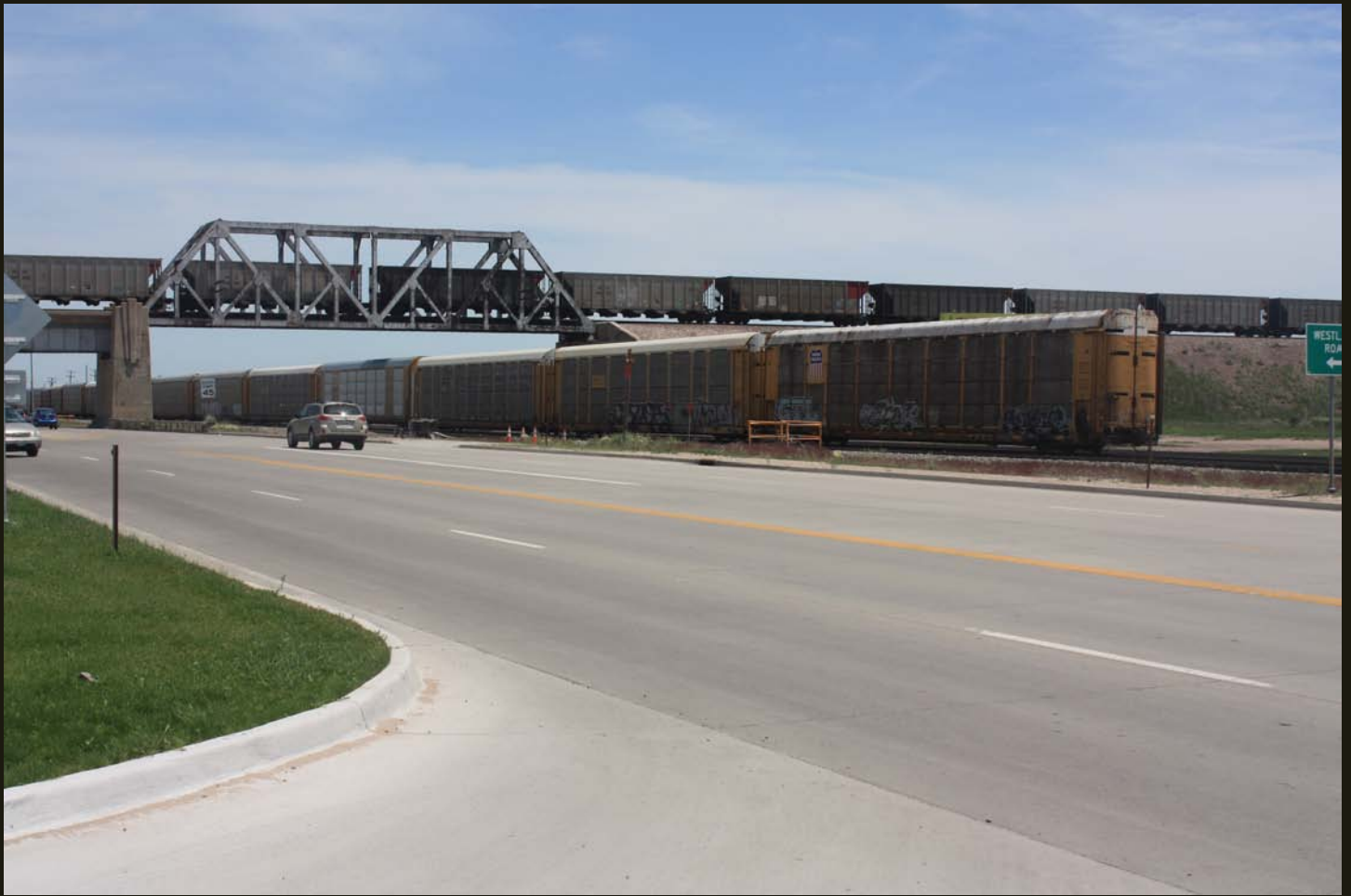
About a mile west of downtown Cheyenne, a grade separation overpass carries a coal train on BNSF's CC-C&N route over the UP mainline. This is not the original crossing, and the C&N originally connected to the UP at a wye that became downtown Cheyenne (see above for photos and information).
