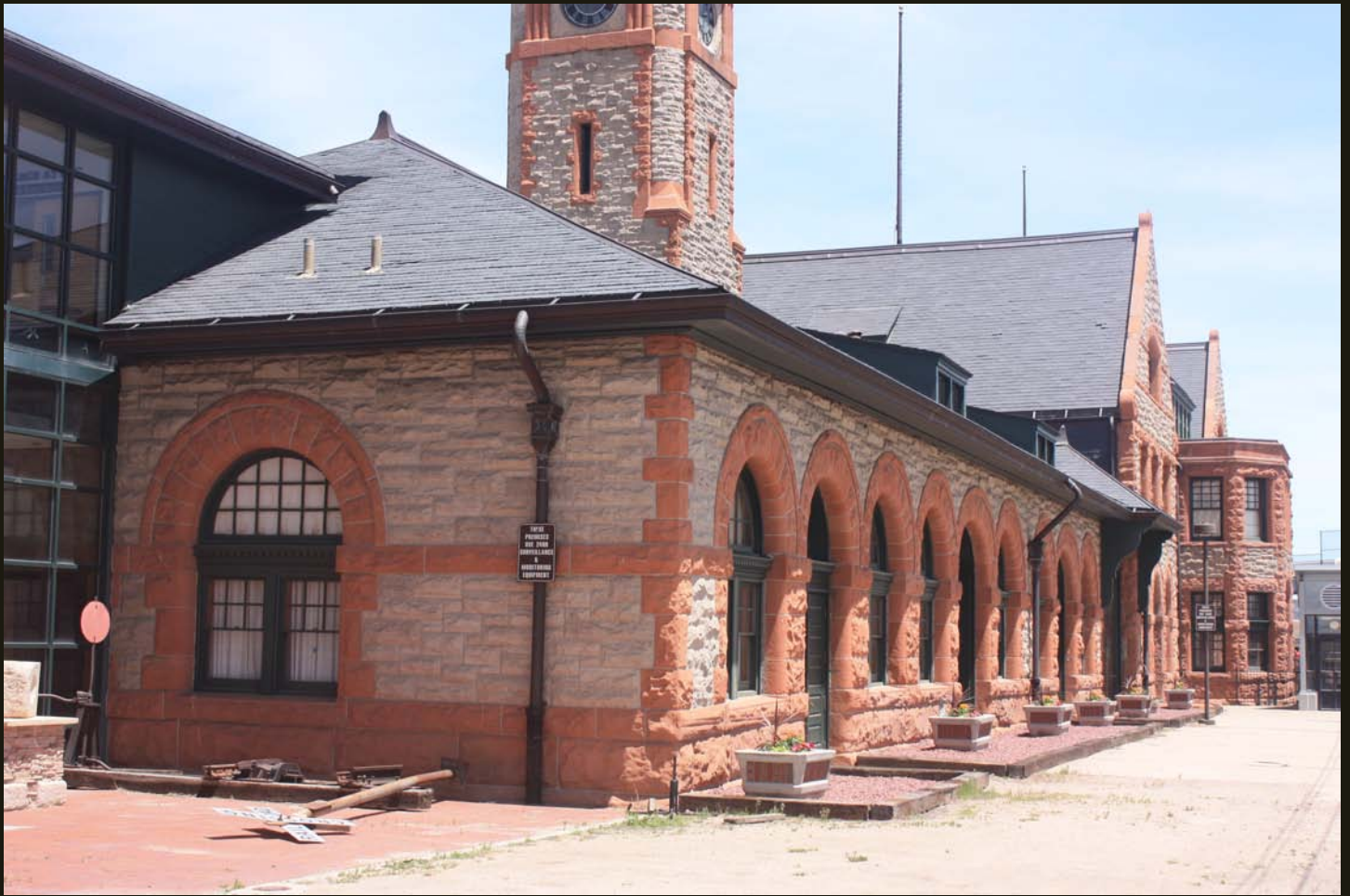
The UP's Cheyenne Depot, now the Wyoming Transportation Museum, was built in 1886-1887 on the UP mainline and is self-proclaimed to be the most beautiful rail station in North America. The station is built from blocks of sandstone quarried and transported from Ft. Collins, Colorado, and stands directly down the street from the Wyoming State Capitol. He depot received major renovations in 1922 to lengthen the building and a redecoration in 1929.
