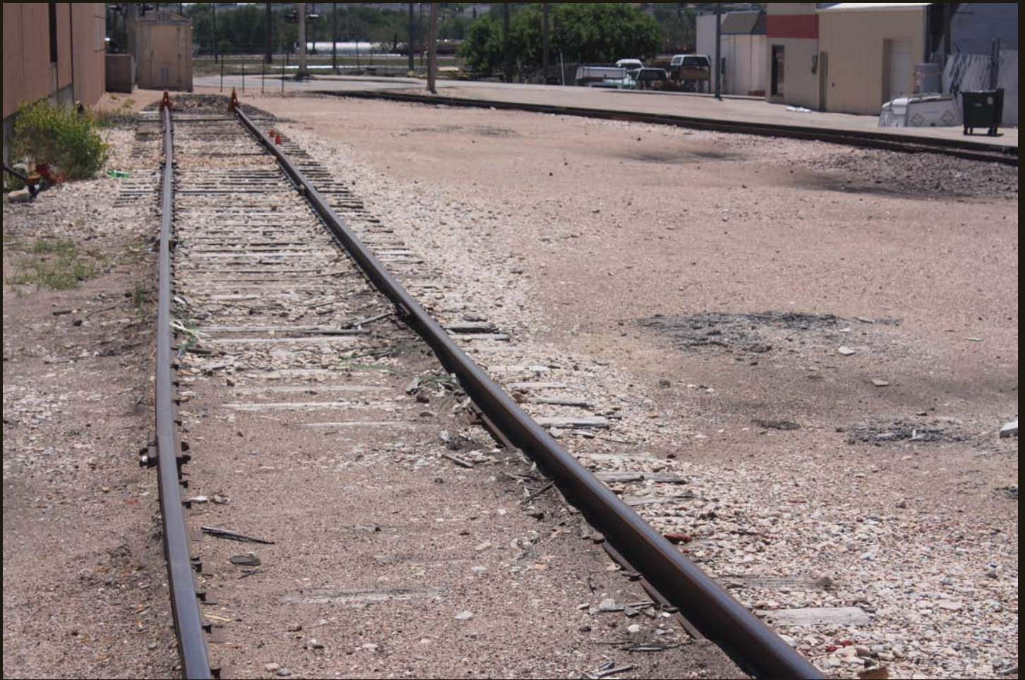
This southward view of the 1886 C&N wye in downtown Cheyenne shows the left branch (to the eastbound UP mainline) has been cut off, but the right branch (to the westbound UP mainline) continues to the UP mainline, visible in the distance.
