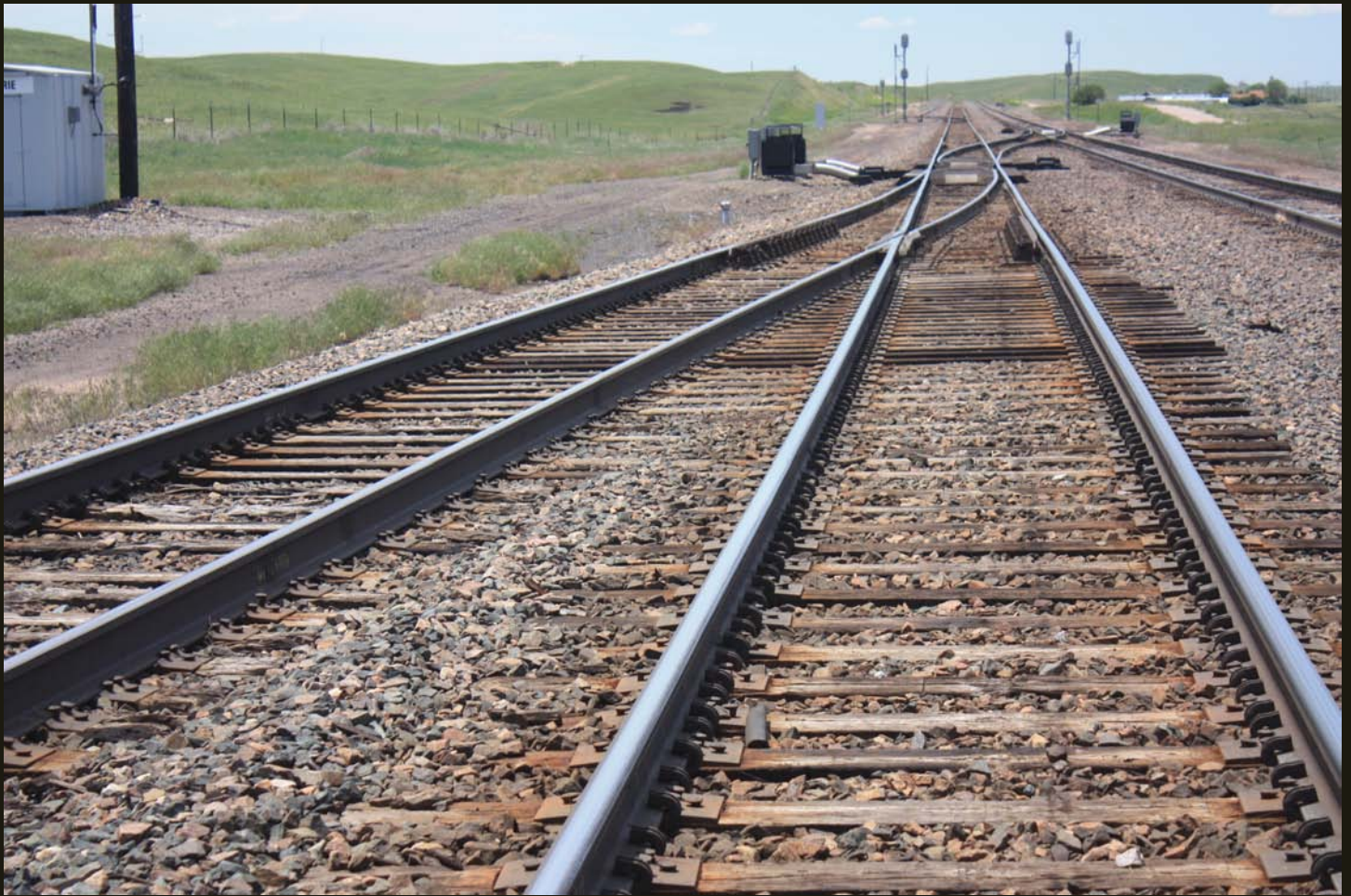
Westward view from same location as above; the single-track cutoff converges with the UP double track, which continues up Sherman Grade to Evans Pass, the most significant grade on the UP mainline. The TV series "Hell On Wheels" spent an entire season in Cheyenne as Sherman Grade slowed UP construction in 1868.
