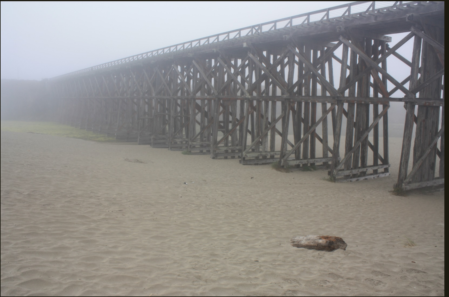
Southwestward view of the Pudding Creek Trestle.
