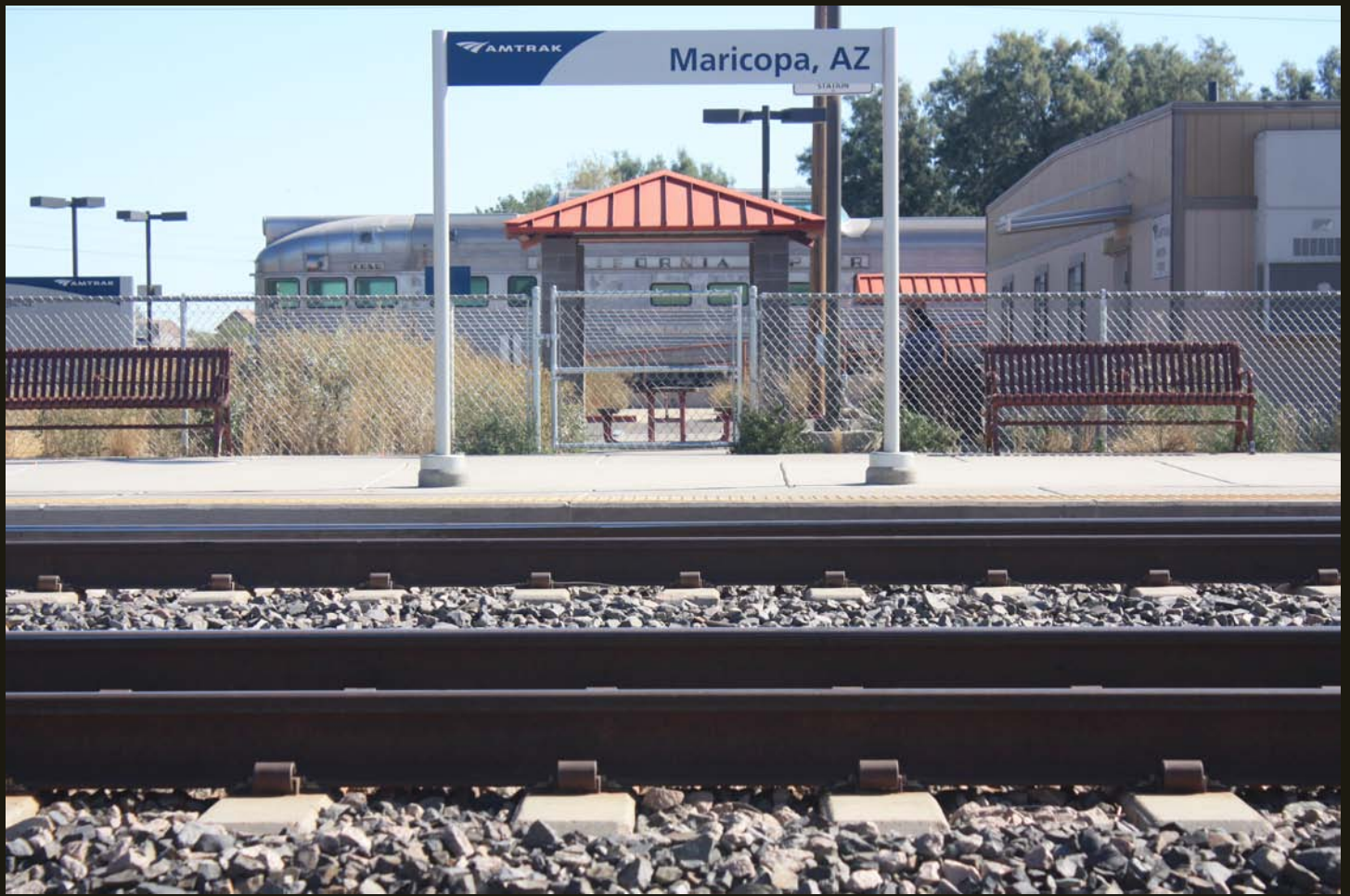
Closer view of the Maricopa Amtrak station. Note the vintage rolling stock in the distance (see below).
