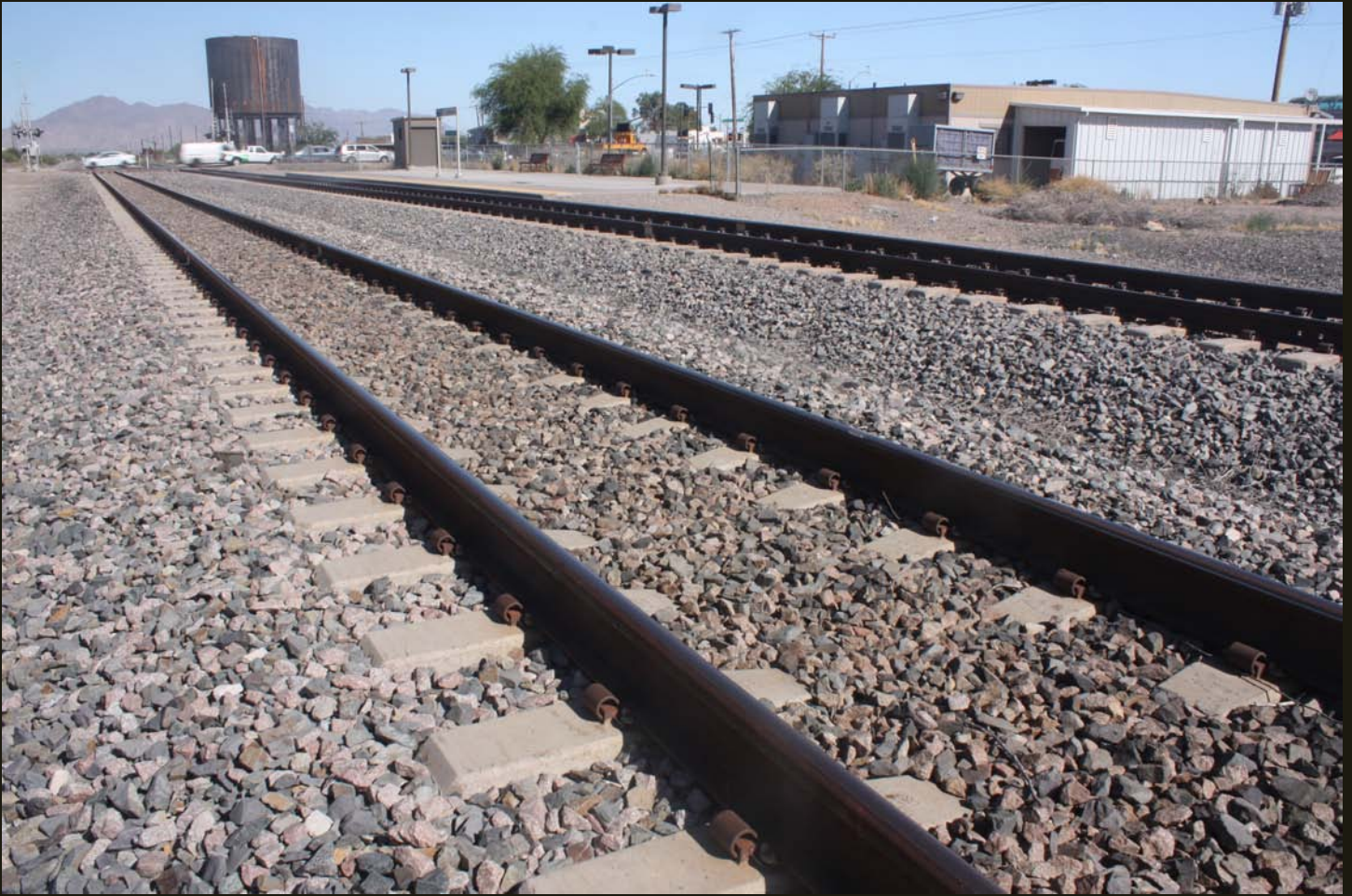
Westward view of the SP Sunset Route (1881), showing the same water tower as before. The autos are on Arizona Highway 347, which is built over the M&P alignment for much of the distance to Phoenix. The wye and loading facilities extended beyond the water tower, as seen in the previous photo, and to the location of the building on the right, which is now an Amtrak station.
