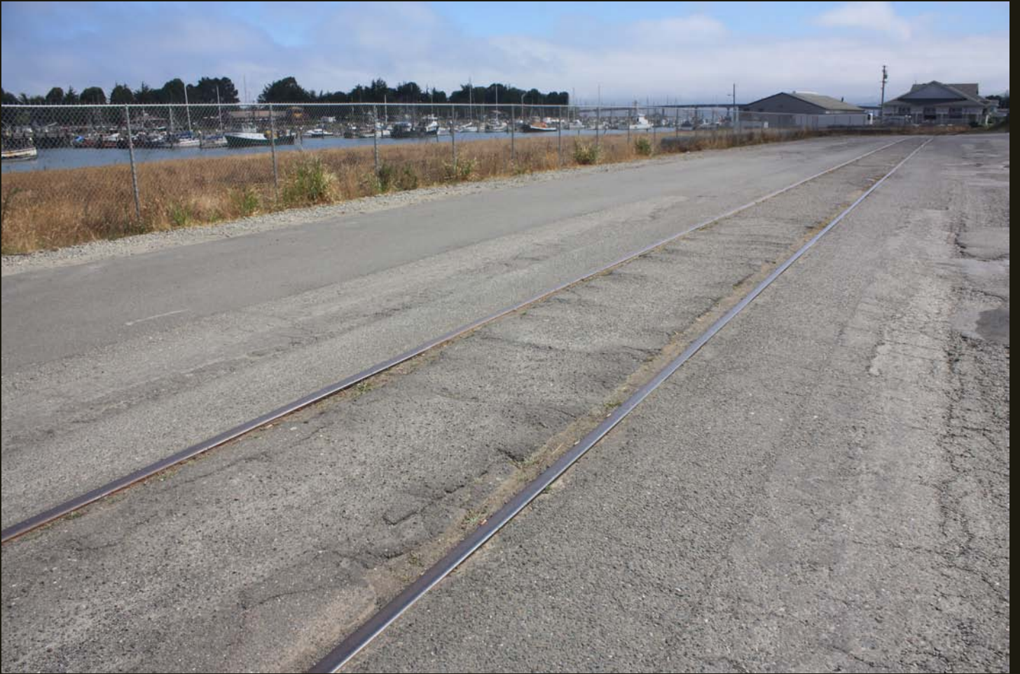
A few blocks northeast of the previous location, the C&N (1901)/NWP trackage runs along Eureka Harbor.
