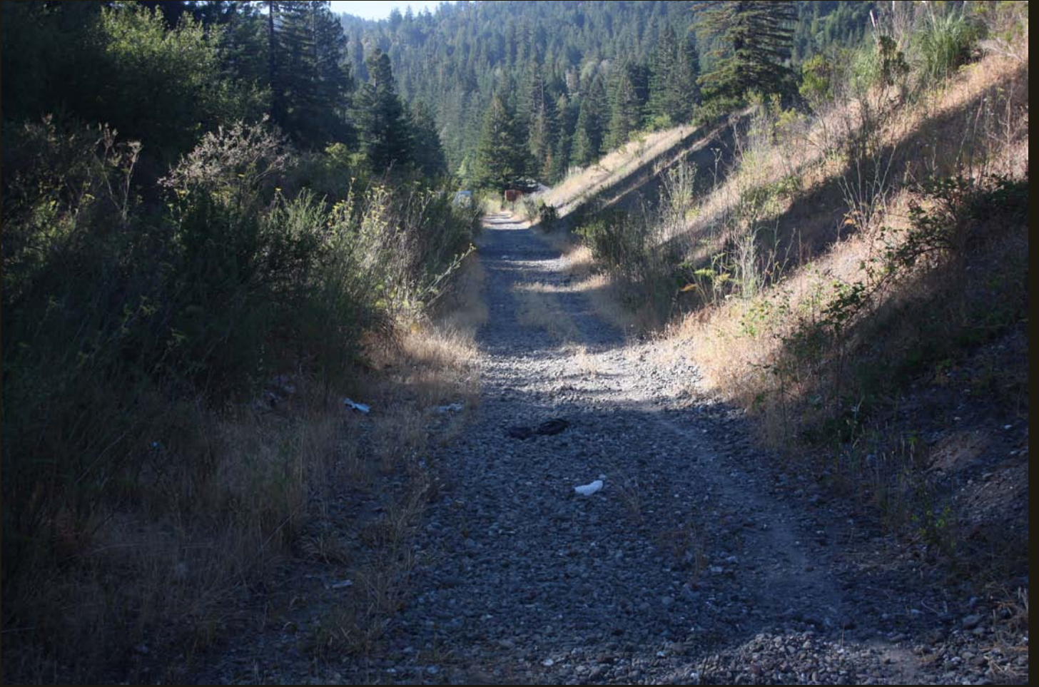
The SF&E/NWP tracks have been removed from this cut grade at South Fork.
