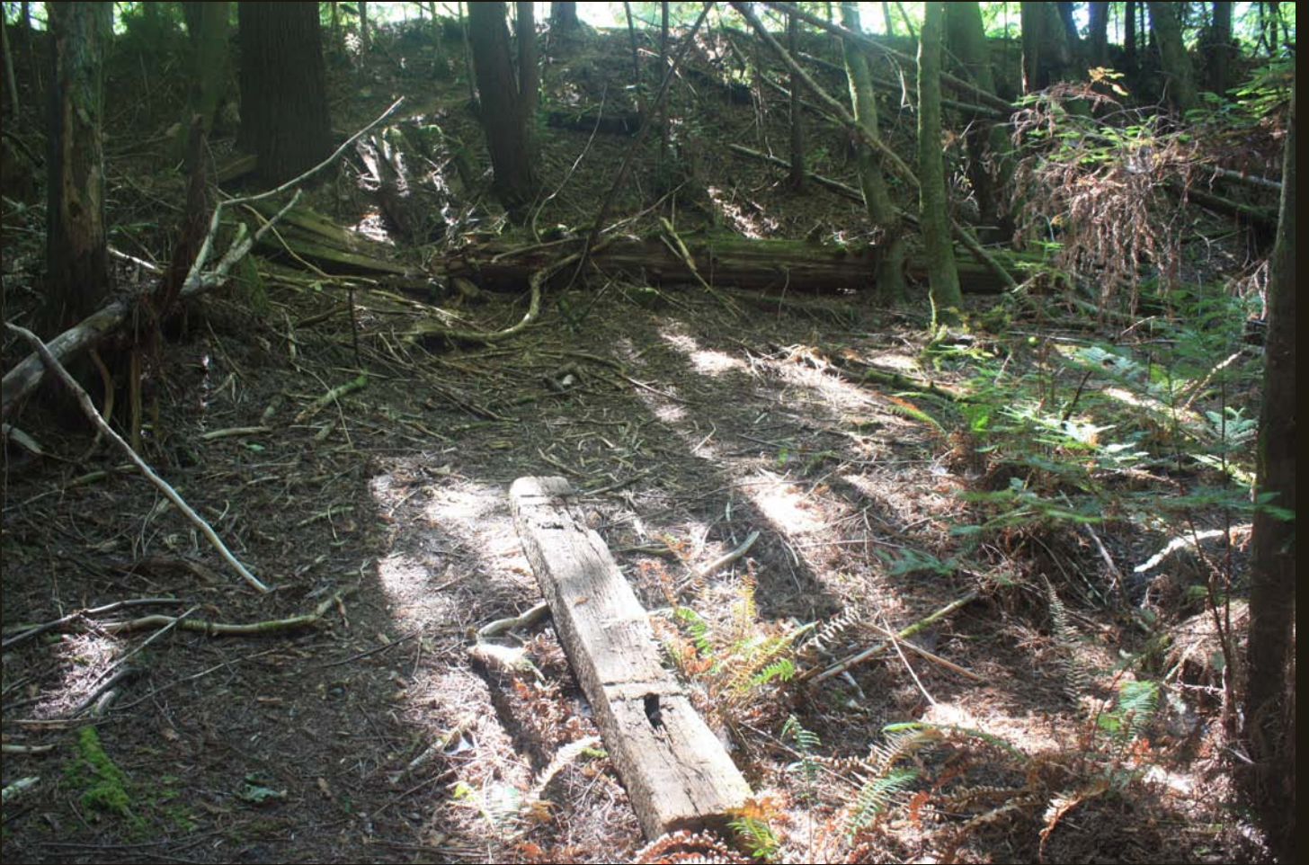
Same location as above, note the tie in the foreground and the fill grade behind it.
