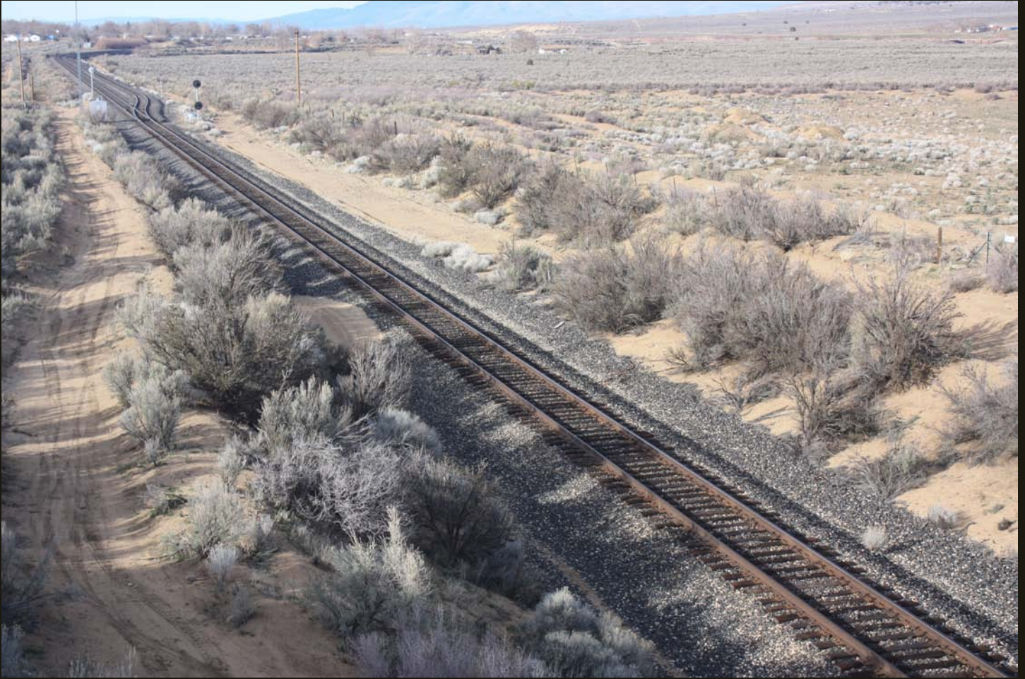
Northward view of the WP from the same location as the previous photo, with the town of Doyle in the distance. The N-C-O grade should be in the upper right part of the photograph heading into Doyle, but it's hard to tell.
