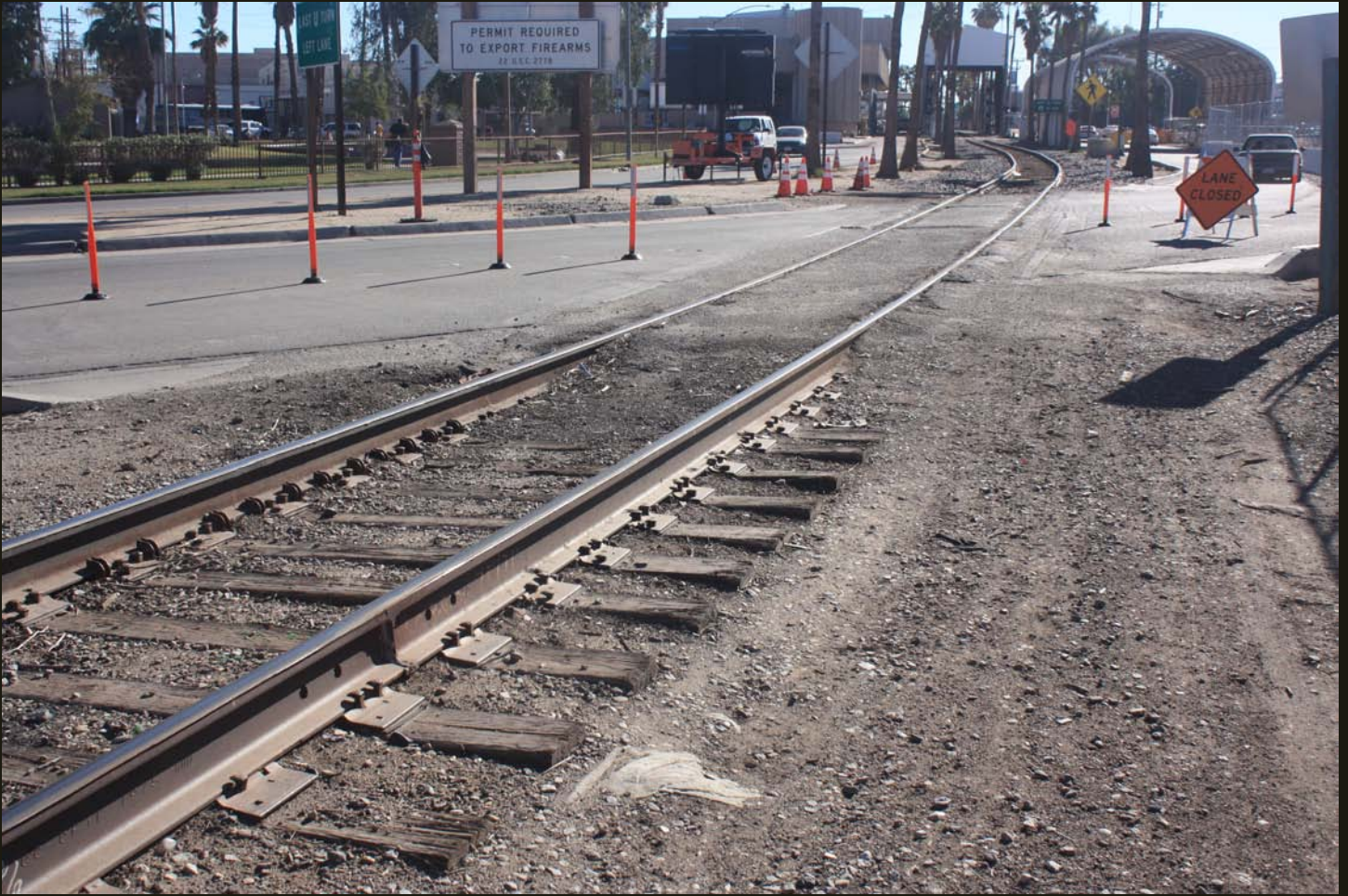
Southward view of the SP Inter-Cal (1904) at Calexico, 400 feet north of the Mexican border. The overhangs for autos and trains and the buildings beyond are border facilities.
