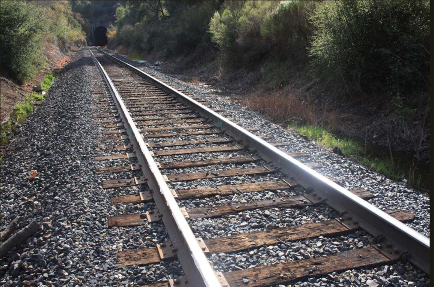
A closer southward view of the Cuesta Pass summit tunnel on the SP Coast Line (1894). Note the groundwater draining from the tunnel, which penetrates the water table.
