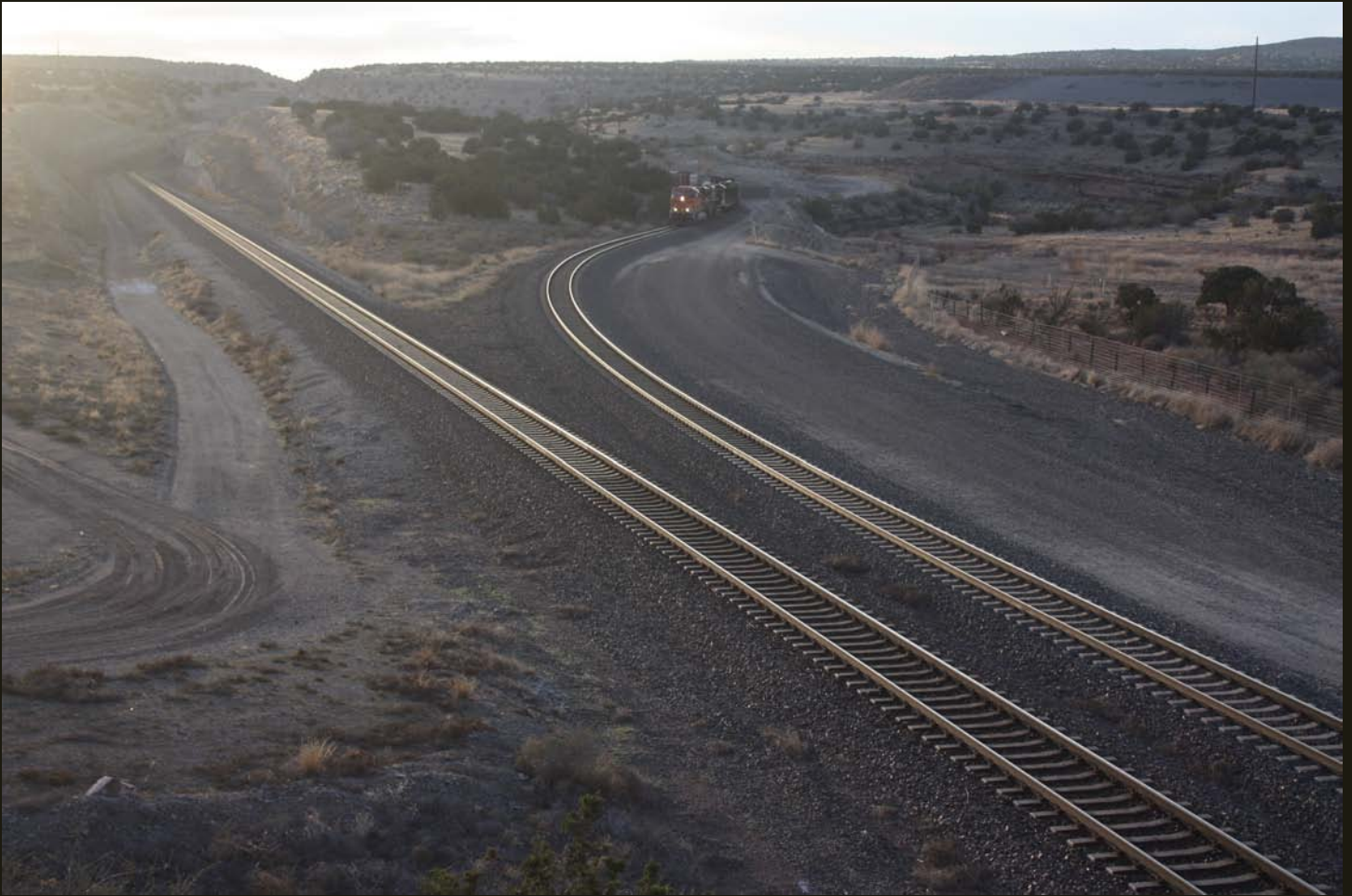
About 5 miles east of the previous photo, a BNSF container train climbs out of the Rio Grande Rift Valley to a low point between the Manzano Mountains north of the ERNM line and the Los Pinos Mountains to the south. Note double track and all concrete ties. Once past these mountains, the line has clear sailing across the Great Plains.
