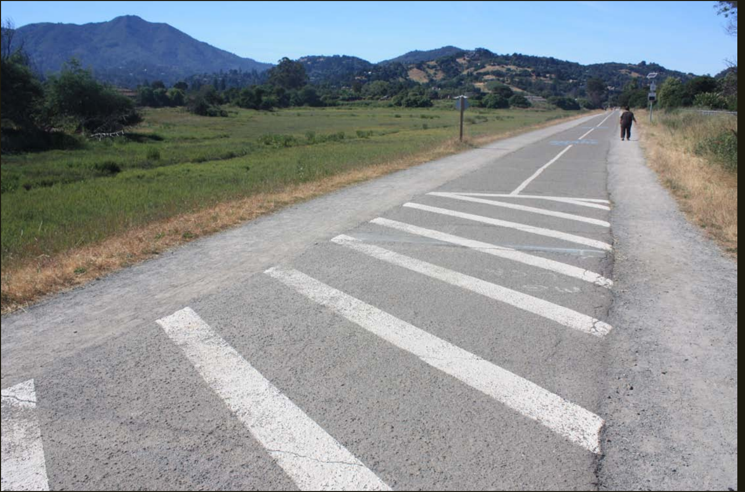
Northwestward view of the abandoned NPC/NS/NWP grade, same location as previous on tidal marshland.
