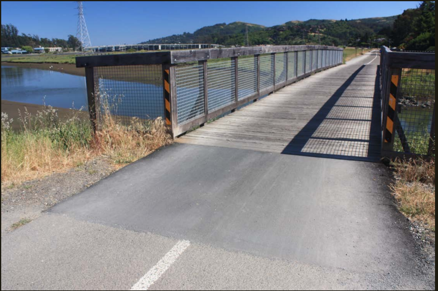
Southeastward view of the abandoned NPC/NS/NWP grade, 4 miles northwest of Sausalito. The grade is now a rail-to-trail, the Mill Valley-Sausalito Path. The bridge carries the grade over a tidal creek with an impressive name, Arroyo Corte Madera del Presidio, which drains to Pickleweed Inlet. The bridge in the left distance carries U.S. Highway 101 over Pickleweed Inlet.
