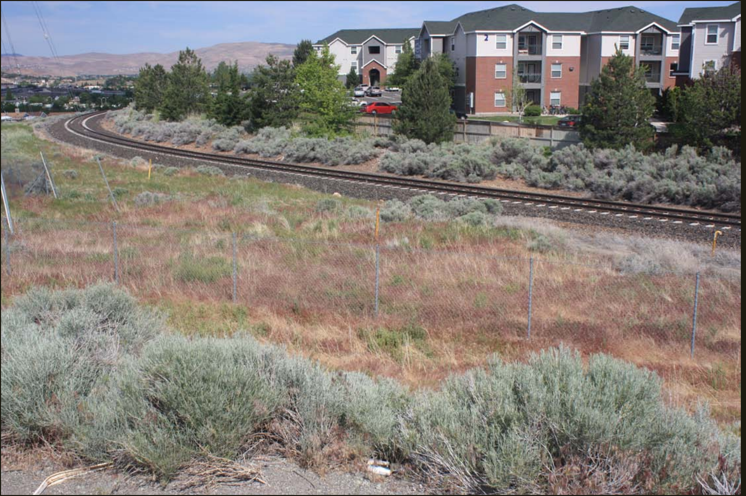
Southeastward view of the N&O (1882n), now the UP Reno Branch, 2.3 rail miles north of the previous location, as the alignment winds its way up out of the Truckee River valley. This curve is more than 180 degrees and winds almost completely around this apartment complex. The concrete ties extend only to the outskirts of Reno.
