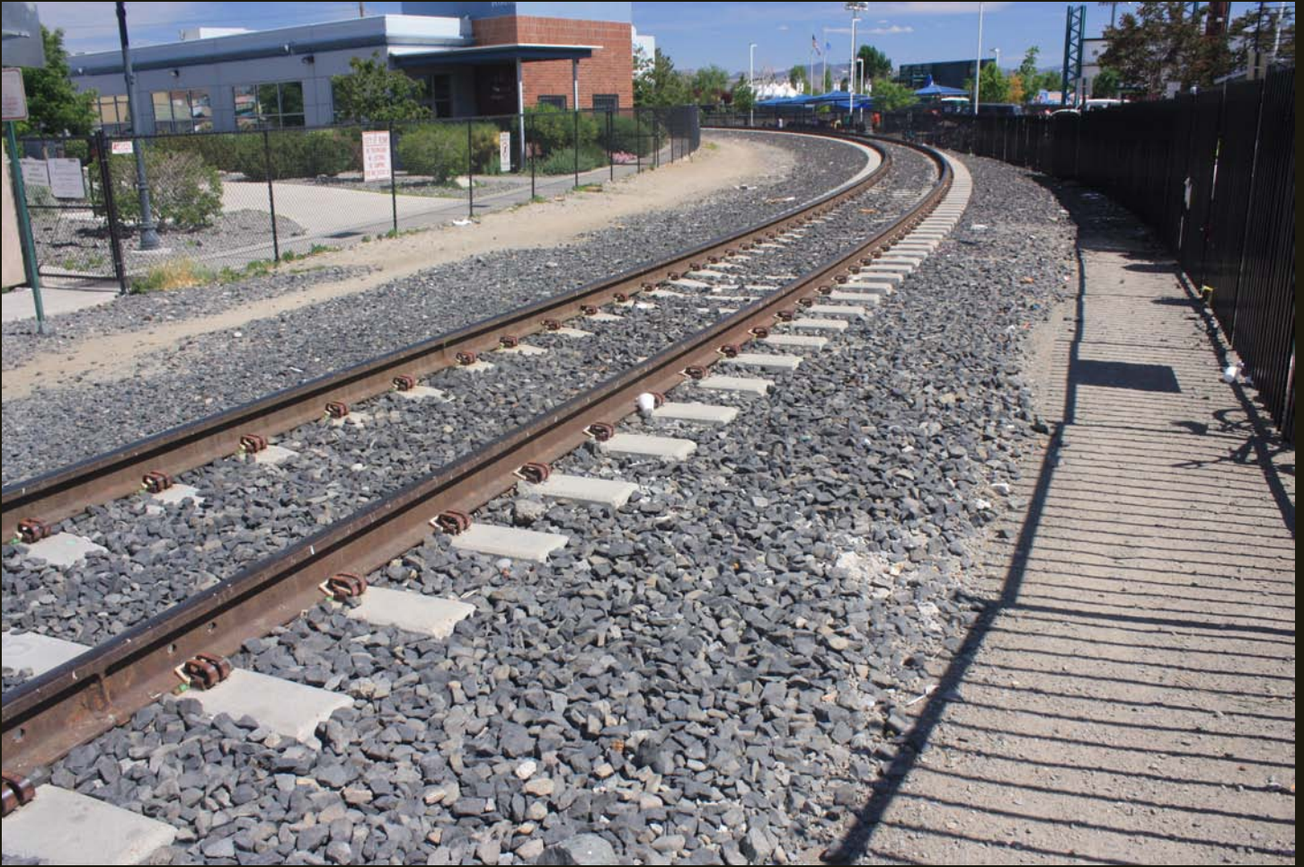
Southeastward view of the N&O (1882n), later the N&C, N-C-O, WP, and UP, here with concrete ties. This track continues to the 2,700-foot siding; the CP is just beyond the blue umbrellas.
