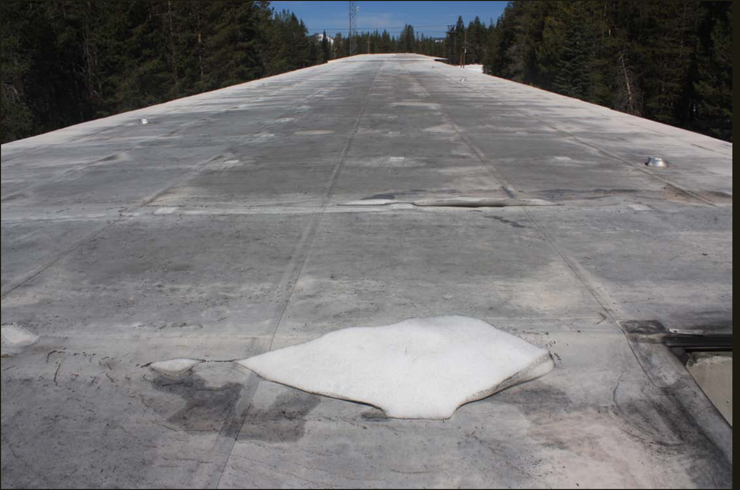
Another westward view of the west entrance snowshed.
