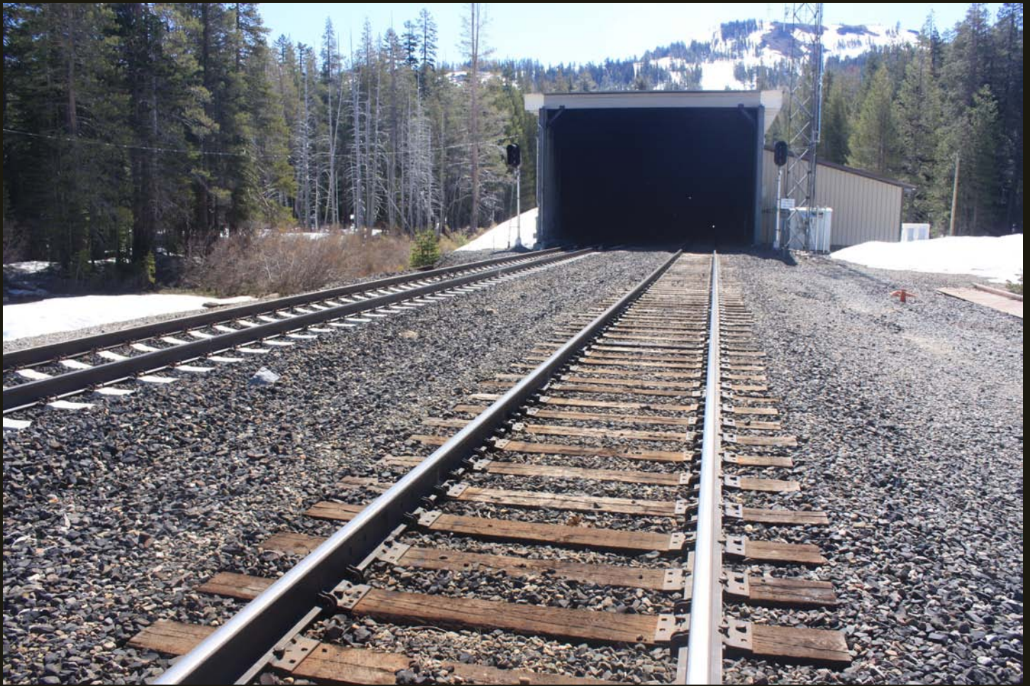
Eastward view of the west entrance of the SP's 1925 summit tunnel under Donner Pass, 1.1 miles east of Norden (previous location). The west entrance of the 2-mile-long tunnel has a 700-foot snow shed that covers a switch that brings the double track down to one track before entering actual tunnel. On-line discussions indicate this is a bottleneck on the UP's primary transcontinental route and diverts traffic to the UP's Western Pacific (1909) Feather River Route.
