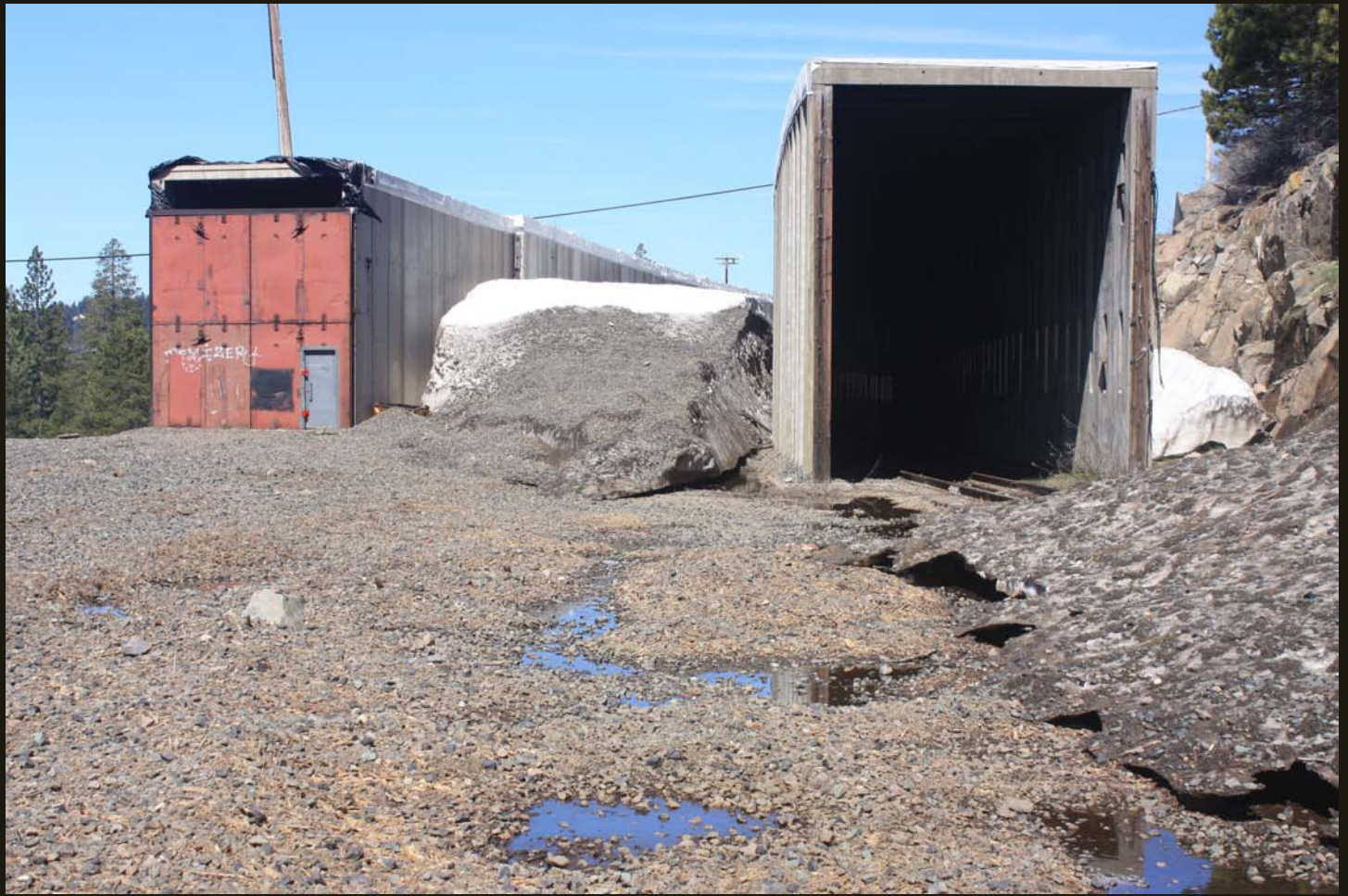
Westward view of the original (1925) east entrances for the Norden snowshed complex. The original CP alignment is on the right and still has tracks; this is the line to the original/higher summit tunnel. The shed entrance on the left (with the red door) is the 1925 second track to the lower summit tunnel. Both entrances had to have been built in 1925 to accommodate the two tracks, but it is unclear why their construction is so different.
