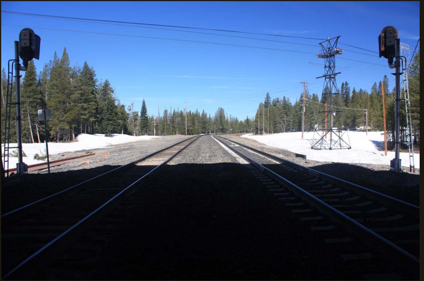
Westward view of the west entrance of the SP's 1925 tunnel/snowshed.
