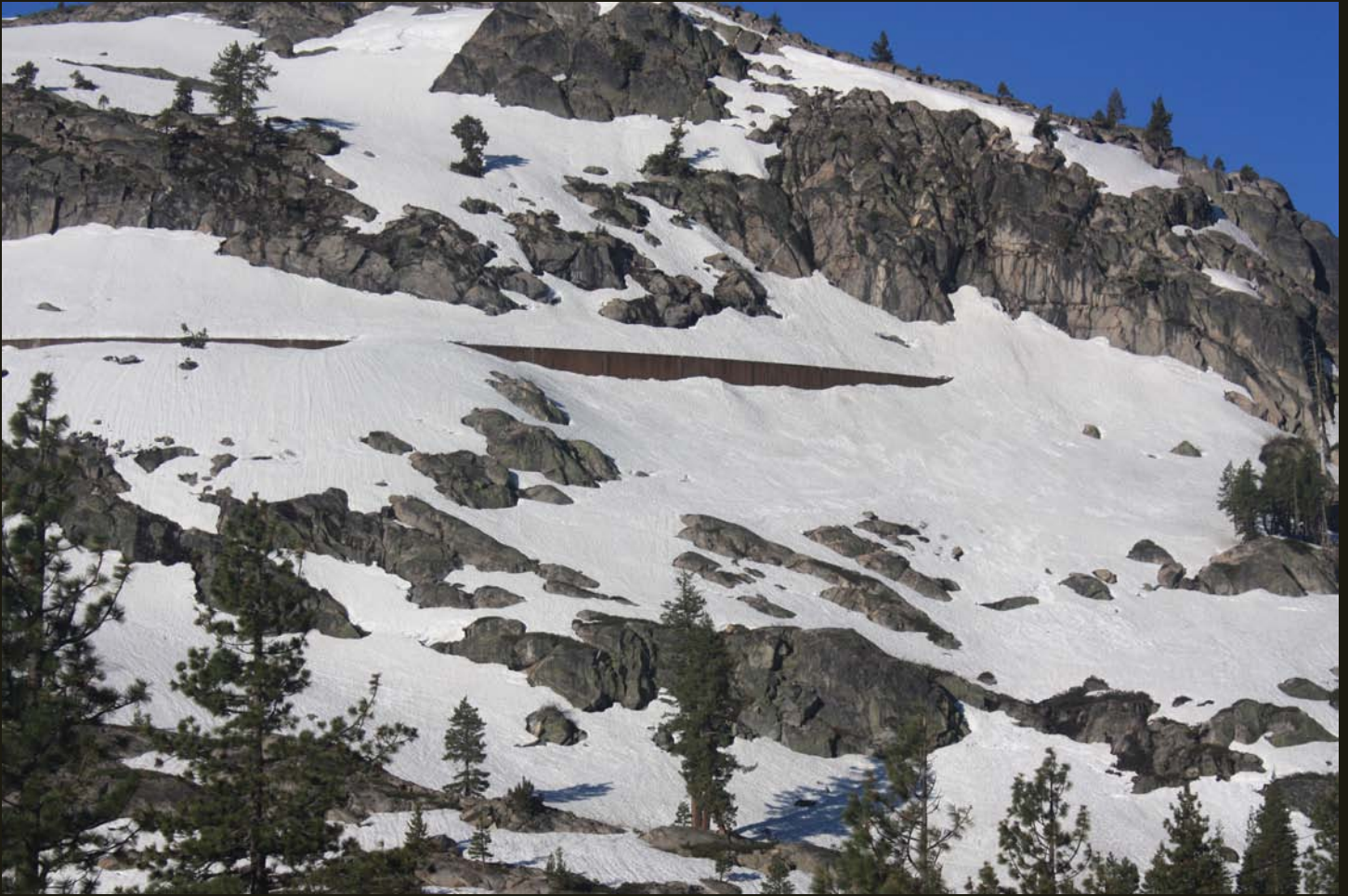
Southwestward view of the snowshed east of the China Wall. This shed continues 1.4 rail miles down the slope, interrupted only by four short tunnels. A lot of snow for late May.
