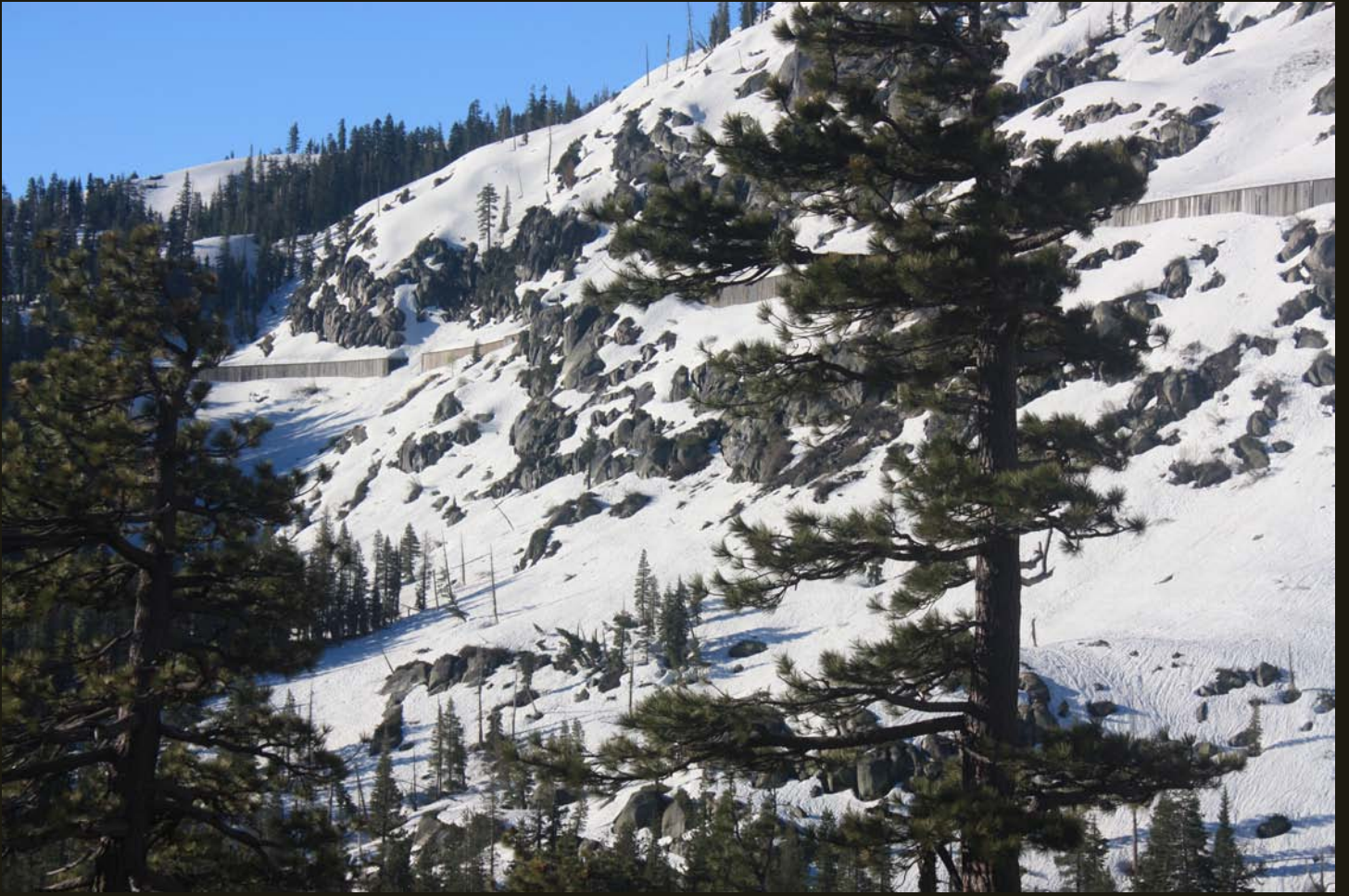
Southward view of the 1.4 mile snowshed east of the China Wall, just east of the previous location, where an avalanche has breached the shed.
