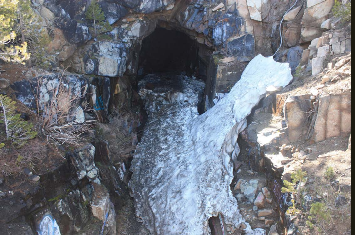
Eastward view of the west entrance of the original CP tunnel from Sugar Bowl Road.
