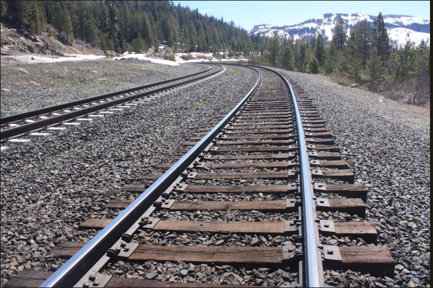
Eastward view of the active UP tracks on the 1925 alignment to the lower tunnel. The snow on the left slope accentuates the abandoned grade of the CP (1869) over Donner Pass via the original, higher-elevation tunnel.
