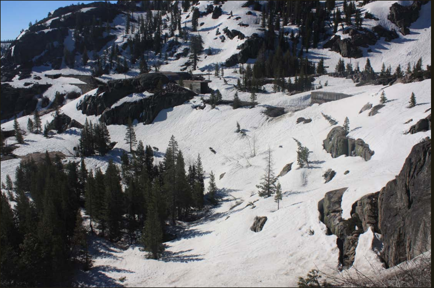
Southeastward view near the same location as previous. The snowshed on the right is the same one as in the previous photo, i.e. the east entrance of the original CP tunnel. Going left (east) from that shed is an open cut grade, then a shed built into a cut grade through a granite hump, then an open ledge grade with retaining walls – the “China Wall.”
