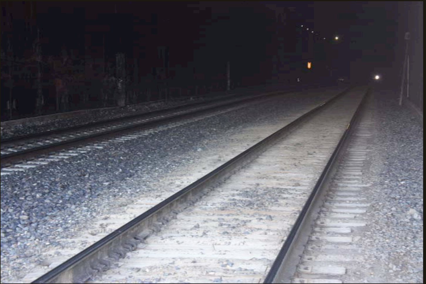
Eastward view of the trackage within the snowshed at the west entrance of the SP's 1925 summit tunnel. The switch that brings the double track down to one track is marked by converging track and the bright orange chevron on the switch. The light at the end of the tunnel is 2 miles away and is in the Great Basin.
