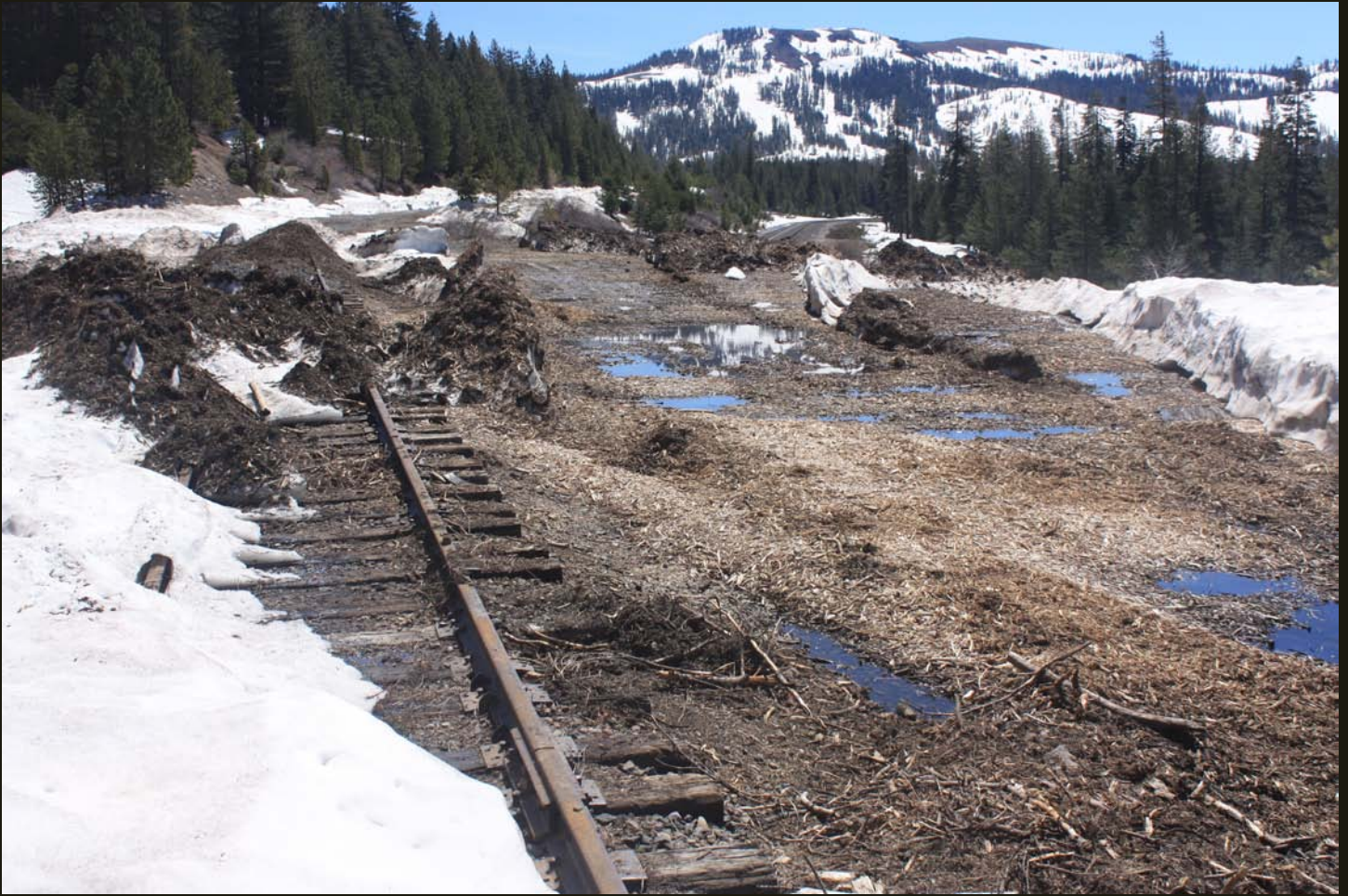
Eastward view of the original CP alignment, as it begins its climb to the upper tunnel and cuts a steeper grade than the active tracks (visible in the center distance) to the lower tunnel. The old track ends at a pile of dirt on the left.
