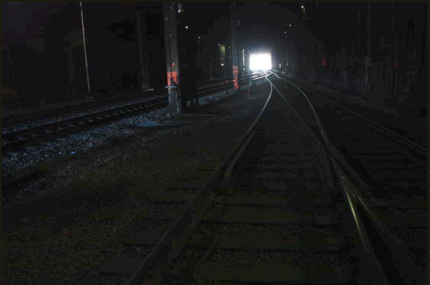
Westward view of the west shed entrance showing the inner workings of the Norden snowshed complex. There are four tracks here, from right to left: the original CP (1869) alignment; the 1925 second track alignment, which was re-aligned and once continued to the left side of the west entrance; and the two active tracks with concrete ties and fresh ballast.
