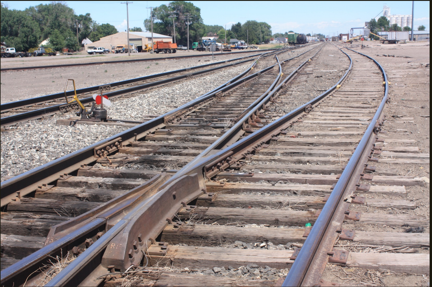
Now we're back at the M&SW (1905), just east of the junction for the OSL Goose Creek Branch (c1912) and looking east at the same location as the first photo. From left to right the tracks are a half-mile-long industrial spur, the M&SW (1905) mainline, a crossover track from sidings to the mainline, and two sidings. The two sidings converge to one track in the immediate foreground and that one track is the single siding that continues west (behind the viewer) as the OSL Goose Creek Branch (c1912). Note the silos in the right distance (which are not the "Union Seed" silos, which are behind the viewer).
