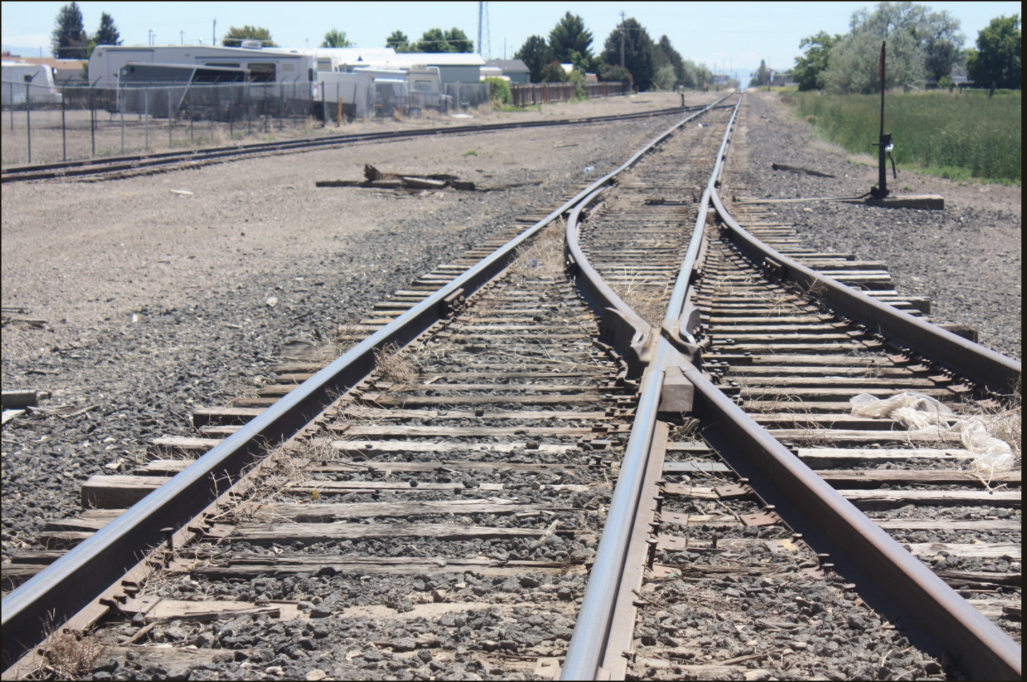
Closer look at the switch and trackage to the right that may have been the west branch of a wye for the OSL Goose Creek Branch (c1912). The Goose Creek Branch (c1912) originally extended 25 miles south of this location to Oakley but, probably around 1980, was cut back 13 miles. The line now ends 12 miles from here, where there are two spurs for (probably) active customers of the Eastern Idaho Railroad -- one spur for Sawtooth Stone and the other for Goose Creek Grain.
